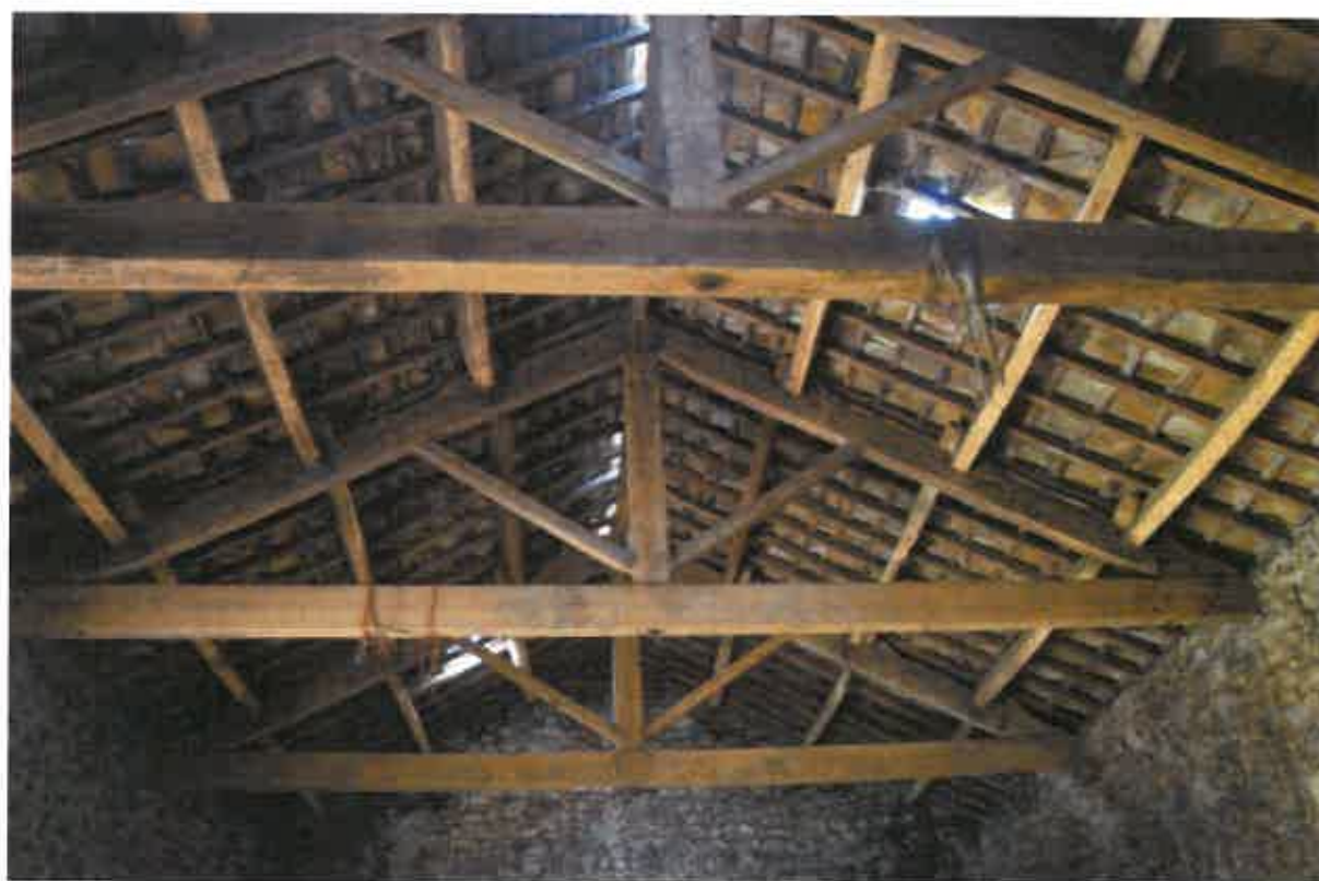
Photo 49: View of king post trusses and timber roof structure to Barn no.1.
