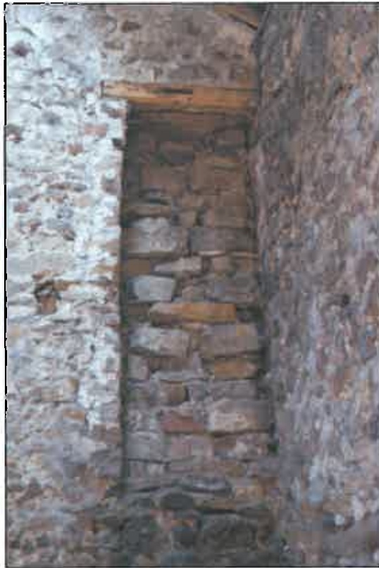
Photo 28 (left): View of blocked up door opening to the east wall at first floor level within barn 02.
