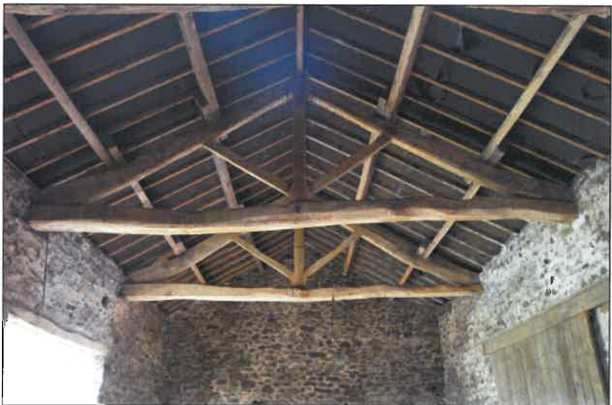
Photo 27: View of timber king post roof trusses and roof structure within barn no.2.
