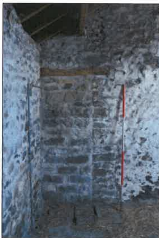
Photo 23: View of blocked up door opening to the first floor area above the stables to barn no.2.
