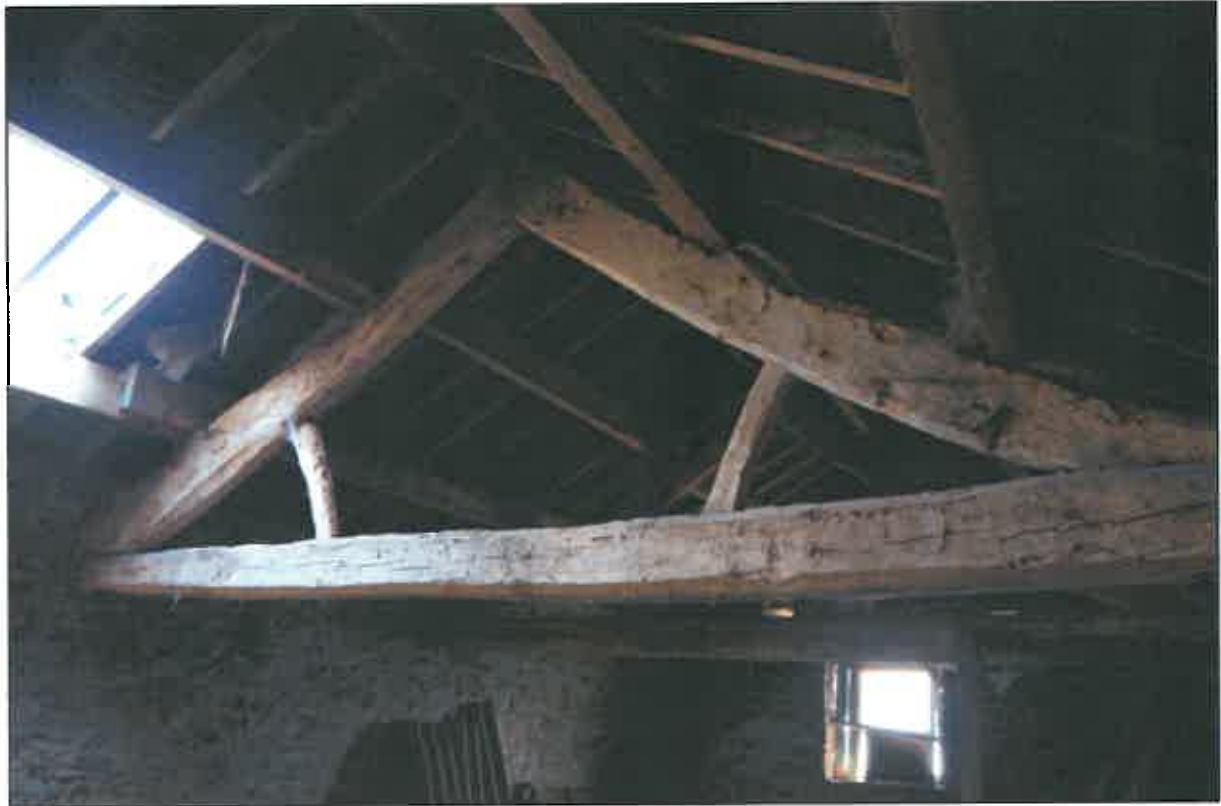
Photo 24: View of timber roof trusses within the first floor area above the stables to barn no.2.
