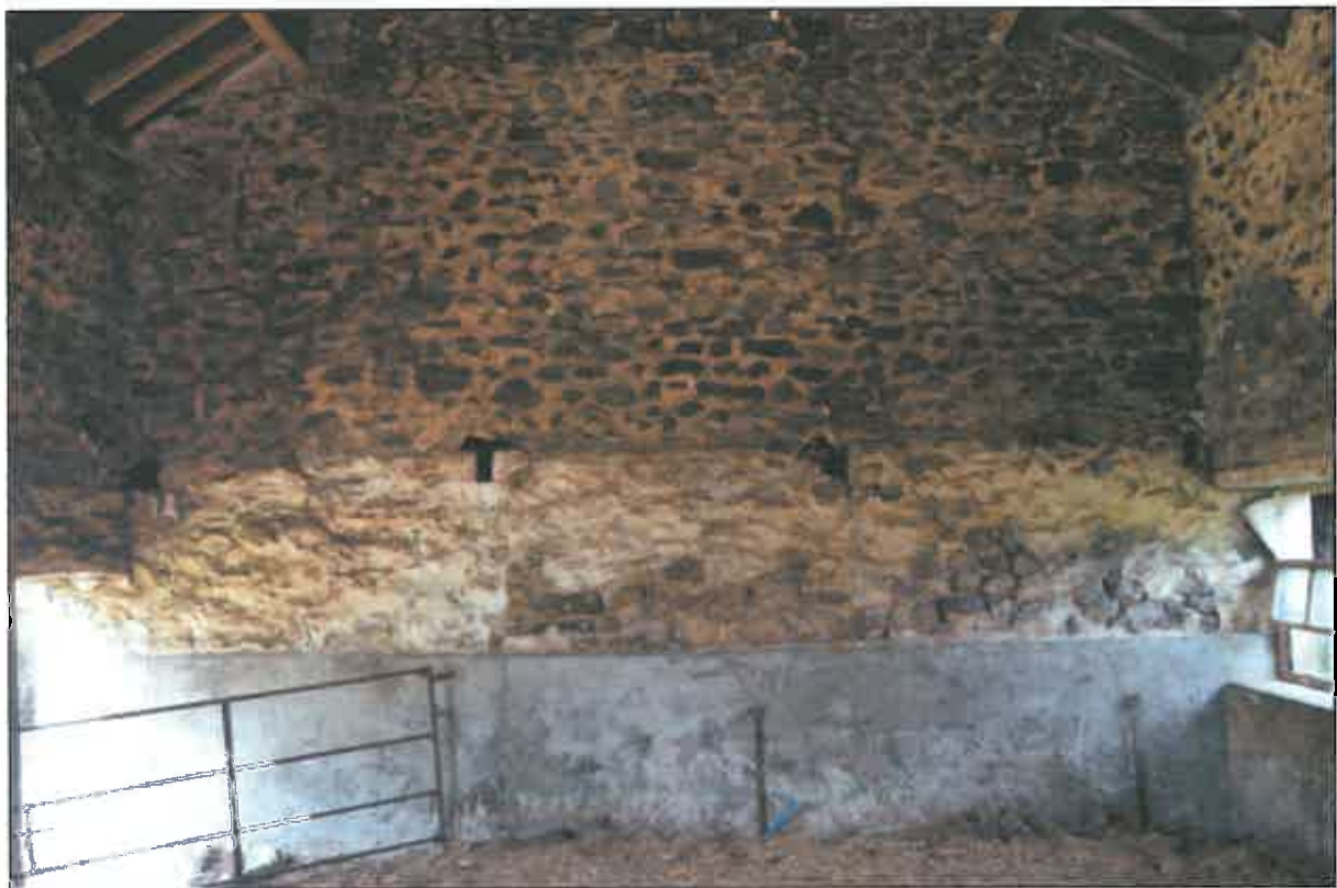
Photo 29: View of west wall within barn no.2. showing joists holes from former loft.
