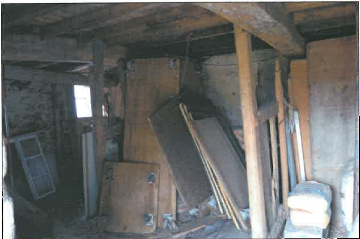
Photo 15: View of timber boskins within stable 01.
