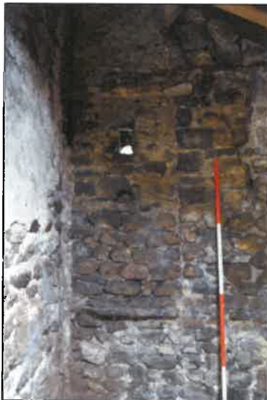
Photo 36: View of blocked up opening to the west wall of the livestock pen.
