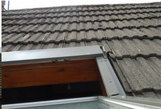
Rear roof pitch.
