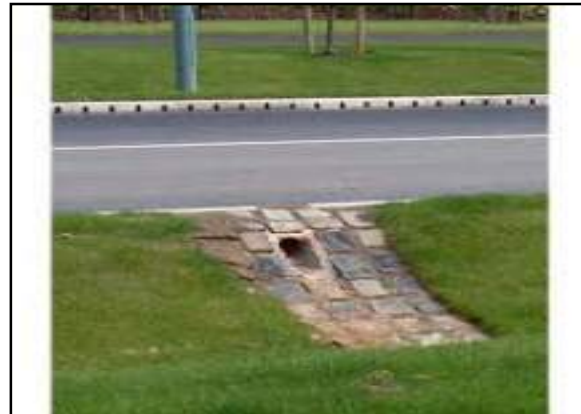
Photo showing gully into swale
