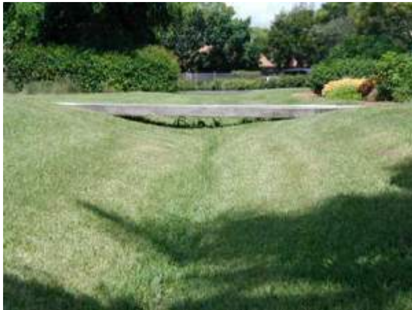
Photo showing typical swale located within open space areas with footbridge.
