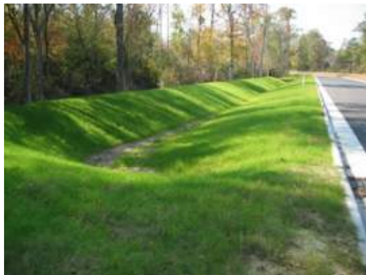
Photo showing typical swale located adjacent to highway
