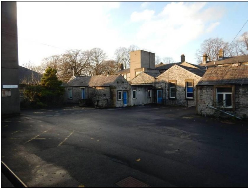
Photograph 12: Single-storey original outbuildings, including porter's lodge and stores at rear of former Workhouse.
