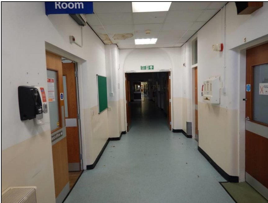
Photograph 3: Central corridor in former Workhouse showing minimal internal features.
