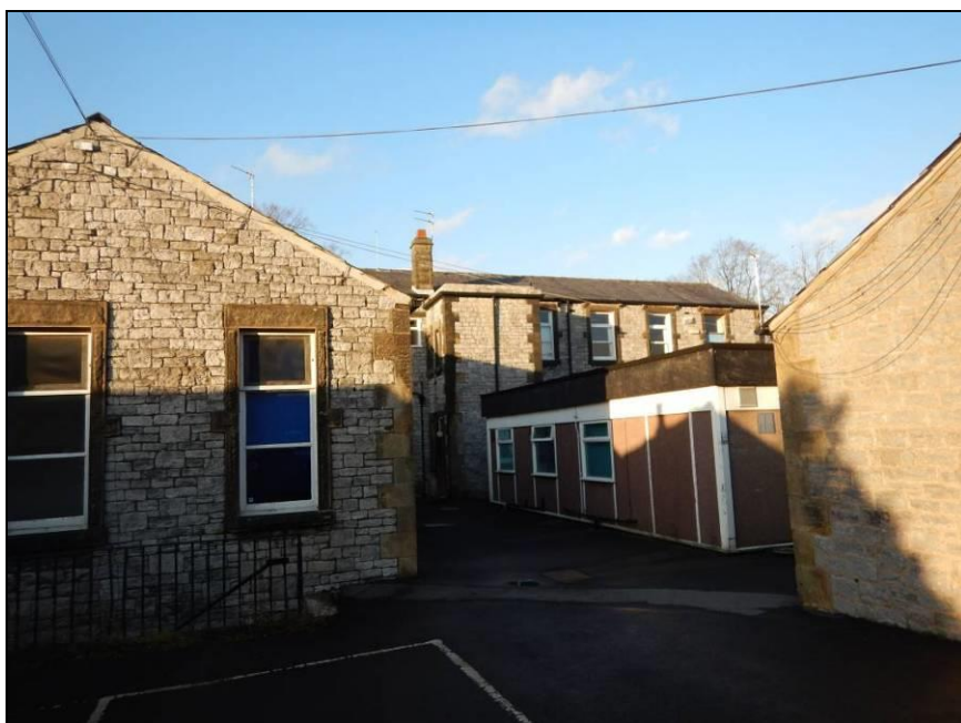
Photograph 2: Rear elevation of former Workhouse with single-storey outshot (kitchens) on the left and smaller two-storey outshot and modern prefabricated building to the right.
