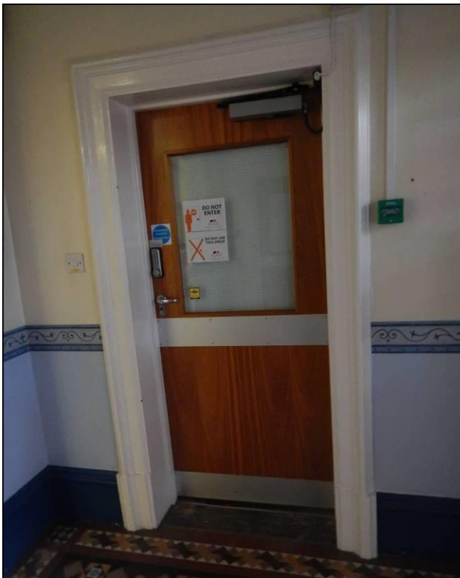
Photograph 6: Original door architrave.
