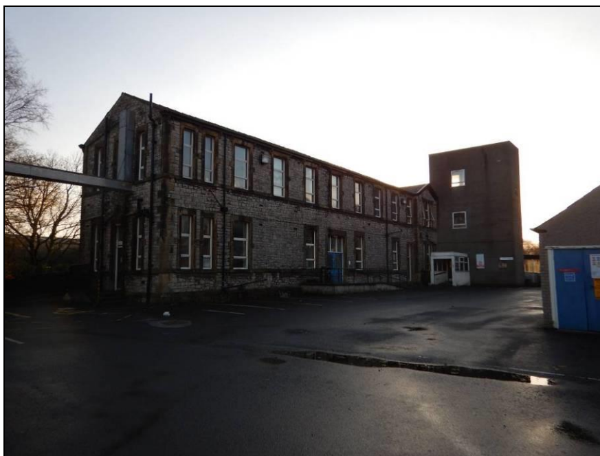
Photograph 7: Front elevation of the former Infirmary. Note the substantial, modern lift shaft and porch on the right of the photograph immediately behind the central gable. The lower windows of the central gable are obscured by the porch.
