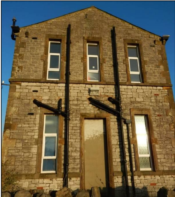
Photograph 8: Gable end return on former Infirmary demonstrating blocked door opening and tripartite windows.
