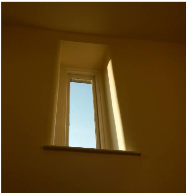
Photograph 11: Curved openings to window.
