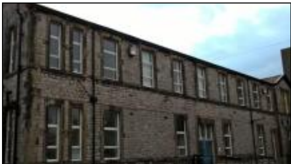
Photograph 7. Second hospital wing
