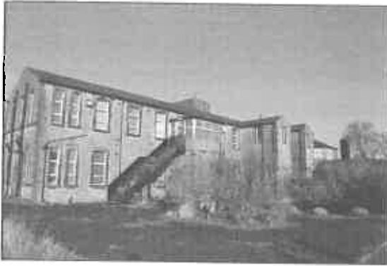
Figure 2.1: Photos of the Application Site
