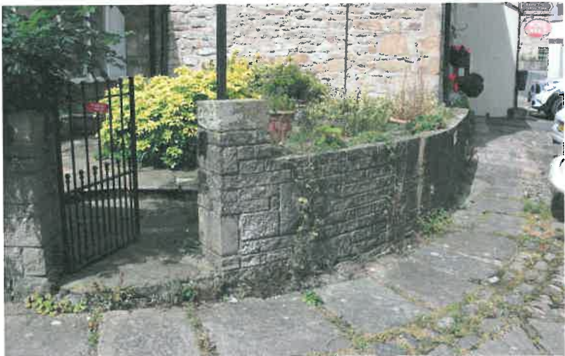
Detail of the garden wall, which is constructed with a reconstituted cut stone. The wall is to be partially removed to provide vehicle access on to the hardstanding and the remainder of the wall is to be replaced with a reclaimed random coursed sandstone, that matches the existing historic stone work.
