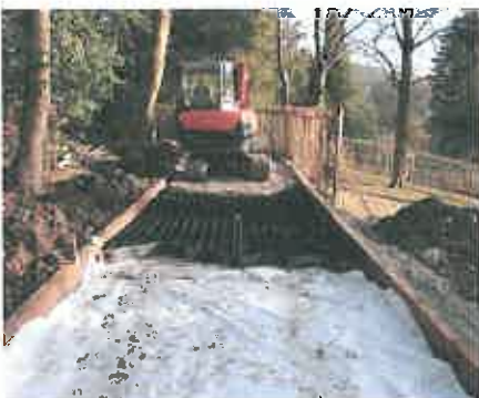
Fallbarrow Park, Windermere: CellWeb TRP® Installation
