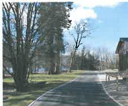
Fallbarrow Park, Windermere: Completed CellWeb TRP® Installation
