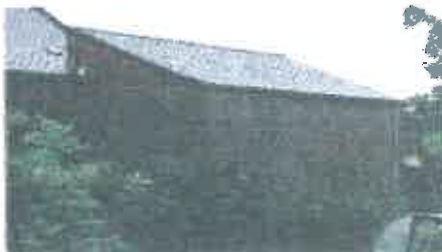
Figure 3. Wall and roof of building (south)
