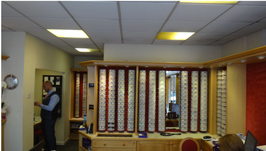
Ground floor plasterboard partition wall to be removed
