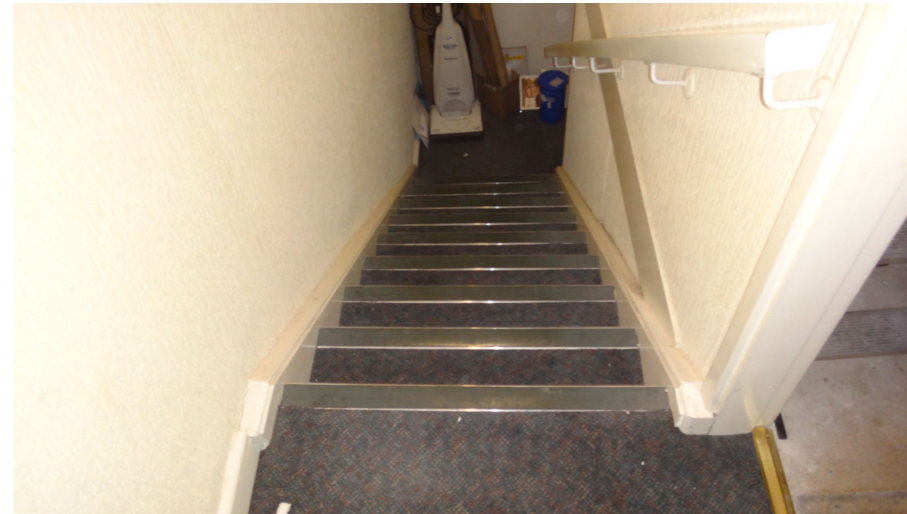
Top of stair flight to be retained in place
