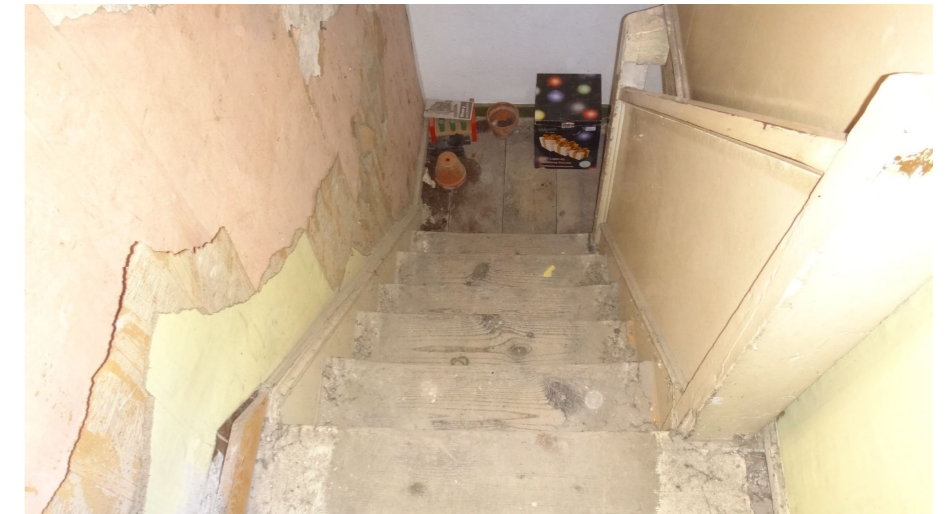
Top flight of stair from first to second floors
