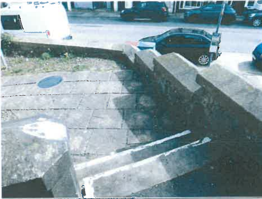
PHOTOGRAPH No. 5: MAXIMUM HEIGHT OF RETAINED GROUND LEVEL BEHIND WALL AT SOUTH END ADJACENT PARADISE LANE/YORK STREET JUNCTION.
