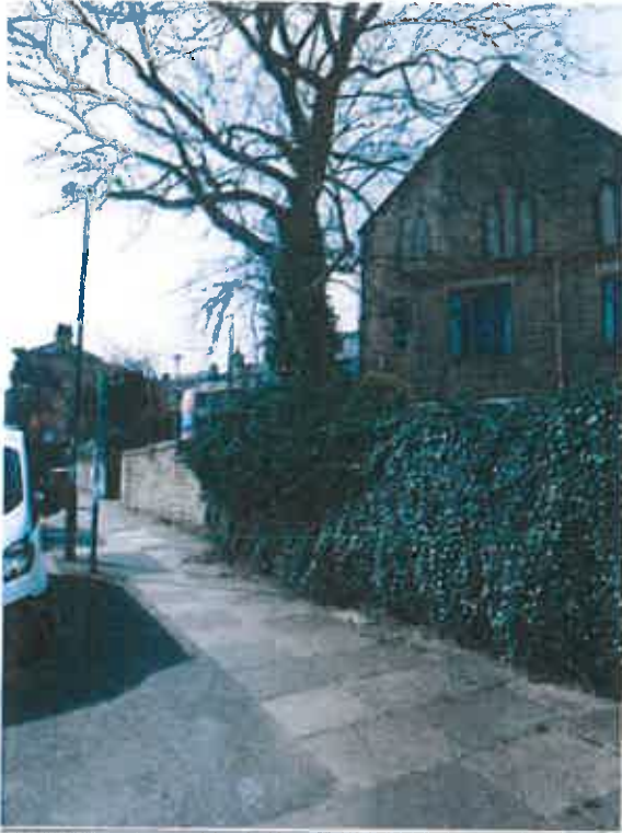
PHOTOGRAPH No. 3: VIEW ON EXISTING RETAINING WALL LOOKING SOUTH ALONG YORK STREET FROM GABLE OF ADJOINING PROPERTY NO.11 YORK STREET.
