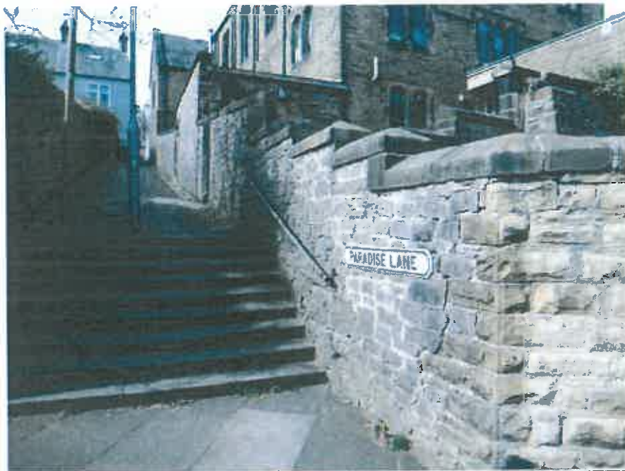
PHOTOGRAPH No. 2: VIEW LOOKING WEST ALONG FACE OF EXISTING STEPPED RETAINING WALL ON PARADISE LANE.
