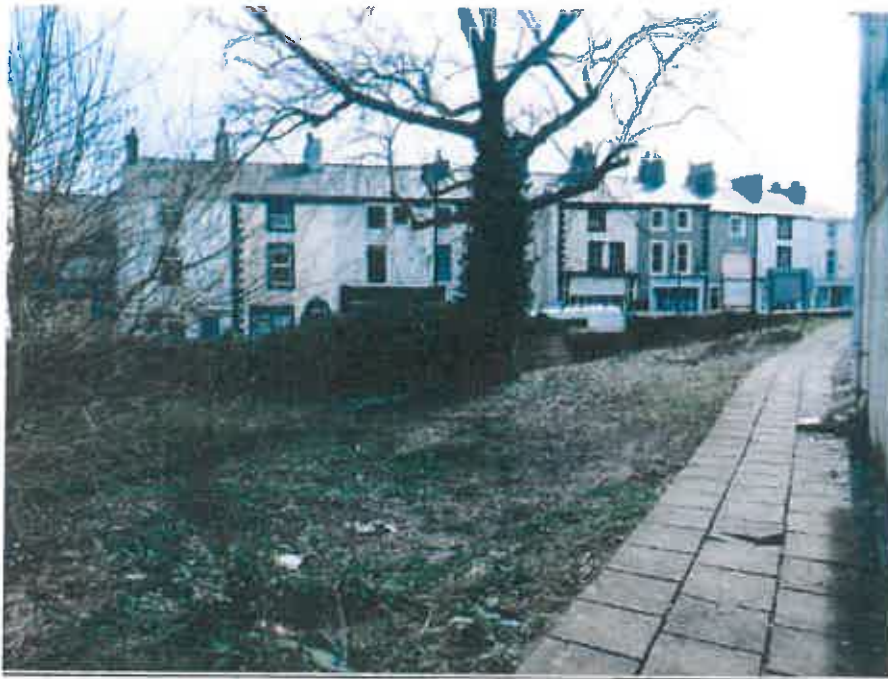
PHOTOGRAPH No. 7: VIEW ON REAR OF EXISTING RETAINING WALL TO YORK STREET.
