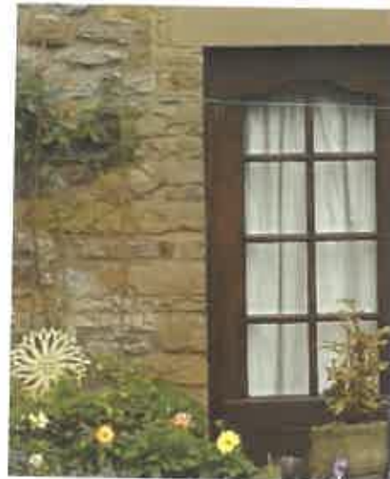
STONework DETAILING TO DOORWAYS STONE LINTOL DRESSED SQUARE STONE REVEAL ALL NEW SINGLE DOORS TO BE HARDWOOD. THE LARGE BIFOLD DOORS TO BE IN ALUMINIUM COLOUR TO MATCH HARDWOOD FRAMES
