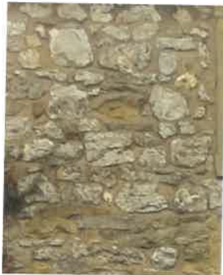
PROPOSED RANDOM STONE WORK WALLING BUILT FROM RECYCLED LOCAL GRIT SANDSTONE NOTE NEW CHIMNEY TO BE BUILT UP FROM MATERIAL OF DEMOLISHED REDUNDANT CHIMNEY TO INCLUDE THE ORNATE POT
