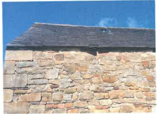
PL4 (Left) and PL5 (Right) showing cracked, chipped and dislodged slates along with vegetation growth.
