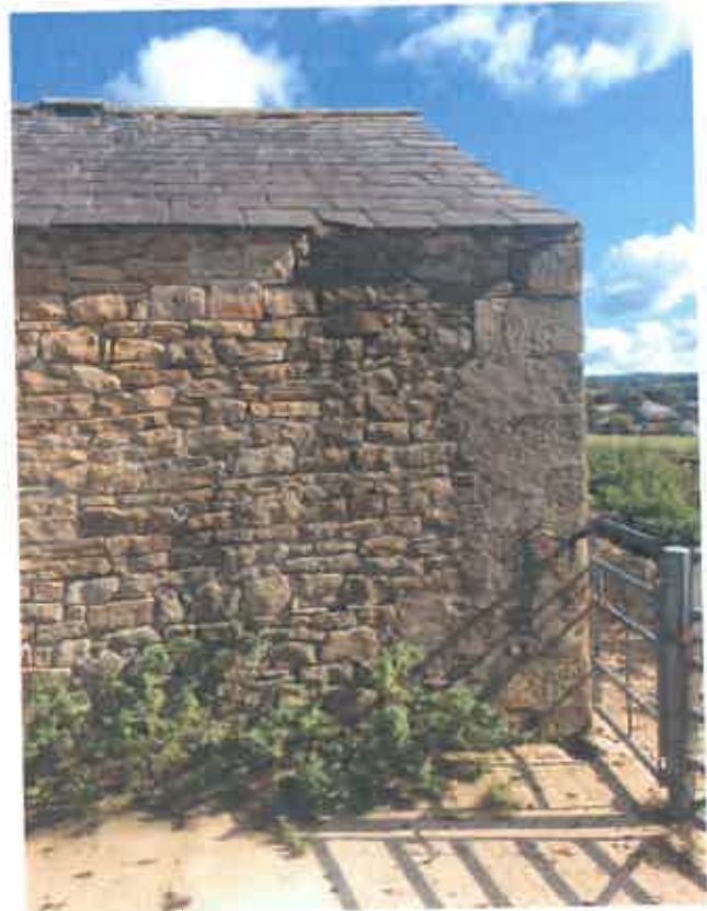
PL35 (Left) shows mortar repairs to stone joints and significant plant / weed growth to base of wall. PL36 (Right) showing mortar patch repairs, mortar degradation and plant / weed growth.
