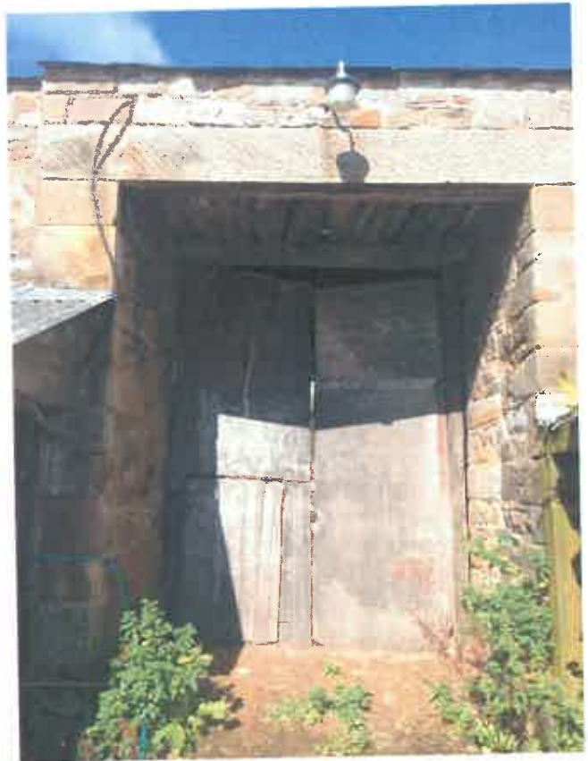
PL46 (Left) and PL47 (Right) showing dilapidated and damaged external doors.
