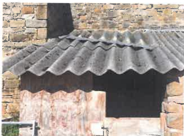
PL8 (Left) and PL9 (Right) showing the condition of the asbestos roof covering and the section of dislodged lead flashing (this particular area is to be demolished).
