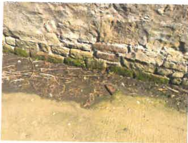
PL33 (Left) showing mortar degradation to base of wall. PL34 (Right) showing hole damage and hairline cracking to west elevation.
