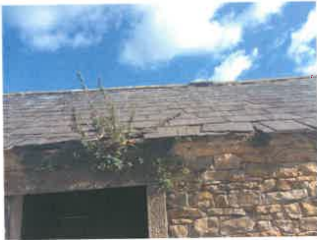
PL4 (Left) and PL5 (Right) showing cracked, chipped and dislodged slates along with vegetation growth.
