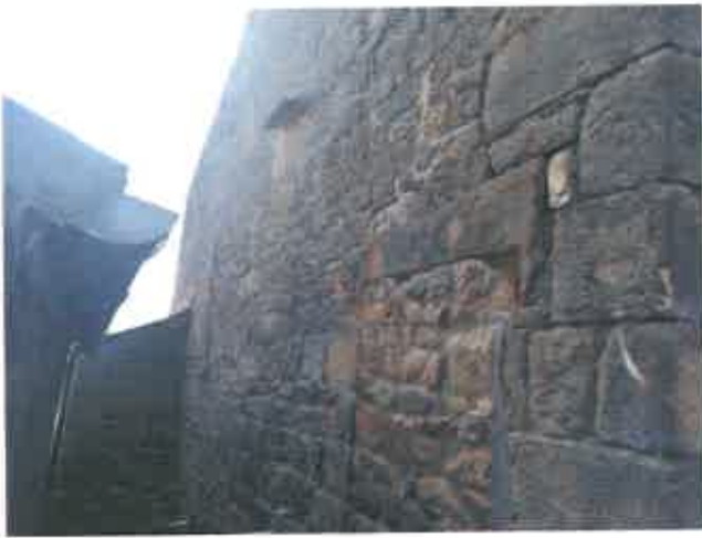
PL25 (Left) showing condition of the east elevation gable wall with degraded mortar and patch repairs. PL26 (Right) showing cracking to east elevation gable wall.
