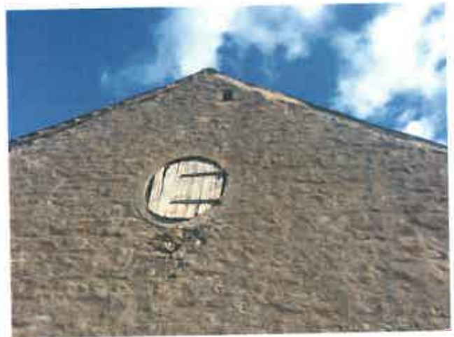
PL48 (left) showing dilapidated window frame with wire mesh infill. PL49 (Right) showing poor condition of pitching hole door and rusting hinges.
