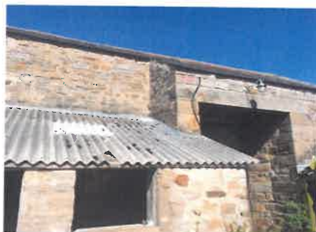
PL8 (Left) and PL9 (Right) showing the condition of the asbestos roof covering and the section of dislodged lead flashing (this particular area is to be demolished).
