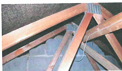
Figure 3: main roof void
