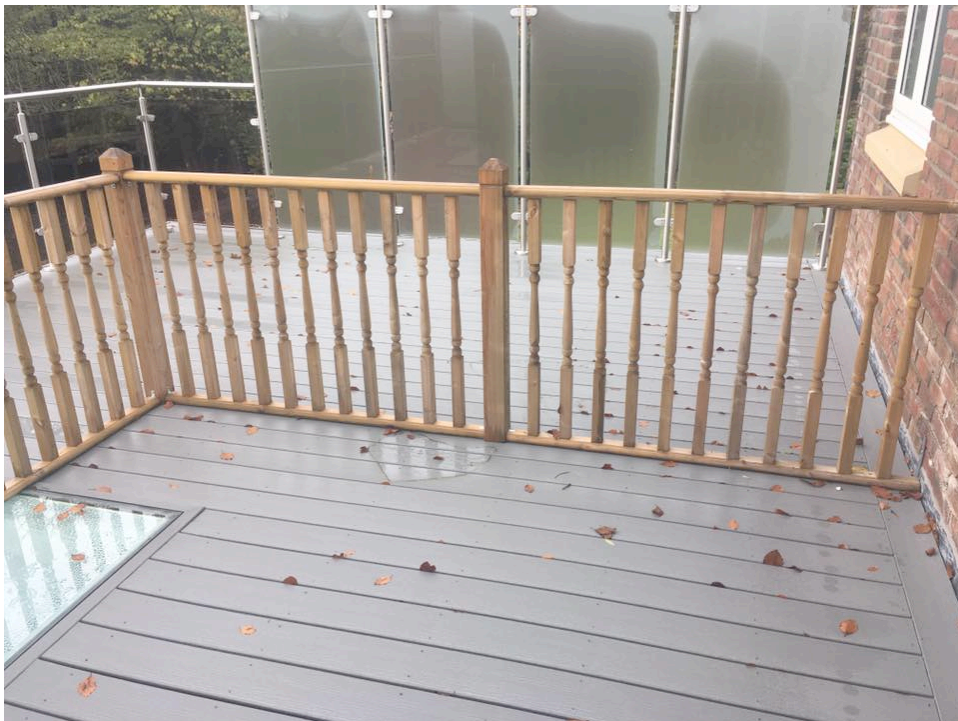
Photo 2: 'Inner' timber balcony feature and 'outer' glazed balcony feature (As implemented, south-west facing view)
