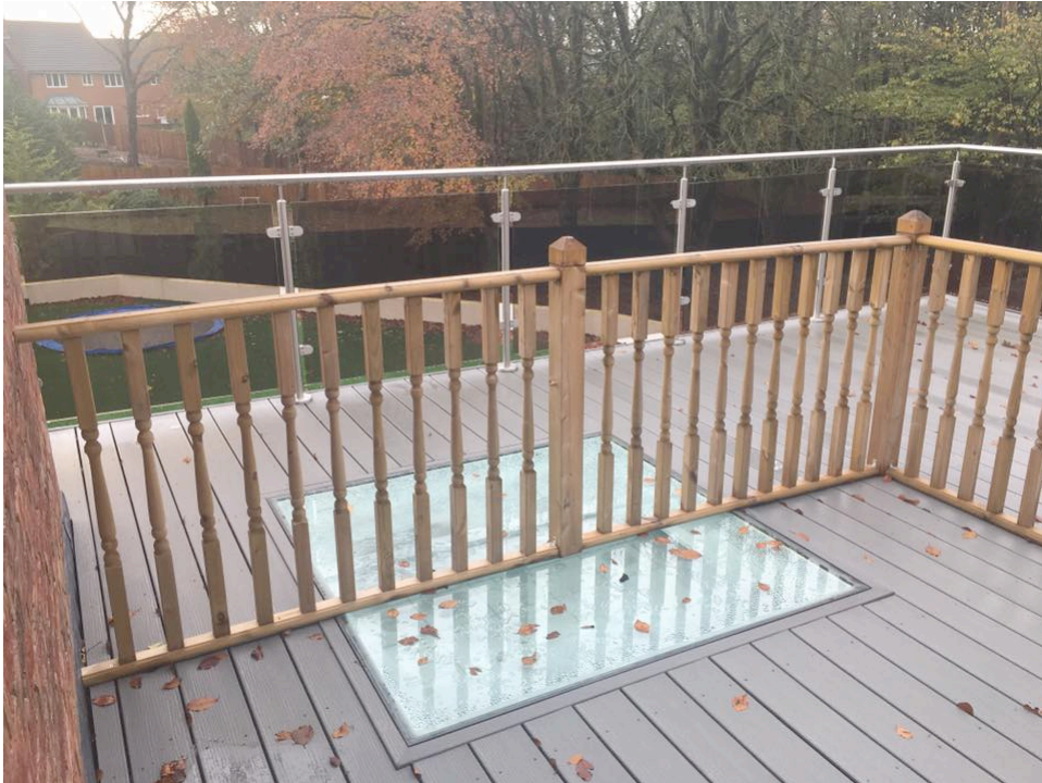
Photo 1: 'Inner' timber balcony feature and 'outer' glazed balcony feature (As implemented, south facing view)
