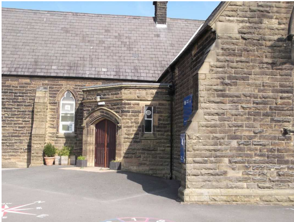
Figure 5(South East Elevation) facing on to the river
