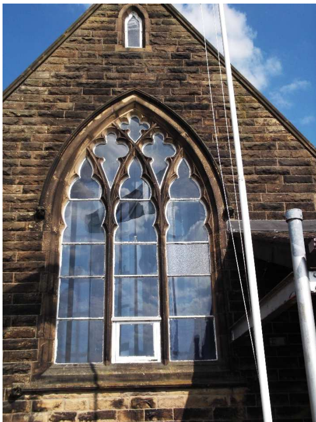
Figure 6 (South East Elevation) facing on to the river
