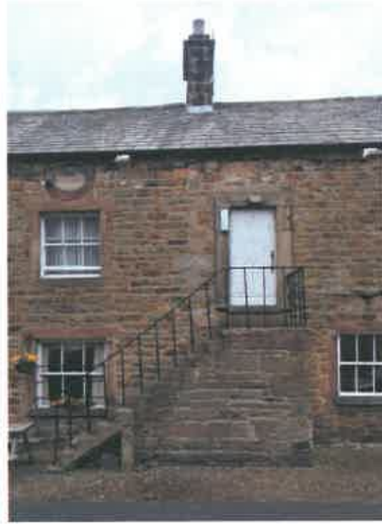
PL14 (left) showing the abutment between the 17 th century building and the 18 th century addition. This is identifiable through the difference in material finishes and the slight setting back of the 18 th century addition. The quoin stones to the 17 th century building indicate its original extent. PL15 (right) showing a clear division between the two different sections of the 17 th century buildings and can be identified through the slightly different external finishes and the stonework which has been used to tie the two walls together (to the left of the first floor door).
