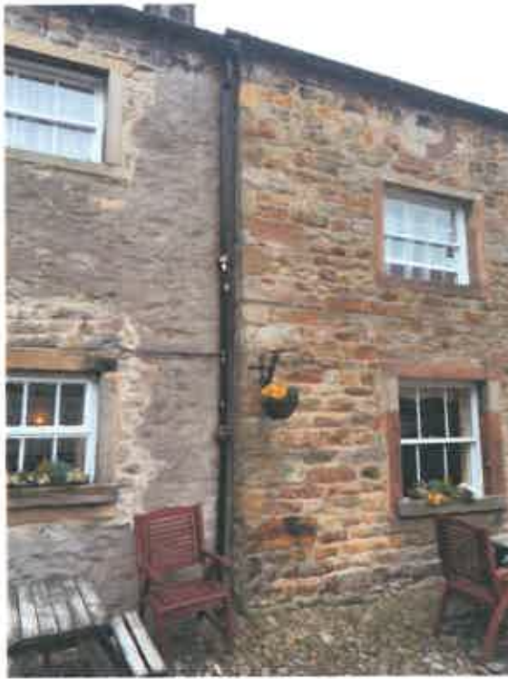
PL14 (left) showing the abutment between the 17 th century building and the 18 th century addition. This is identifiable through the difference in material finishes and the slight setting back of the 18 th century addition. The quoin stones to the 17 th century building indicate its original extent. PL15 (right) showing a clear division between the two different sections of the 17 th century buildings and can be identified through the slightly different external finishes and the stonework which has been used to tie the two walls together (to the left of the first floor door).
