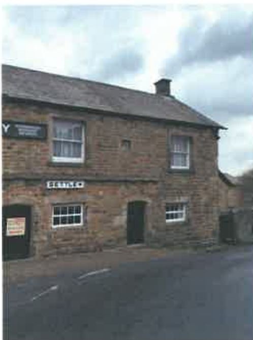
PL16 (left) showing clear dichotomy in the stone work between the ground floor and first floor of the 17 th century building. This would suggest that the first floor has been rebuilt. PL17 (right) showing quoin stones that are partially obscured by the stone steps. This would suggest that this was one the original extent of the building i.e. the gable, or a doorway was one located here prior to the construction of the steps.
