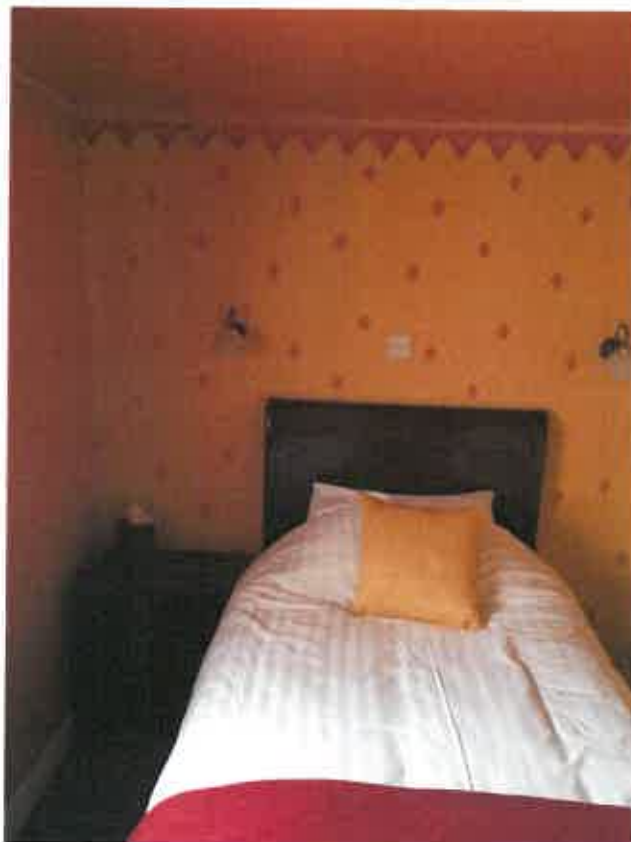
PL08 showing the west gable wall within the front guest room.
