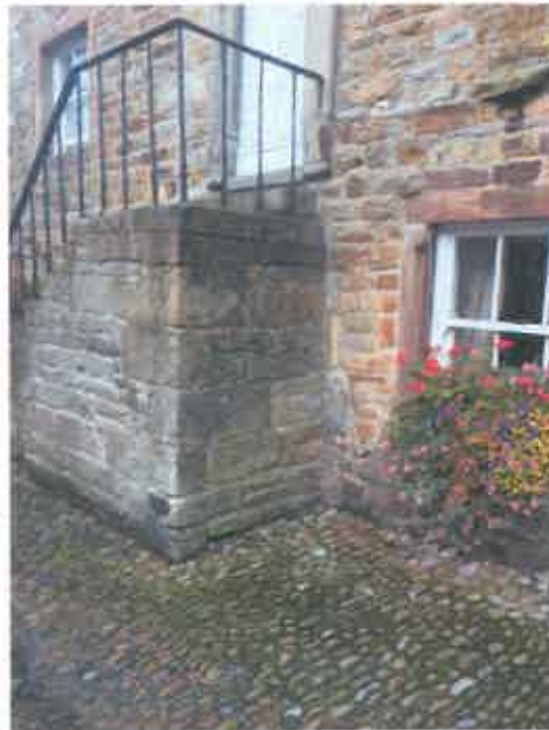
PL16 (left) showing clear dichotomy in the stone work between the ground floor and first floor of the 17 th century building. This would suggest that the first floor has been rebuilt. PL17 (right) showing quoin stones that are partially obscured by the stone steps. This would suggest that this was one the original extent of the building i.e. the gable, or a doorway was one located here prior to the construction of the steps.
