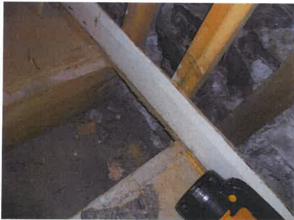
Front Bedroom – floor opening
