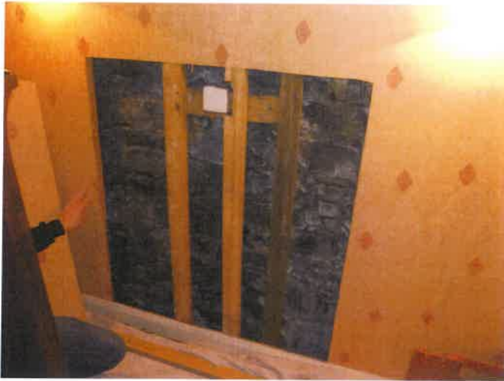
Front Bedroom-opening showing inner stonework
