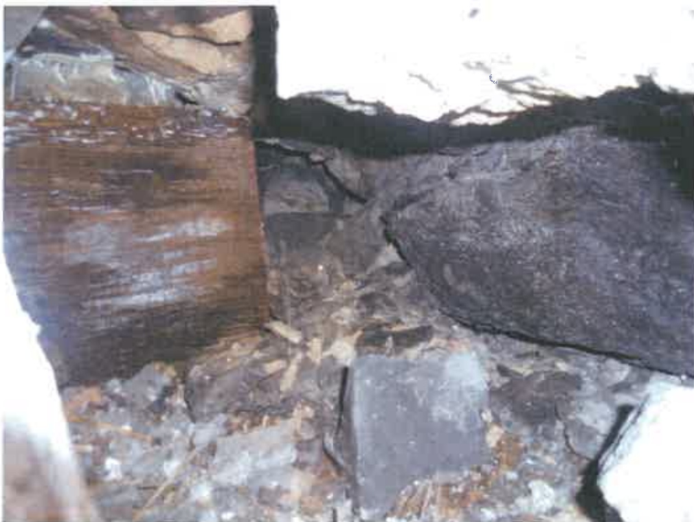
Landing - joist and void in wall
