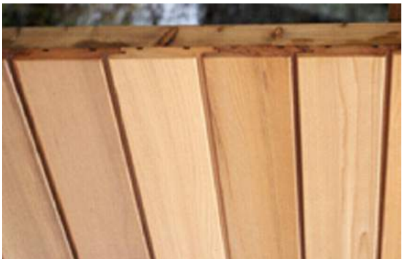
Cedar Cladding: Western Red Cedar Cladding above fixed horizontally to vertical treated battens. Cedar Cladding to be RW115 Secret fix profile. Boards to be 20mm thick and 150mm wide fixed in alternating lengths with staggered joints. Supplied by Russwood or equivalent manufacturer.
