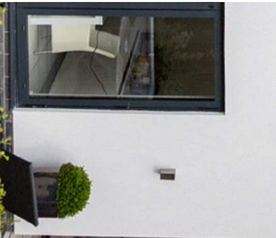
K-Rend Walls to be finished externally with K Rend Scraped Texture Finish 1 Coat (2passes) finish coat 10mm. Proposed colour 'Mink'.
