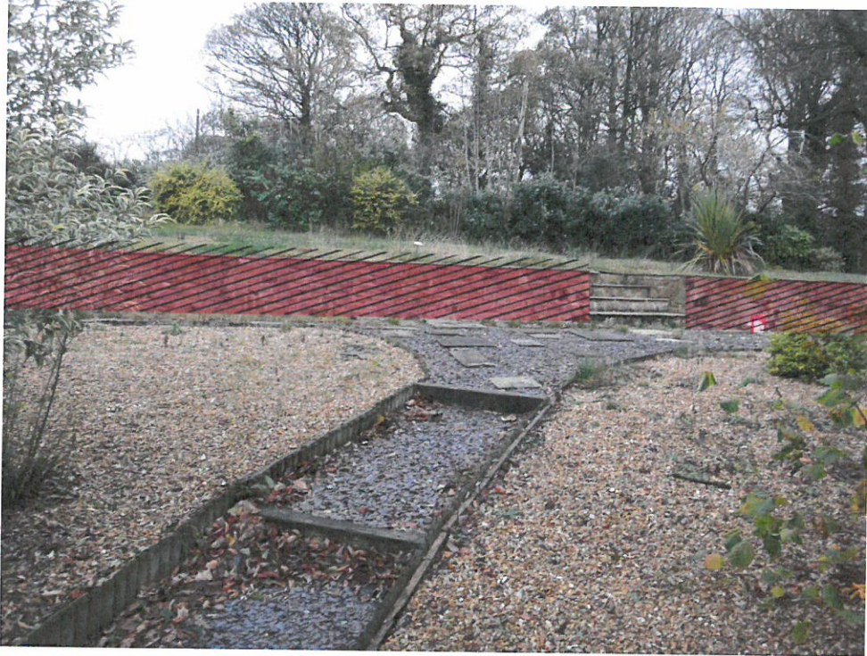
Garden Wall: Hatch area of stone to be reused.
