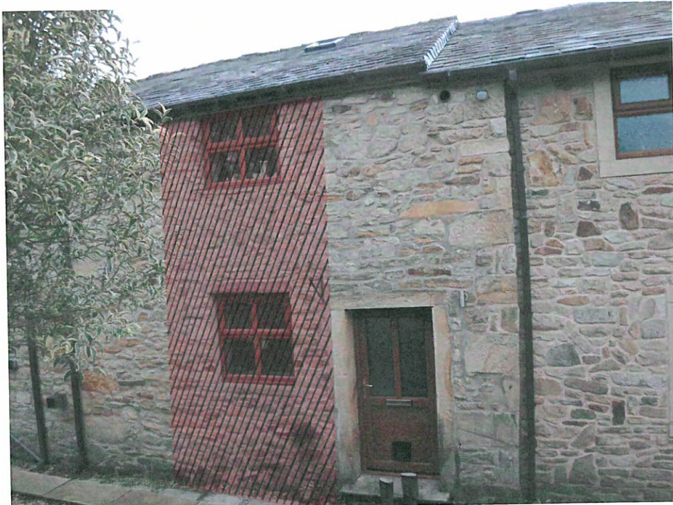
Rear Elevation: Hatch area of stone to be reused.
