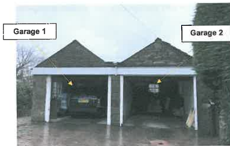
Photograph 1: External View of Front of Garages
