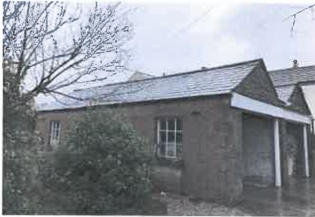
Photograph 2: External View of Garage 1
