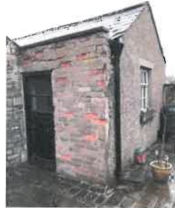
Photograph 3: External View of Garden Store
