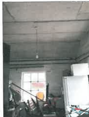
Photograph 6: Internal View of Garden Store
