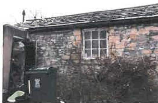
Photograph 4: External View of Garage 2 South Eastern Elevation showing stone tiles
