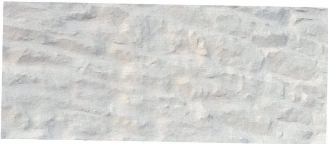
Existing painted stonework and natural slates.
