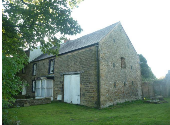
Photo 14: Occupied dwelling and adjoining barn; northern and eastern elevations
