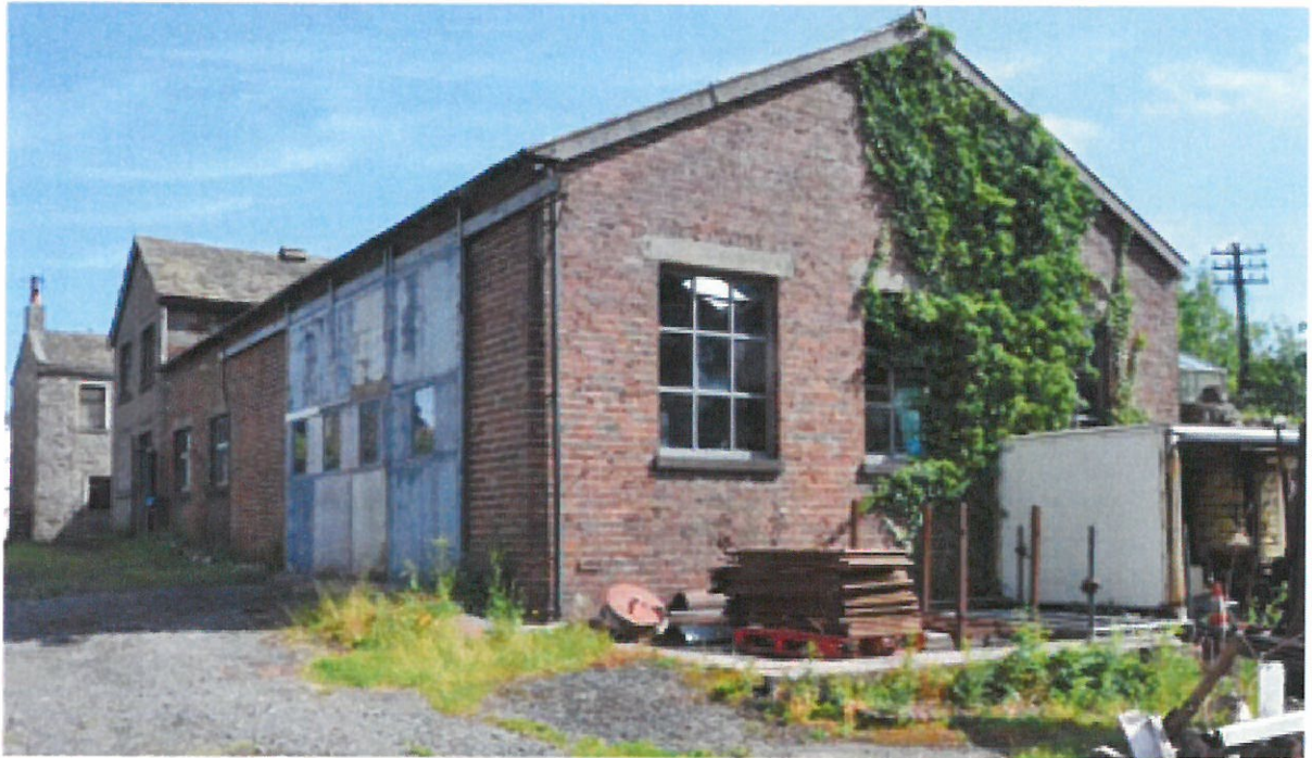
Existing building to be demolished during Phase 1 to make way for Plot 2 during Phase 2
