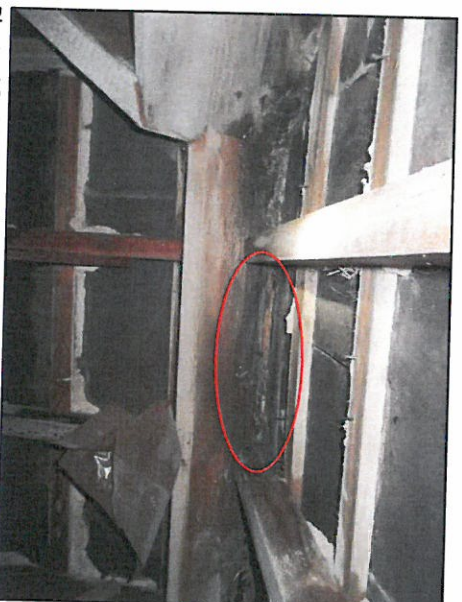
Photo 16: Central ridge correlating with missing mortar.
