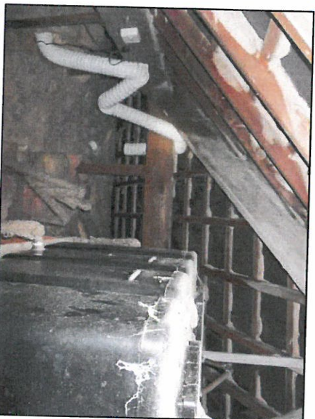
Photo 13: Loft space showing unlined roof structure.
