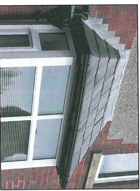
Photo 3: Bay window with half hipped slate roof.
