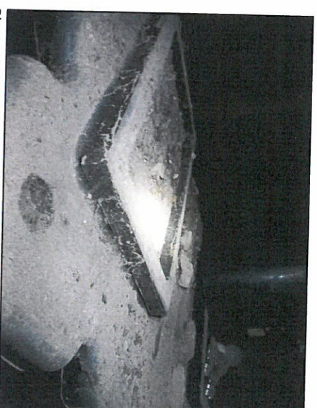
Photo 15: Daylight visible through roof slates.
