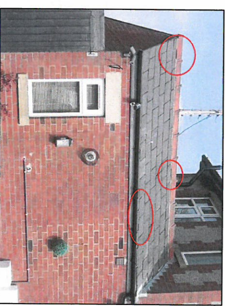
Photo 9: Missing mortar in ridge tiles and gaps in slates.
