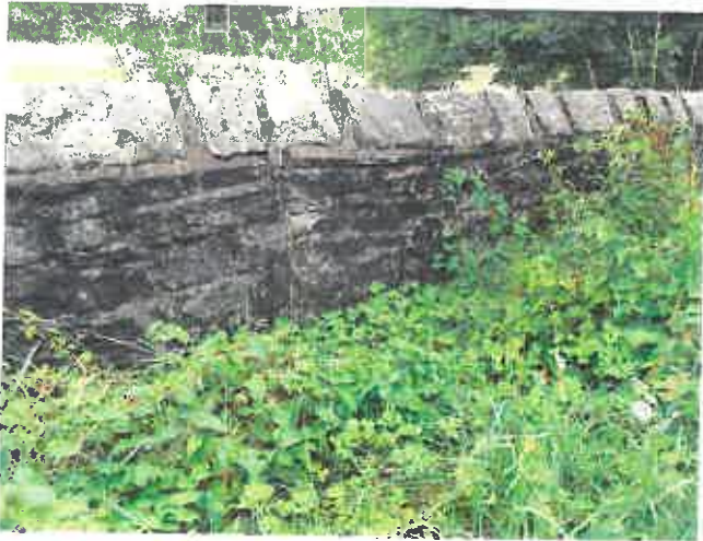
1. Stone boundary wall.
