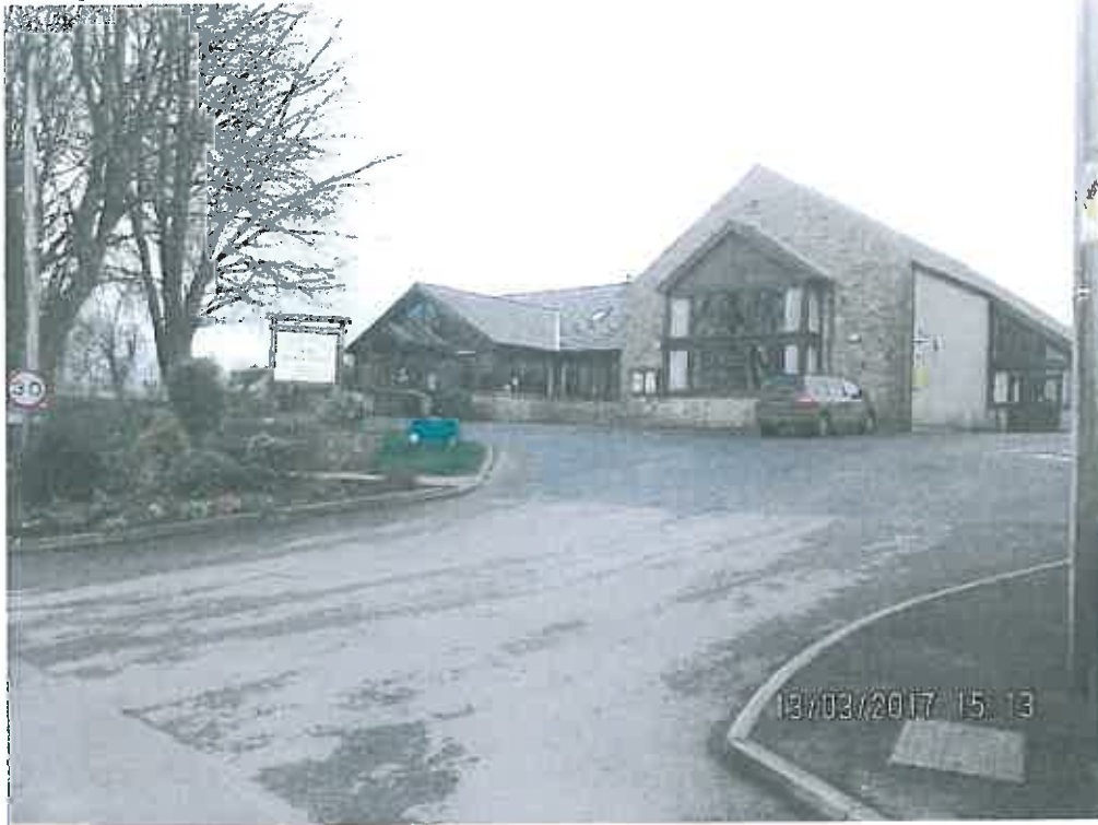
Memorial Village Hall - blue slate roof, random stonework, rendered panels, dark stained timber
