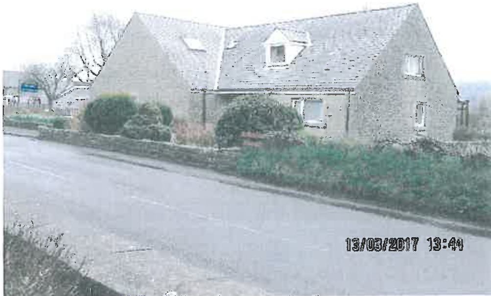
Farm shop/bungalow, artificial stone random blocks, heads, sills, linings, blue slate roof, no overhang
