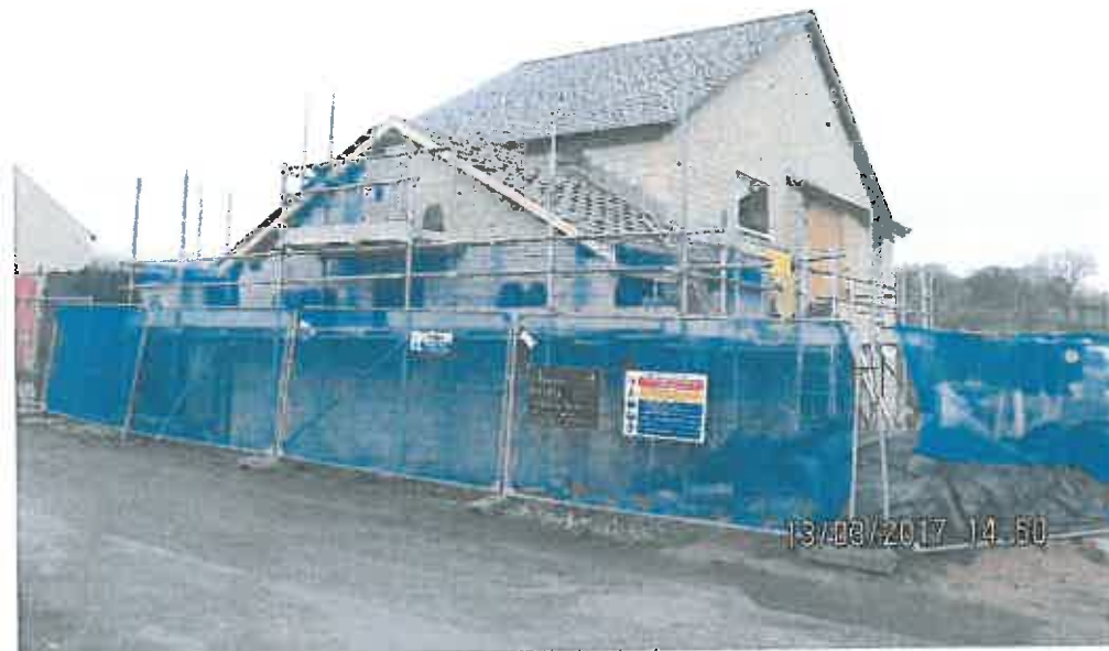
Detached house, Church Raikē, similar to semi detached development except using artificial slate and gable overhangs
