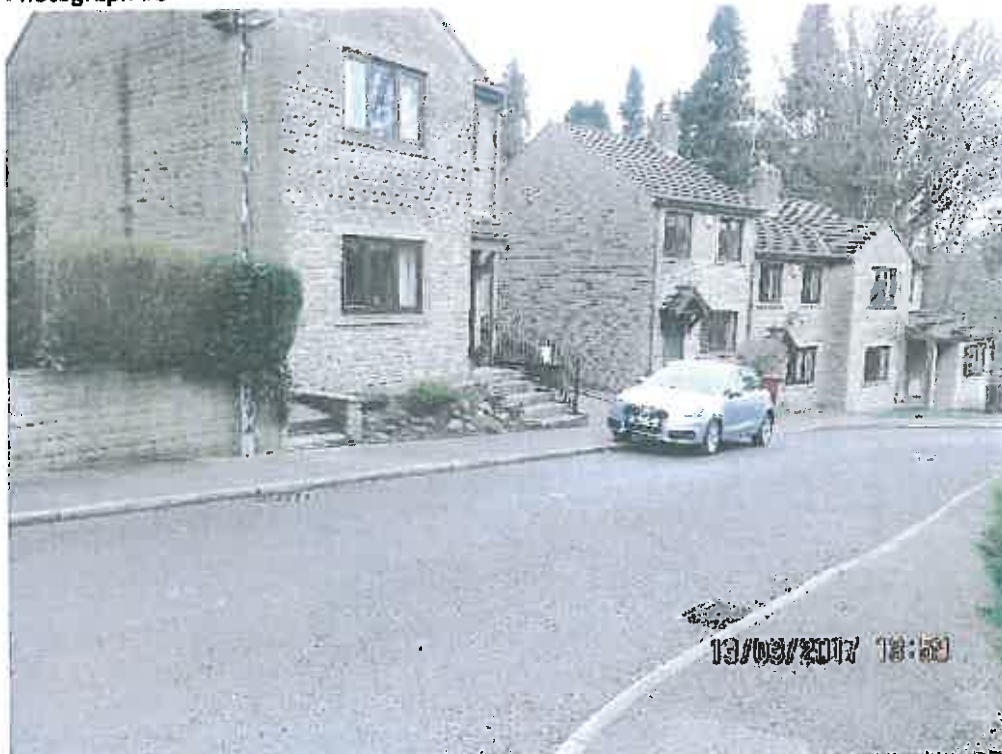
Brooklands Court, artificial stone walls and stack in Moordale, dark grey plain marley modern tiles, artificial stone heads and sills, dark stained windows set back 75mm
