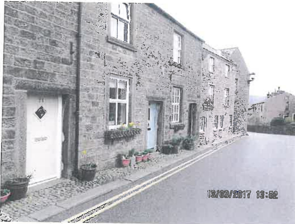
22-25 Windy Street – ribbed dressed door and window surrounds
