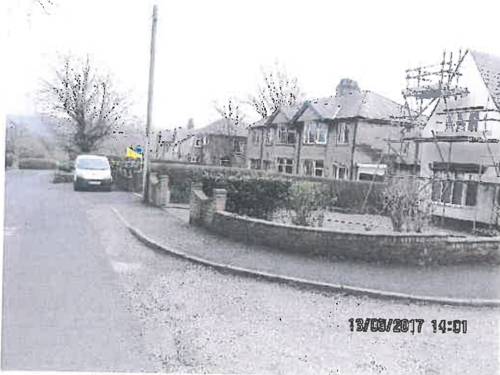
Longridge Road semi detached houses, a mixture of pebble dash, rough cast, stone walls, all stone heads and sills with blue slate
