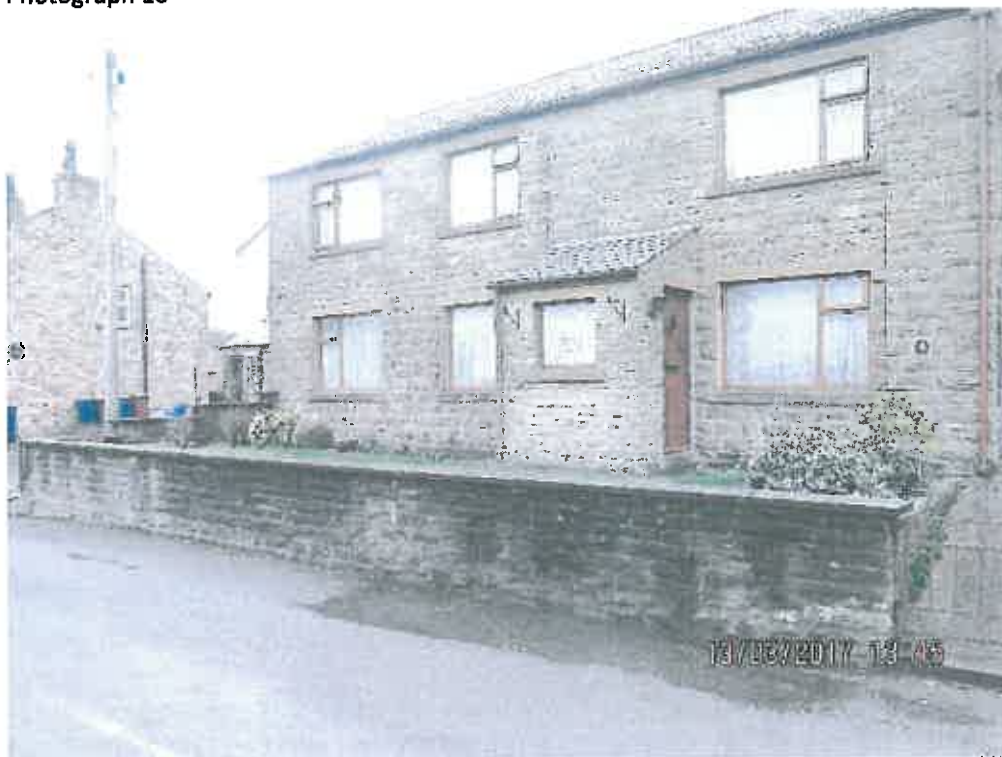
Individual house backing onto car park, natural stone but with artificial heads and sills, blue slate roof, no overhang
