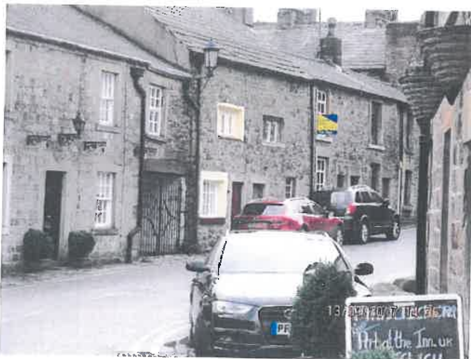
Deep double chamfered stone window set, stone slate roof, simple casement windows including Yorkshire sliding sash, 12-14 Talbot Street, circa 17 th century, Grade II
