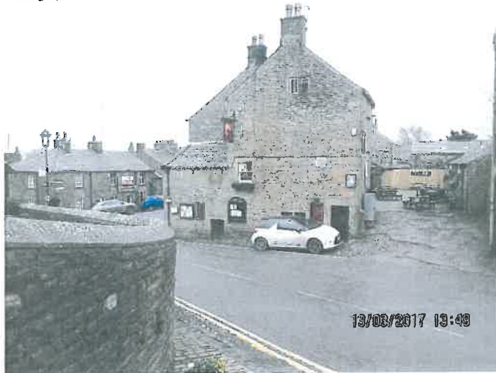
Gable wall to the Sun Inn, large quoin stones, diminishing but random course, mullioned stone heads, windows, Grade II
