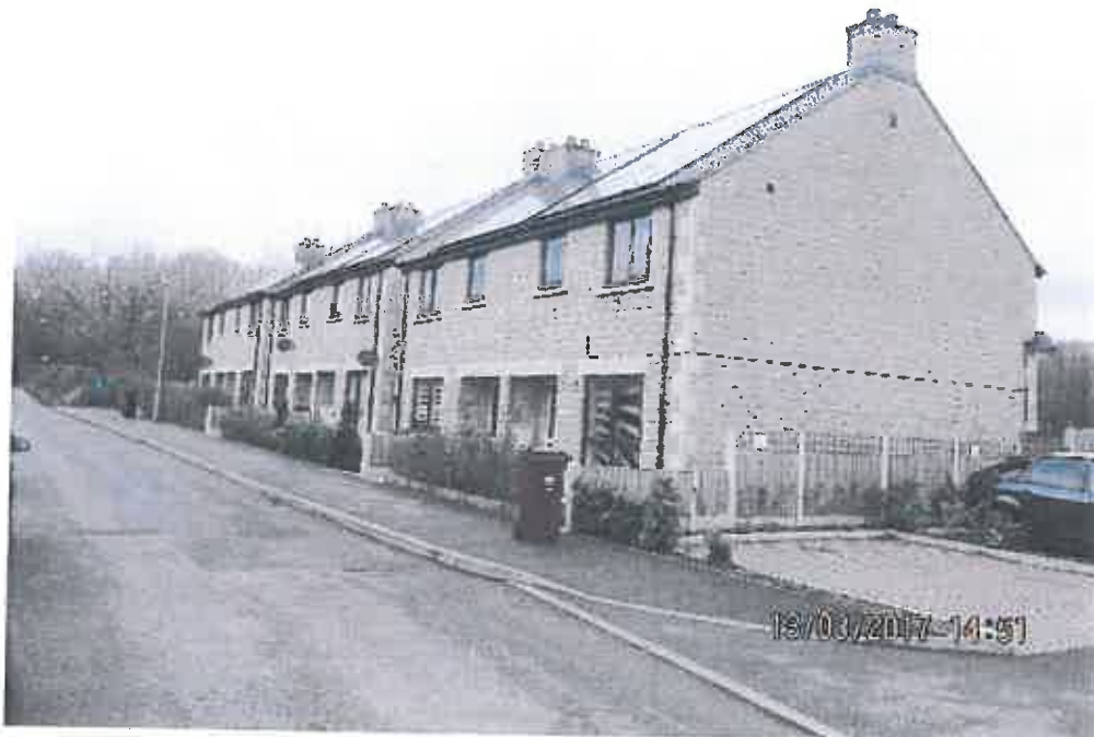
Semi detached houses at Church Raikes, slate roof, stone artificial stone walls, minimal overhang, rainwater goods and fascias dark stained
