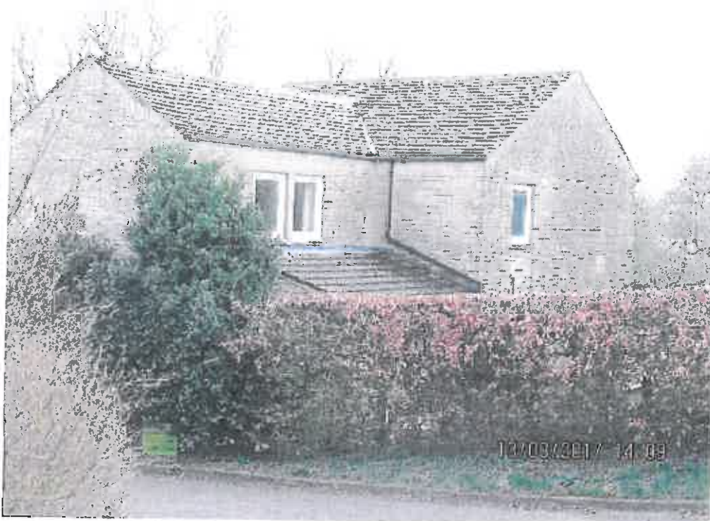
Brooklands, no stacks, hard row concrete tiles, part mullion window openings, similar full size window patterns
