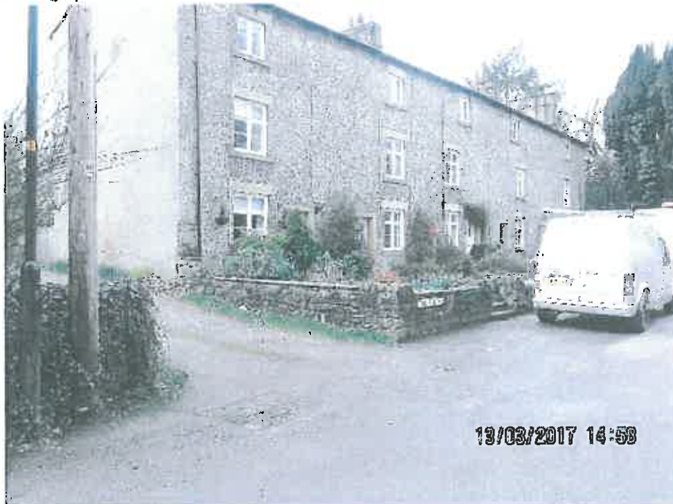
Three storey stone cottages. There is an exposed left hand side corner which revealed very random stone and this may be the reason why they were rendered. They have stone heads and sills and large stone stacks. 1-5 The Grove.
