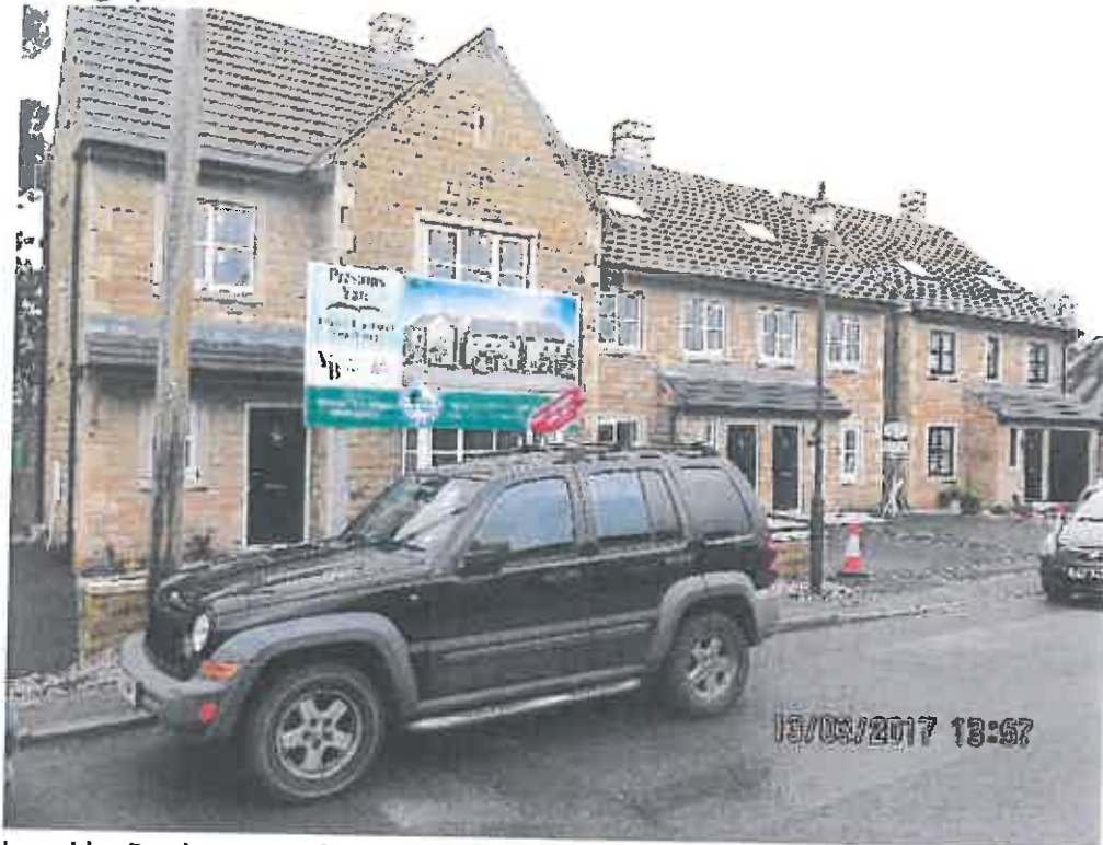
Longridge Road, steep roofs, plain tiles, natural stone walls, upvc windows set forward
