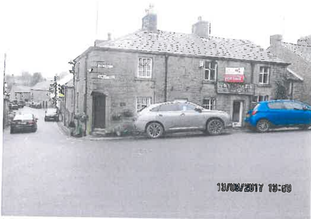
Corner of Windy Street/Talbot Street, dressed projected quoins over cantilevered door surround
