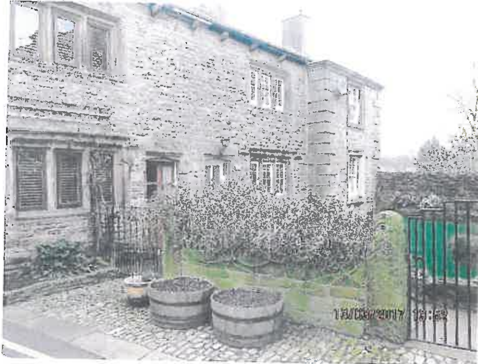
Hooded and chamfered mullion door and window sets, random stone coursing and stone slates, 17-19 Windy Street, circa 17 th century, Grade II
