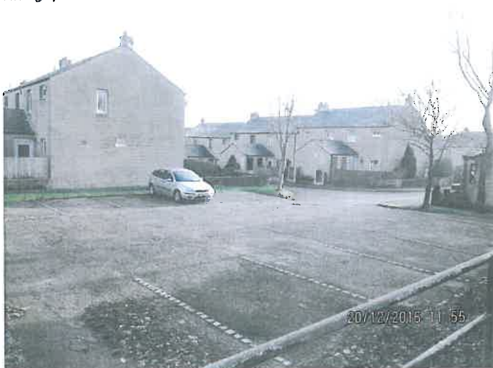
Typical street scene, concrete block walls, simple pattern windows, flush roof detail, small blockwork stacks
