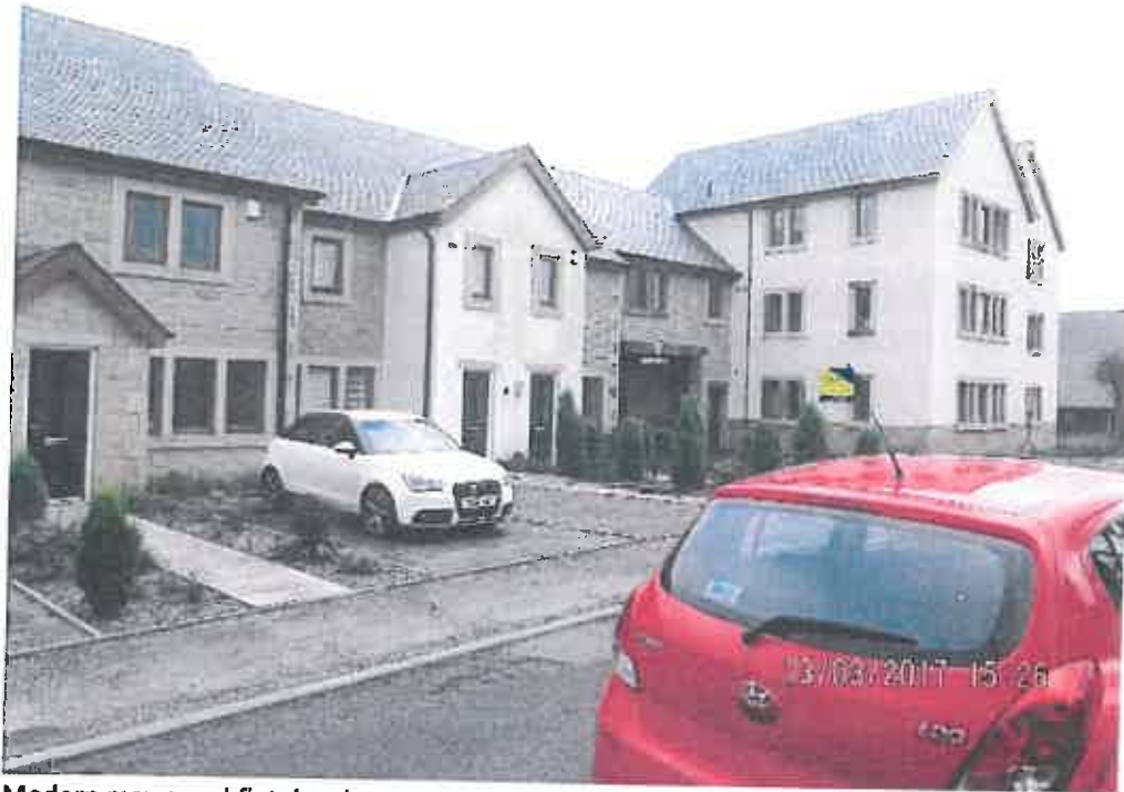
Modern mews and flat development, Kirklands, blue slate, dark stain fascia and windows, artificial heads, sills and linings, course stonework
