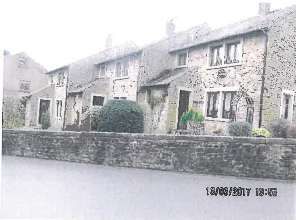
18-22 Windy Street, random stone, rough quoin stones, artificial stone heads, sills and linings, blue slate roof, dark stain window set back
