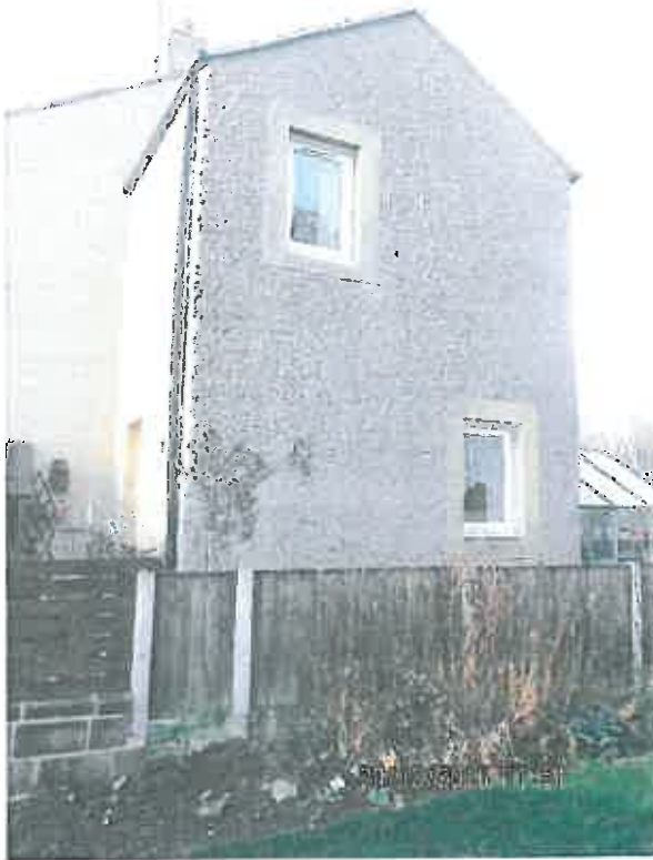
Outriggers to the social house, rough cast render, smooth rendered stone effect window surrounds and windows set back 100mm
