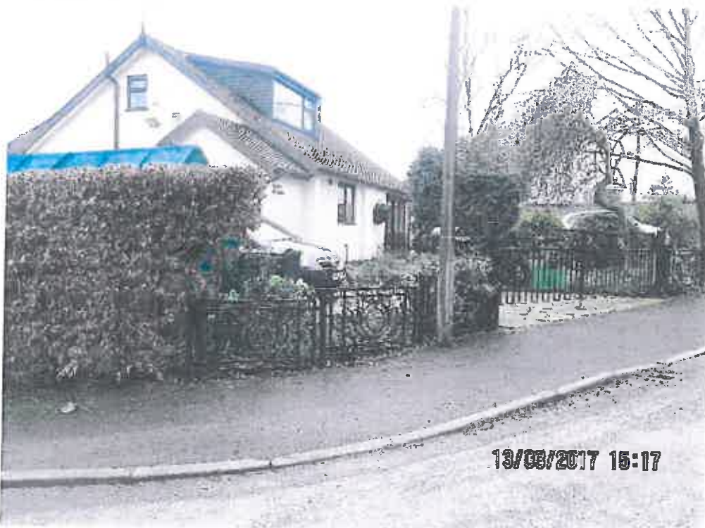
Bungalow at Broad Meadow, roof pitched at 40°, small plain concrete tiles, small roof overhang, off white render
