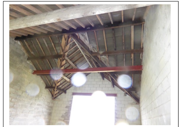
Fig 4. Central Core Roof Structure
