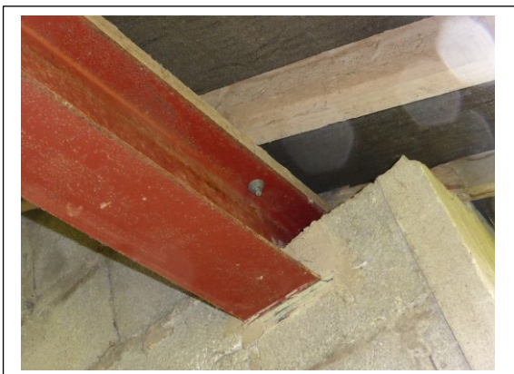
Fig 5. Central Core Eaves Beam/Bolted Wallplate Detail
