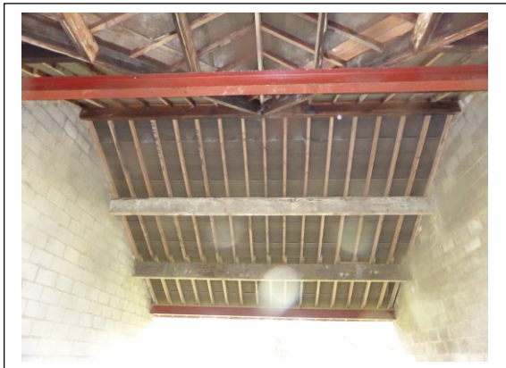
Fig 3. Central Core Roof Structure
