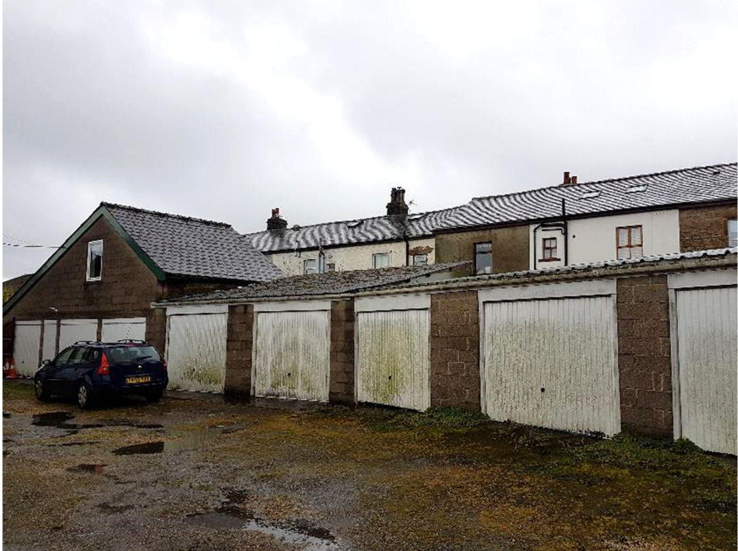
Figure 4: Existing breeze block and sheet roof garages
