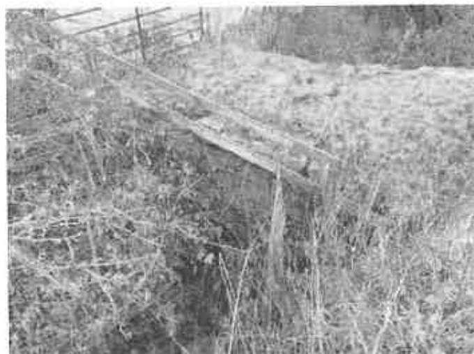
Photograph - Existing culvert and Higgin Brook
