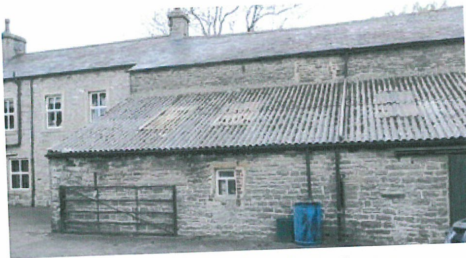
Photograph (6 & 7) – South elevation
