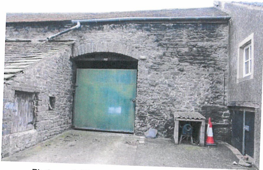
Photograph (5) Lean -to Return and cart opening
