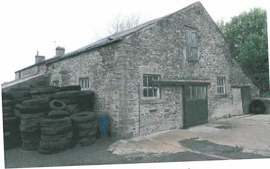
Photograph (3) – East elevation
