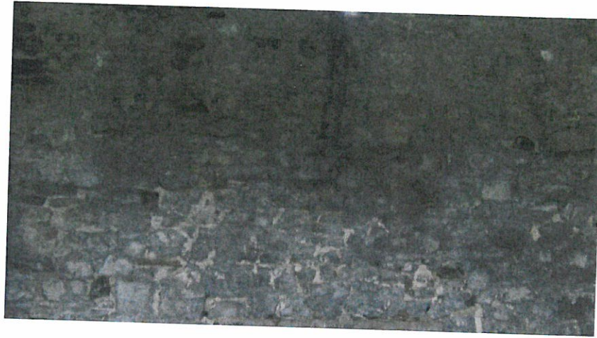
Photography (10) – Internal wall
