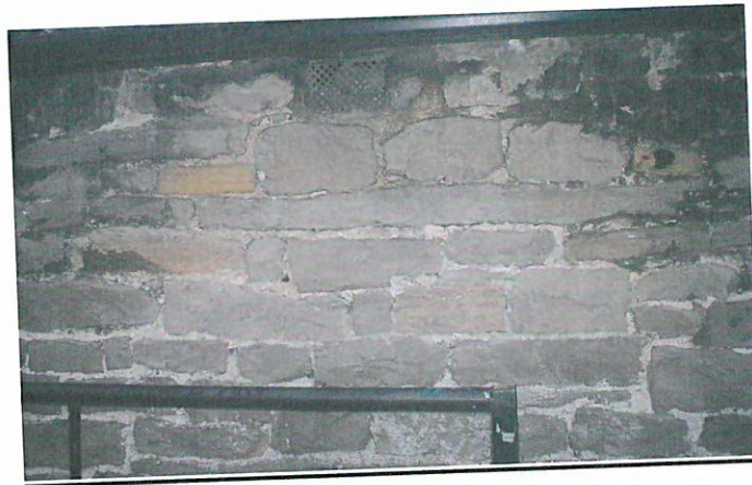
Photograph (8) – Stone detail on south elevation
