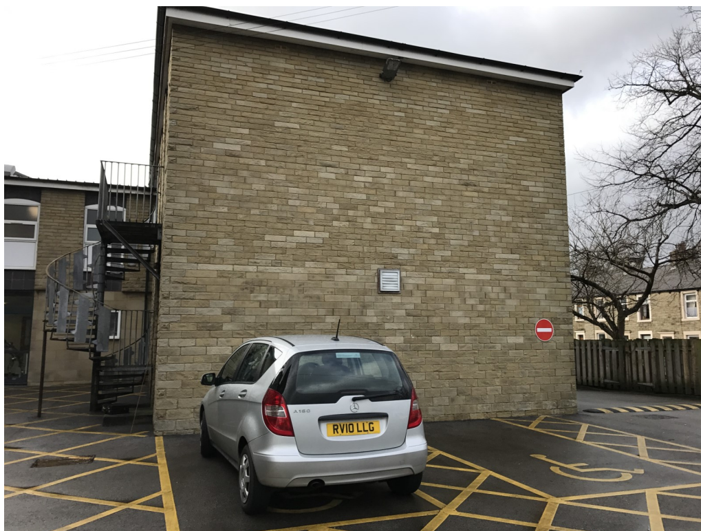
View of existing staircase looking west
