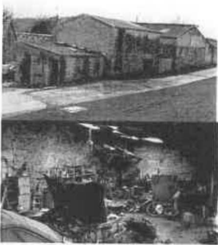
Figure 17: Dairy sheds -- group 'B'
