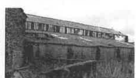
Figure 22: cubicle sheds (east)
