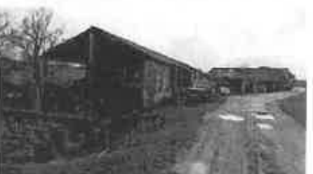
Figure 25: cubicle sheds (west)
