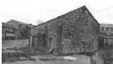
Figure 21: stone barn (east)
