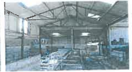
Figure 10: steel-framed cubicle sheds group 'A'
