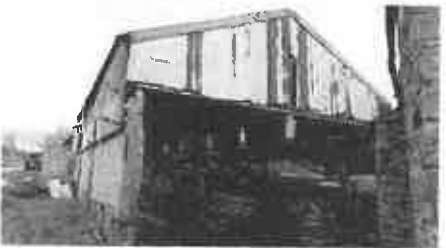
Figure 23: cubicle sheds (east)
