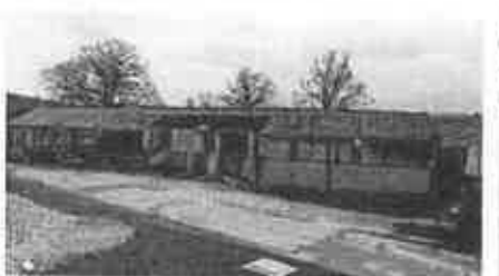
Figure 24: cubicle sheds (east)
