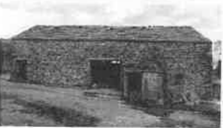
Figure 20: Stone barn (east)
