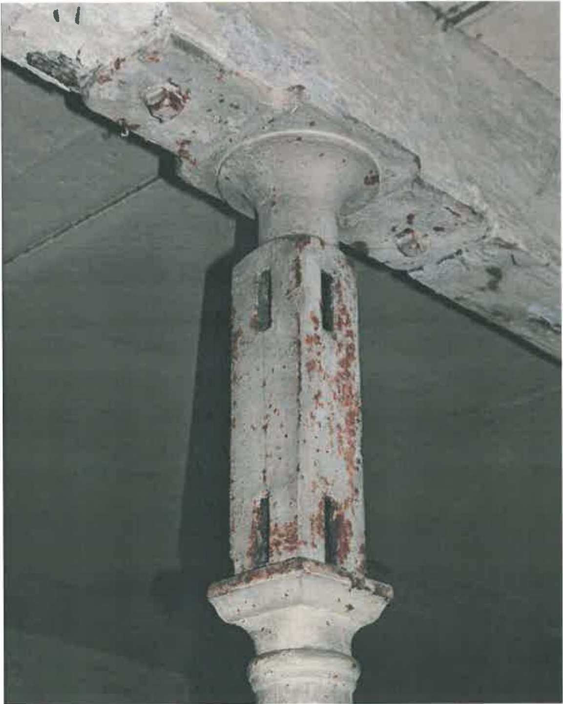
Plate 21: Inserted column with double bolting plate
