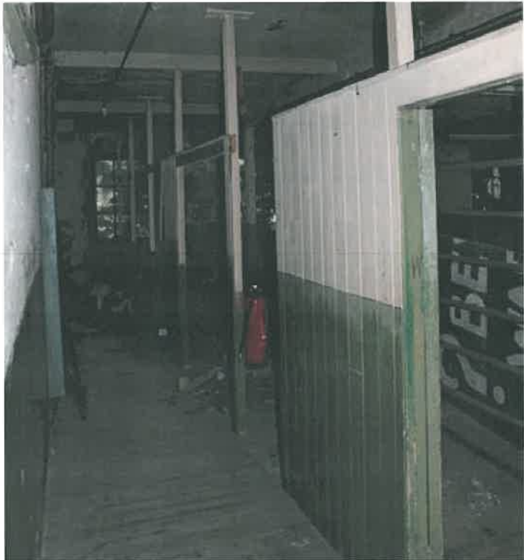
Plate 41: Timber plank partition on first floor of 1823 mill
