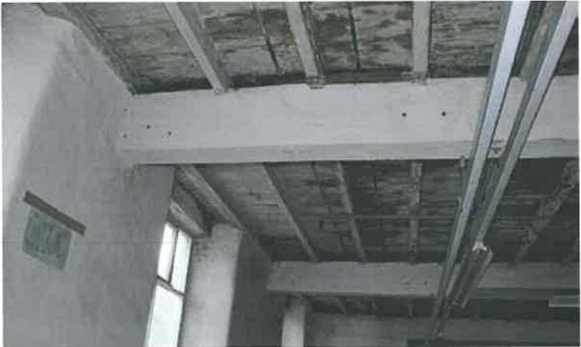
Plate 65: Bolt holes and scars denoting position of line shaft, New Mill
