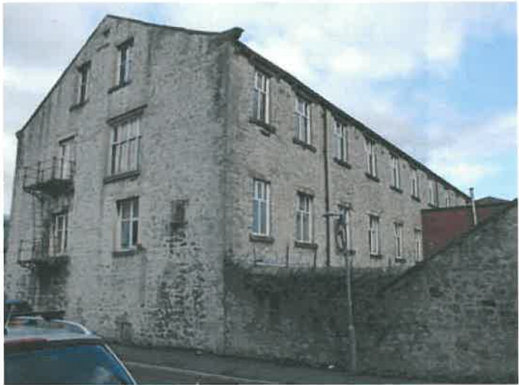
Plate 46: General view of New Mill from Woone Lane
