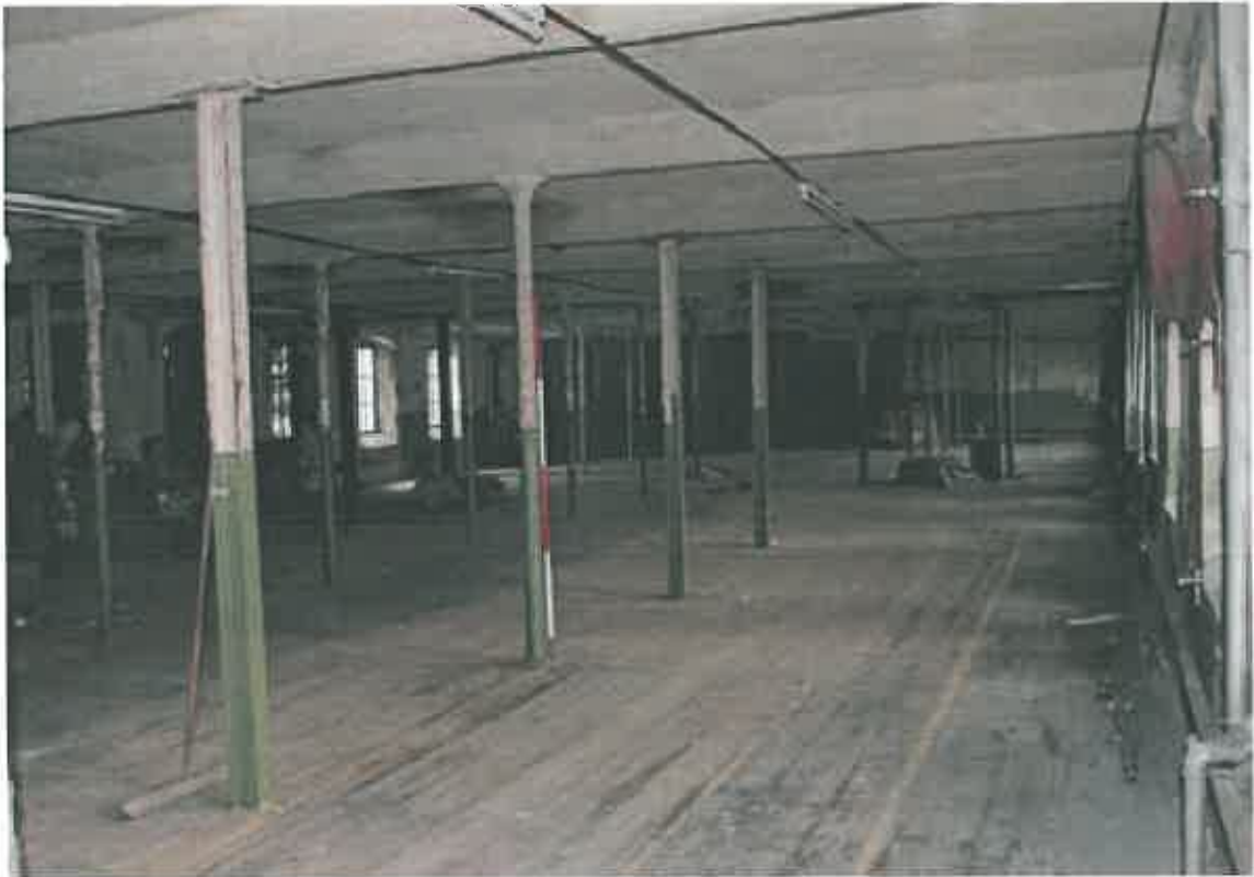
Plate 18: General view of first floor, with replacement cylindrical and I-section columns
