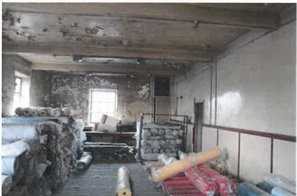
Plate 26: Upper floor of original mill engine house
