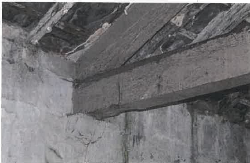
Plate 107: Corbel carrying truss
