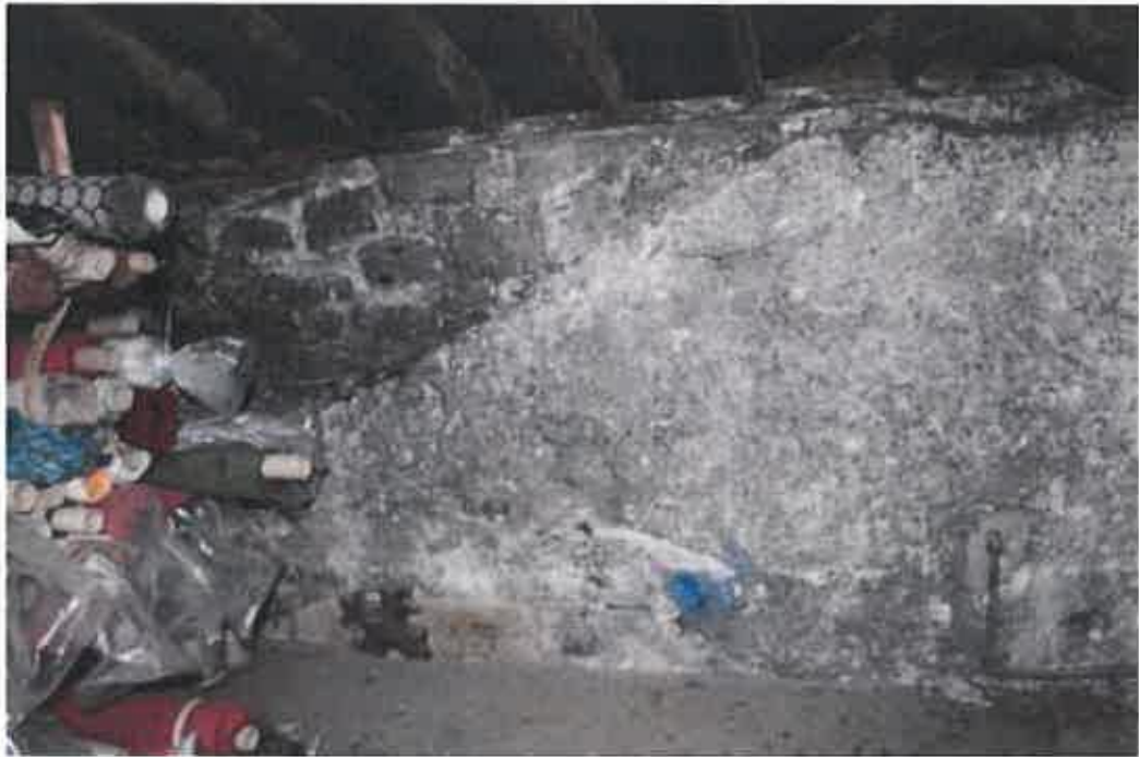
Plate 49: Scar for original roof line of stair tower
