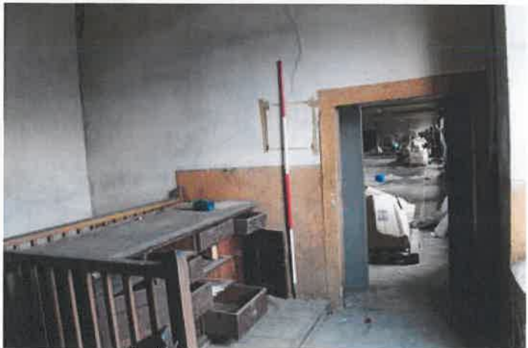
Plate 29: Open landing to upper floor of original mill
