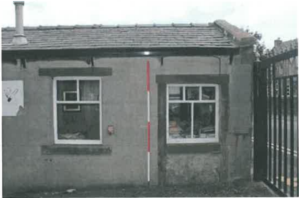
Plate 118: Remodelled doorway, and original window aperture
