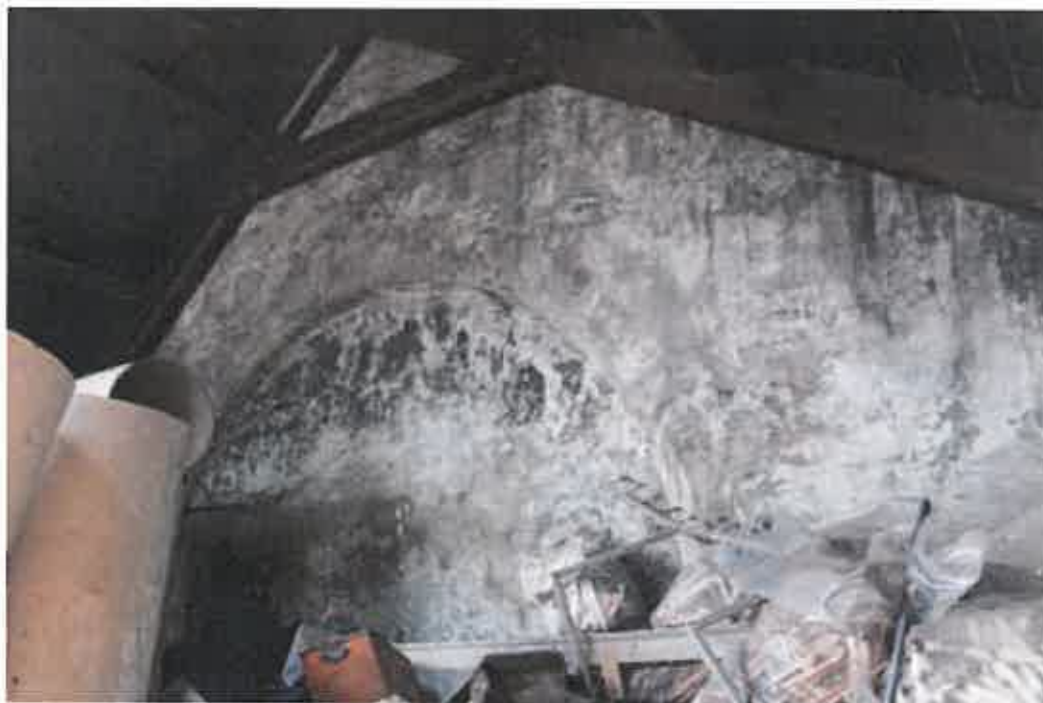
Plate 91: Arched aperture in west gable of engine house
