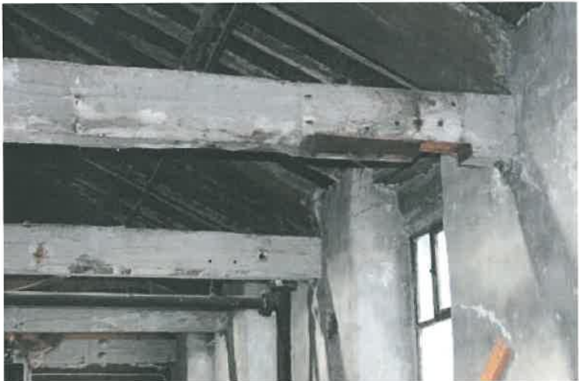
Plate 66: Bolt holes and scars denoting position of line shaft, second floor, New Mill
