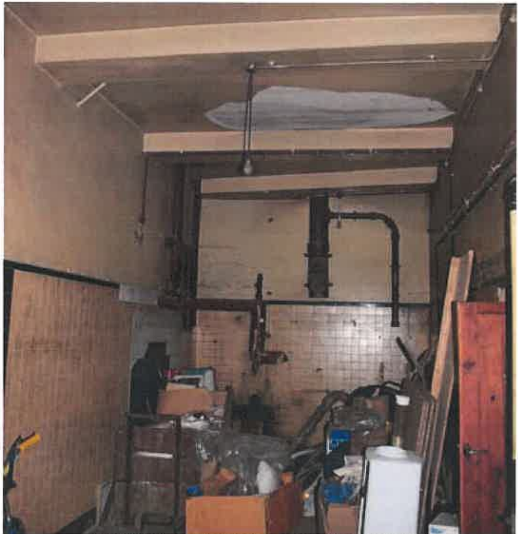
Plate 25: Remodelled engine house, ground floor, original mill
