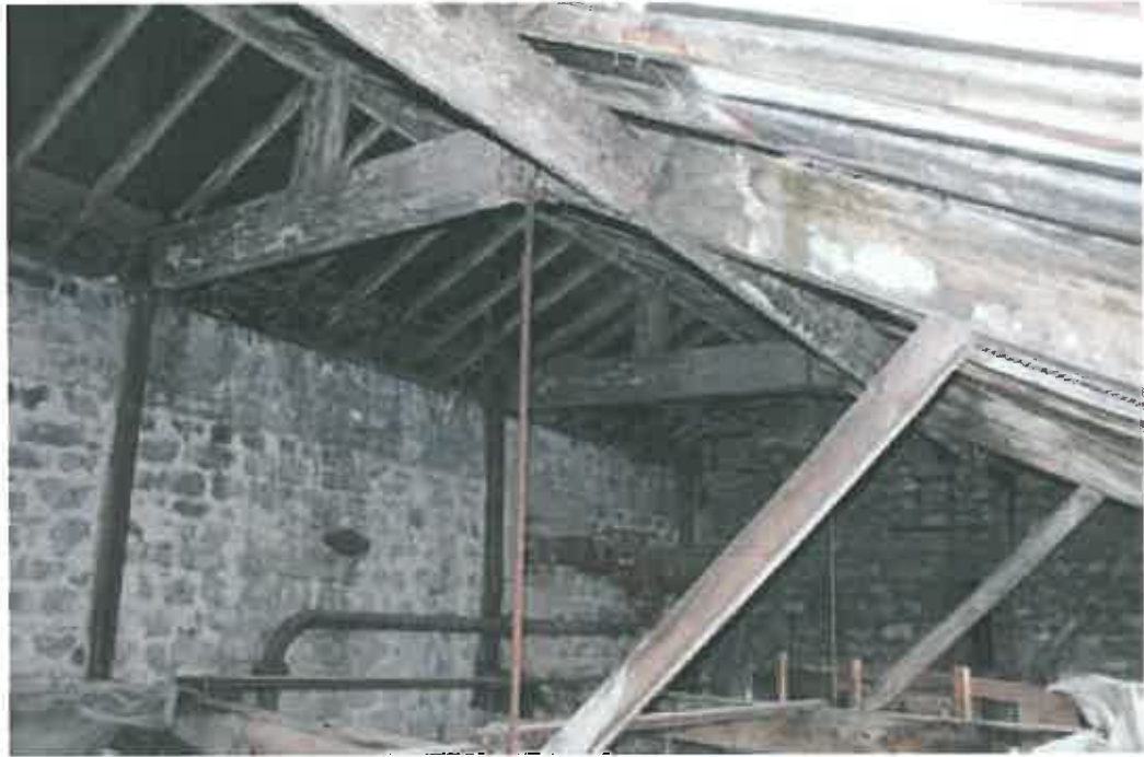
Plate 109: Remodelled trusses adjacent to 1910 engine house
