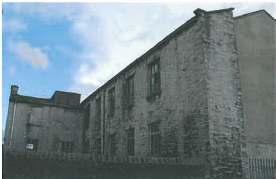
Plate 7: North wall of original spinning block, with projecting privy tower and later hoist tower
