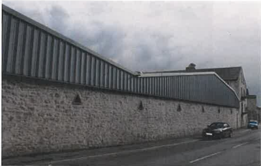
Plate 110: West wall of weaving shed
