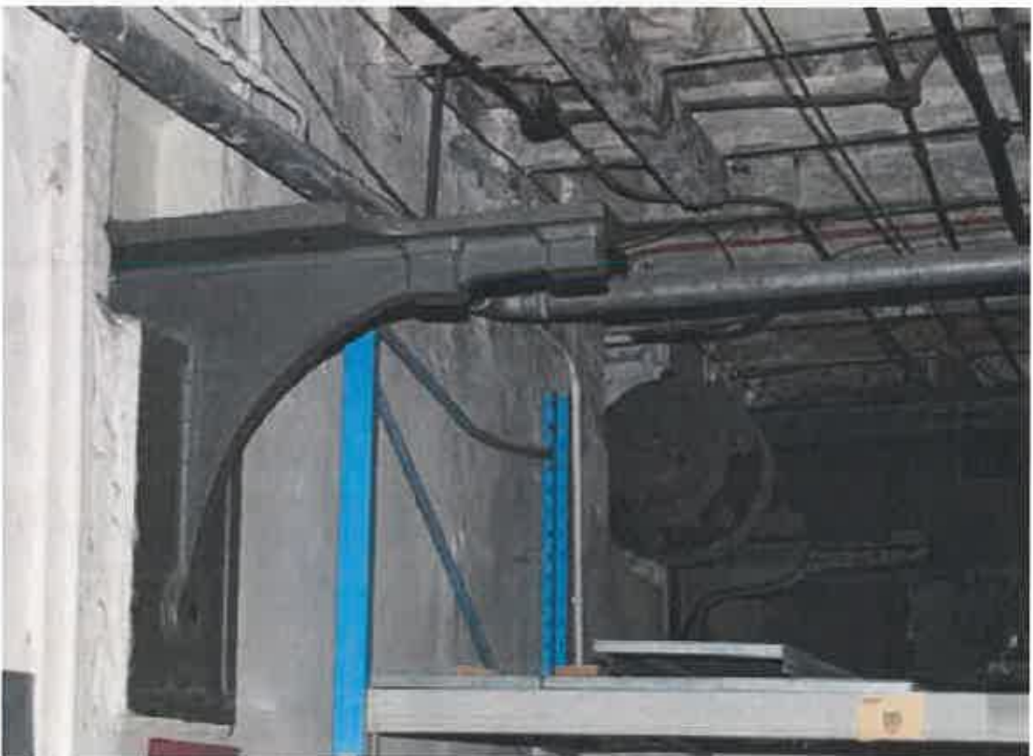
Plate 58: Cast-iron corbel carrying secondary shaft to weaving shed
