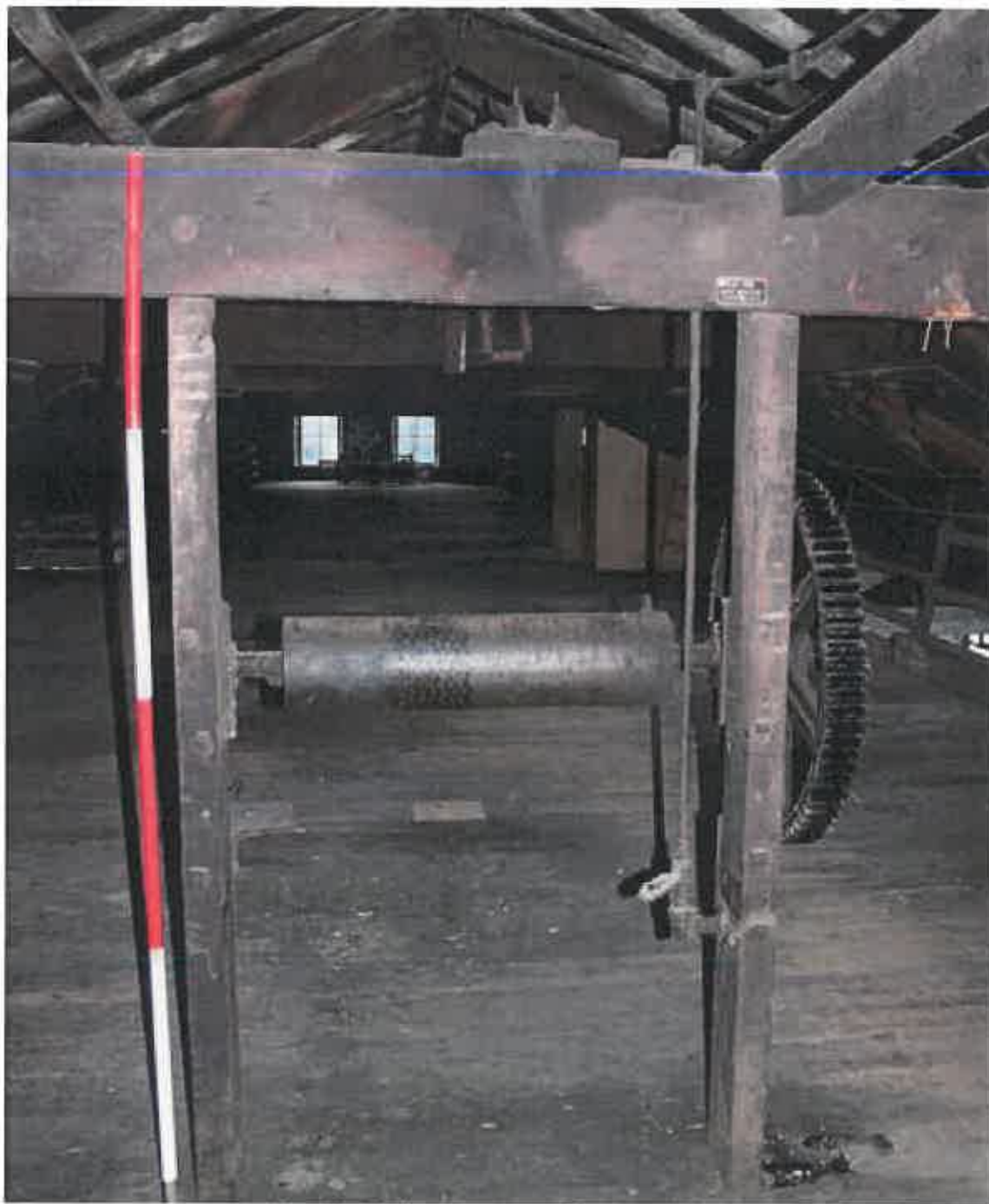
Plate 51: Winding gear in attic for New Mill hoist
