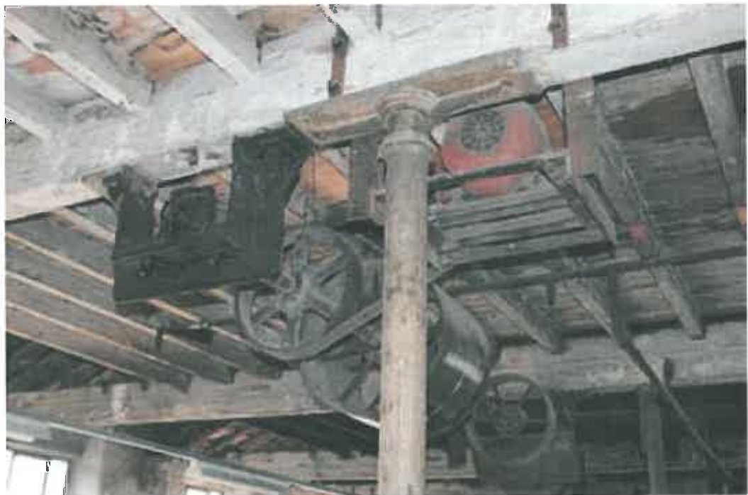
Plate 69: Central line shaft on second floor, with added electric motor
