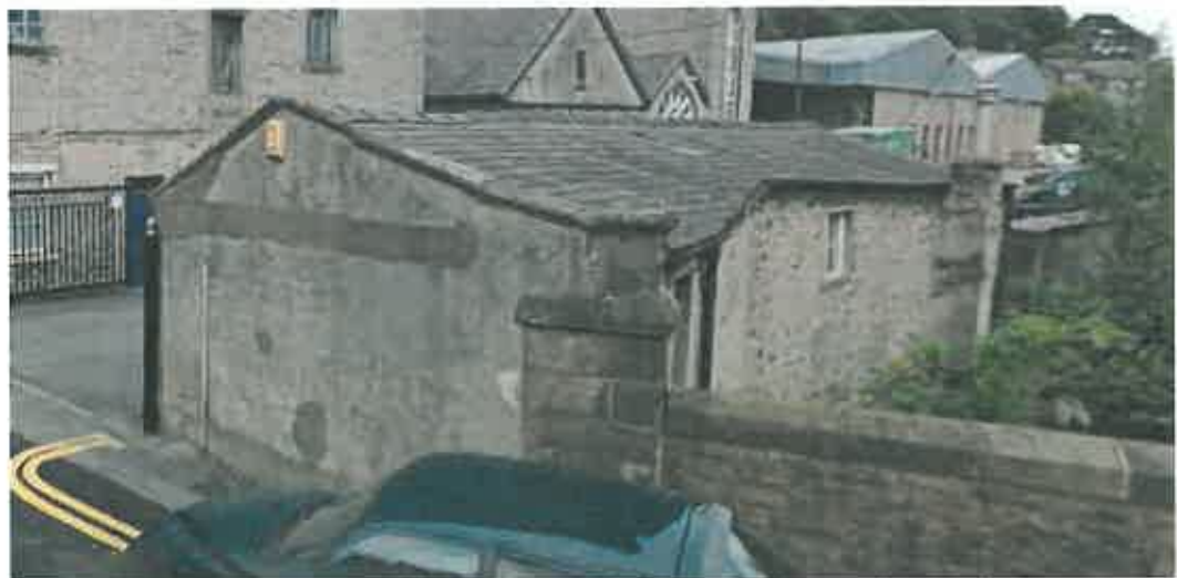
Plate 119: Rear of gatehouse, with chimney stack at northern end
