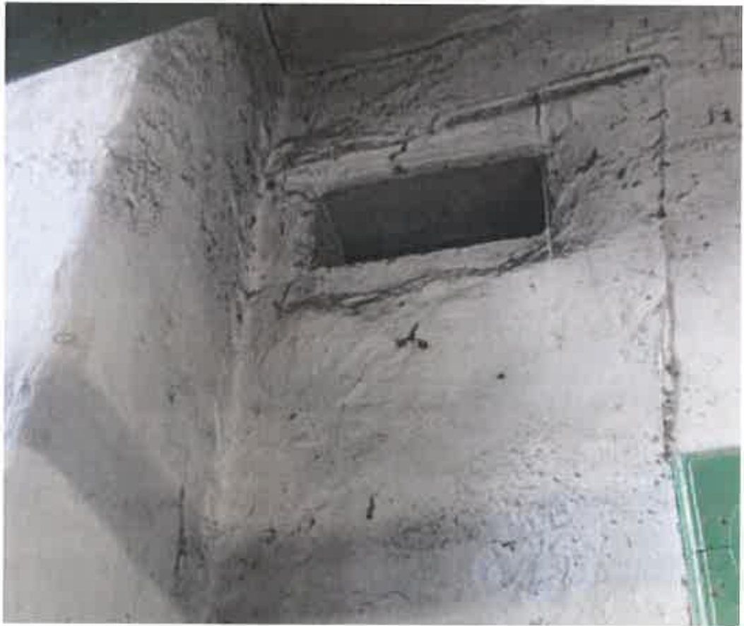
Plate 64: End bearing box adjacent to south wall, for line shaft, ground floor, New Mill
