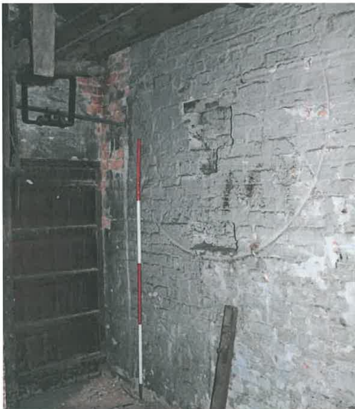
Plate 50: Scars for winding drums at upper floor level of New Mill hoist
