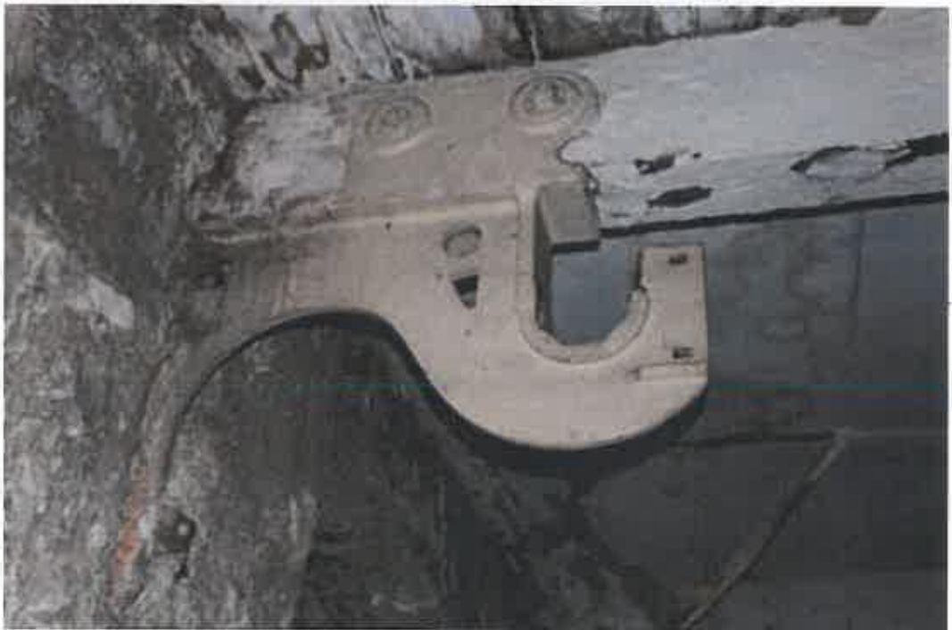
Plate 43: Line shaft hanger adjacent to south wall of 1823 spinning block
