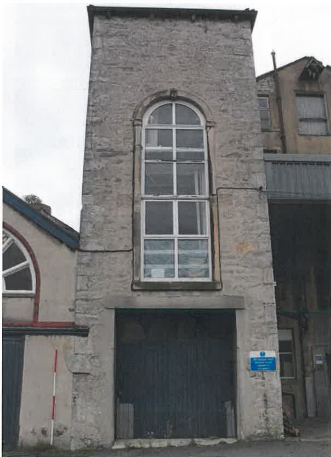
Plate 78: New Mill original beam engine house
