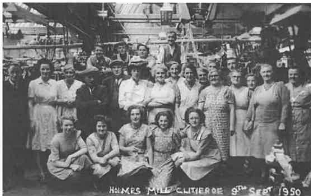
Plate 3: New Mill weaving shed in 1950, shortly prior to its internal refurbishment
