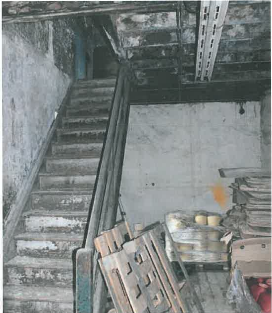
Plate 38: Stair within hoist tower
