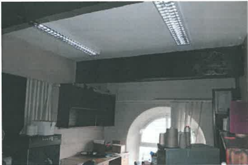
Plate 82: Large roof timbers of beam engine house
