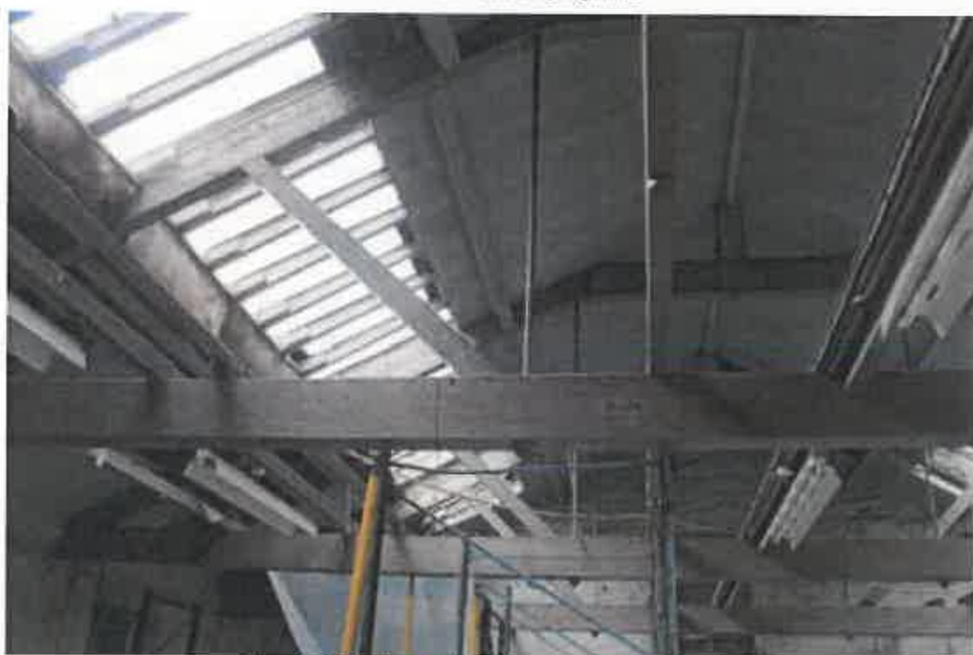
Plate 108: Timber and metal trusses of warehouse
