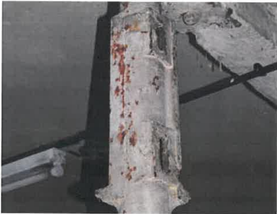
Plate 22: Through bolt-holes on double-plated column
