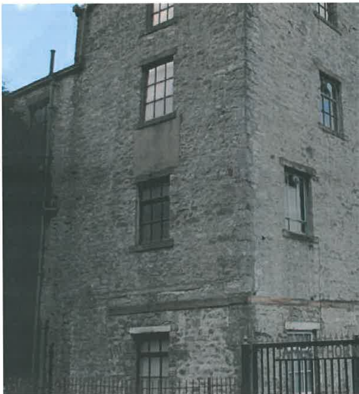
Plate 13: Butt joint of eastern jamb of engine house window, and arch of boiler house aperture
