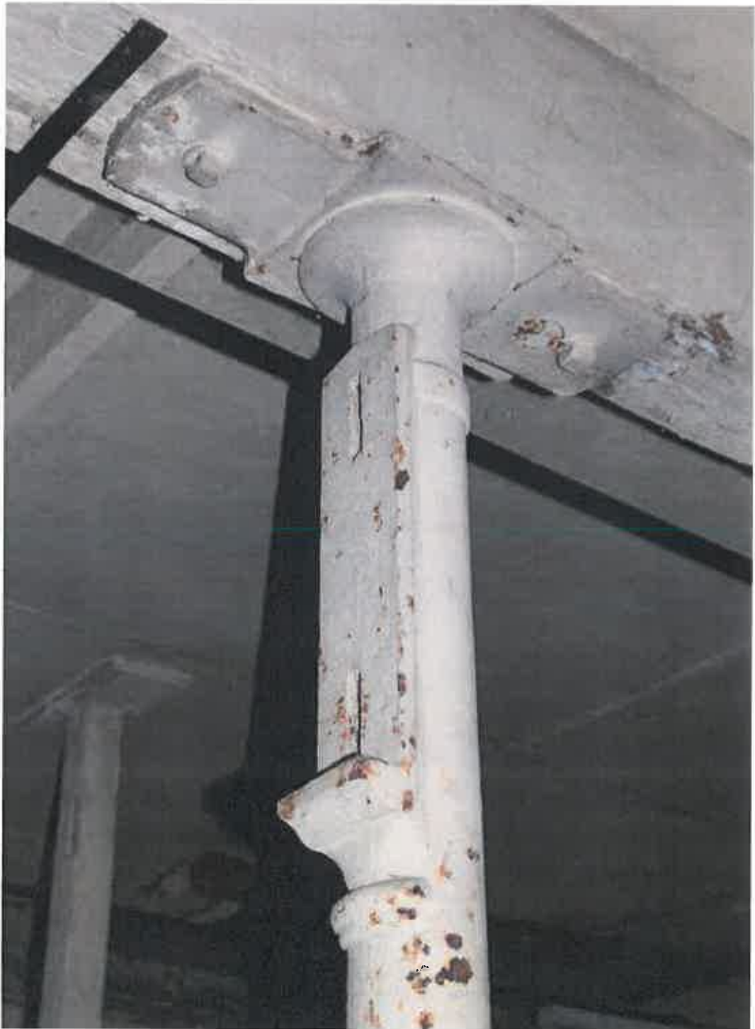
Plate 20: Inserted hollow cylindrical column with bolting plate
