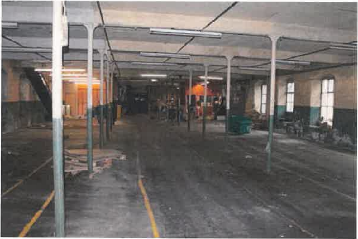
Plate 16: Ground floor of 1823 mill
