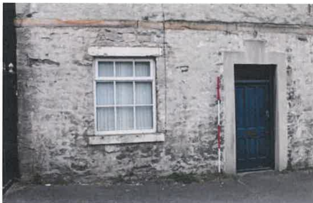
Plate 14: Doorway and remodelled window in east gable of 1823 mill
