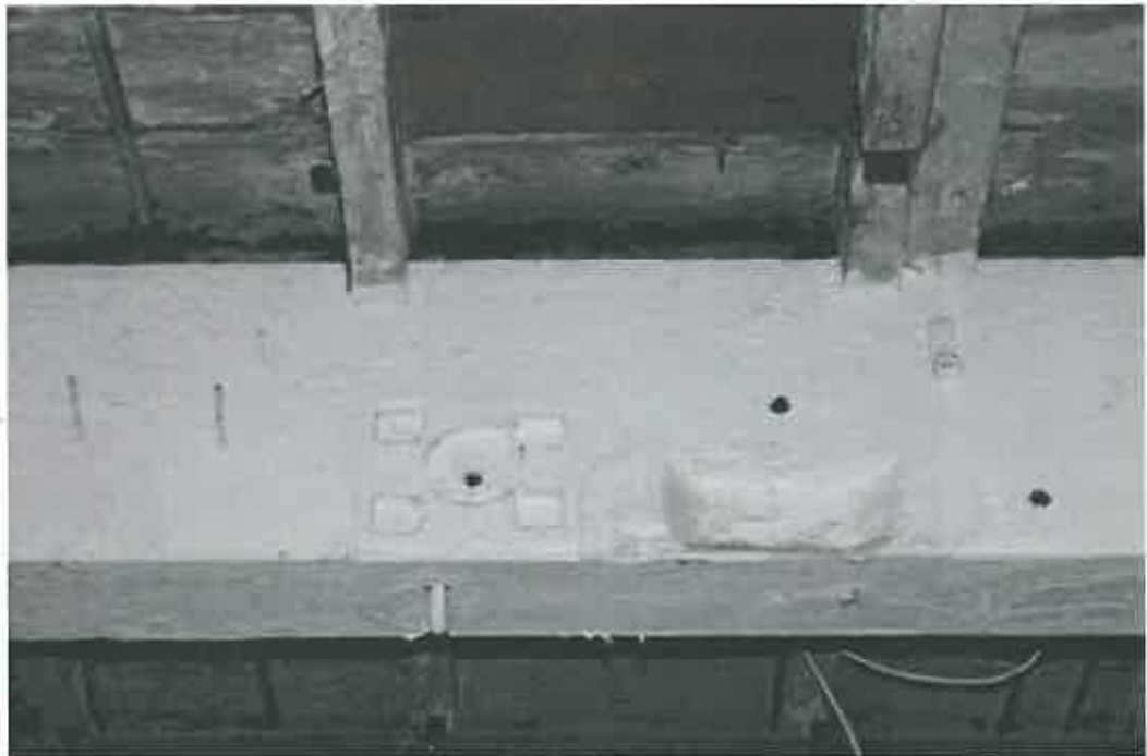
Plate 62: Bolt and cut-out denoting position of earlier line shaft, New Mill
