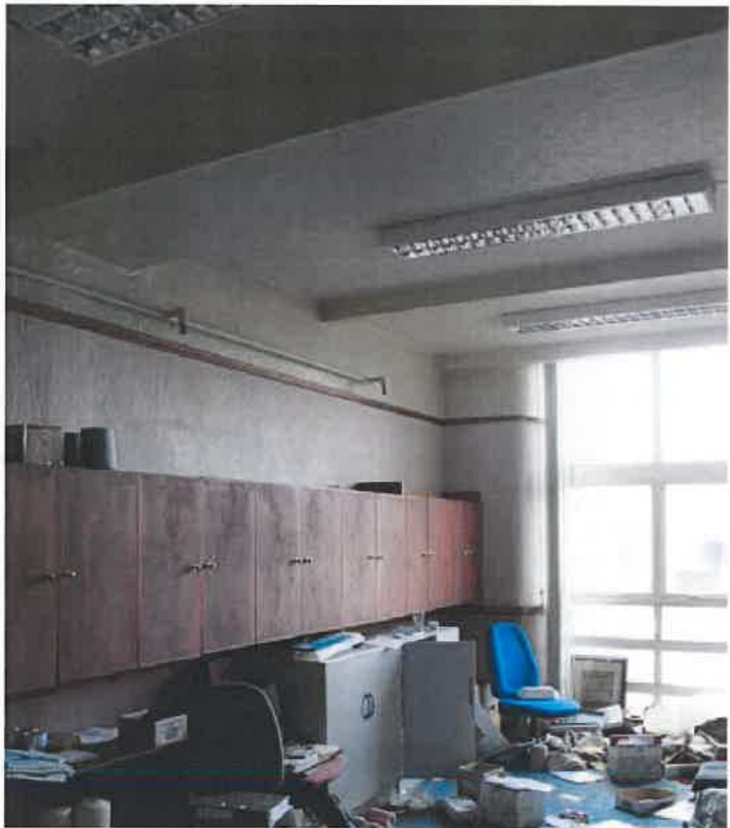
Plate 81: Office inserted into beam engine house, with enclosed entablature beam within ceiling
