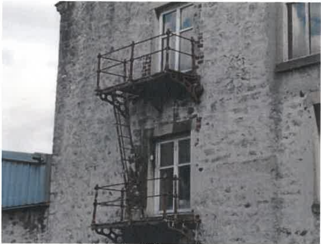
Plate 74: New Mill fire escape, added 1913
