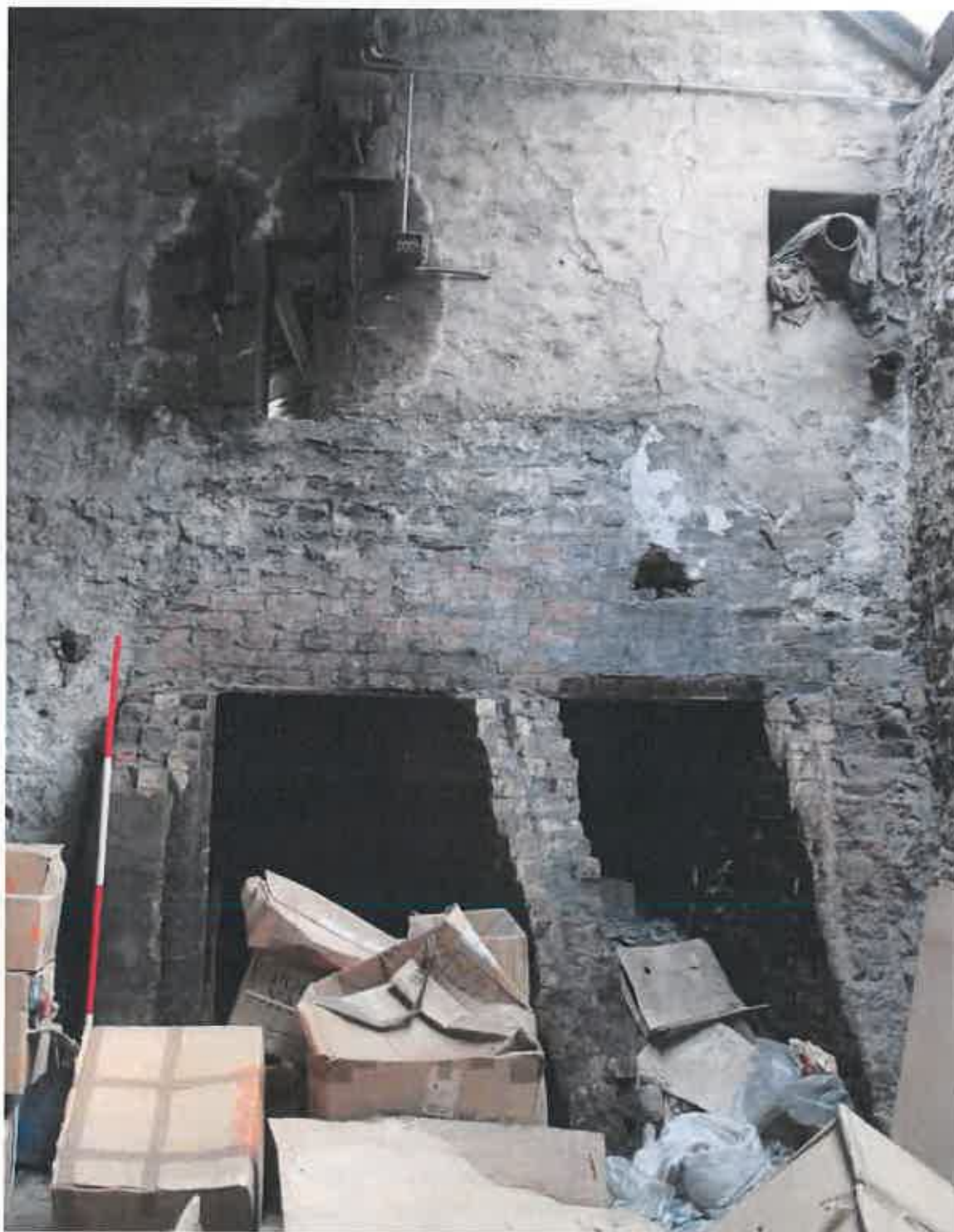
Plate 85: Flues and damper aperture at rear of boiler house
