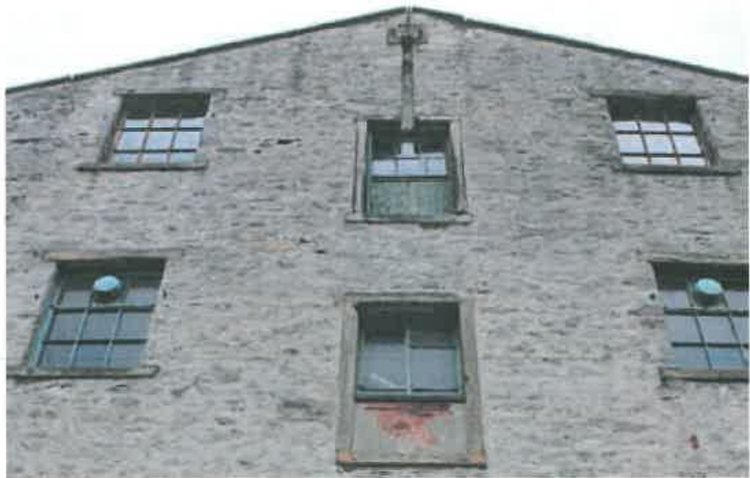
Plate 15: Loading loophole in east gable of 1823 mill
