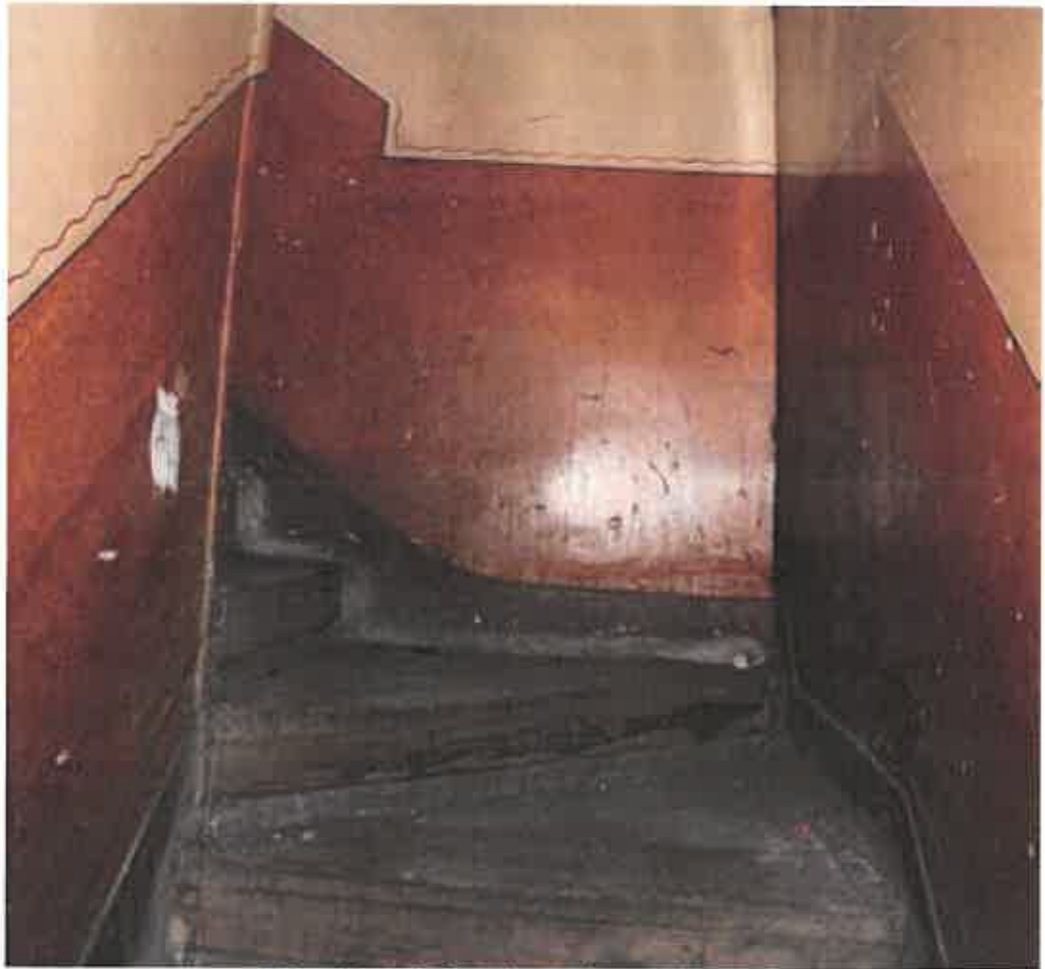
Plate 28: Angled winders in fireproof stair tower
