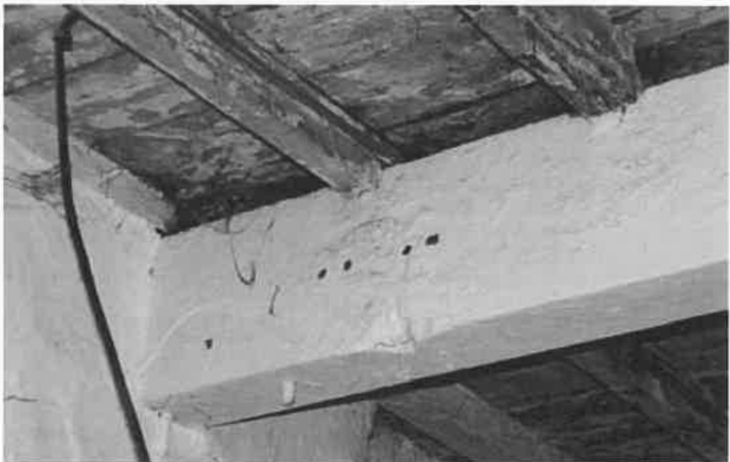
Plate 61: Bolt and scar of earlier line shaft hanger, New Mill
