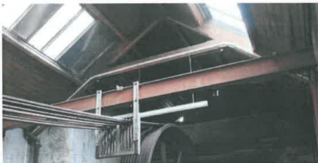
Plate 89: Engine house roof detail
