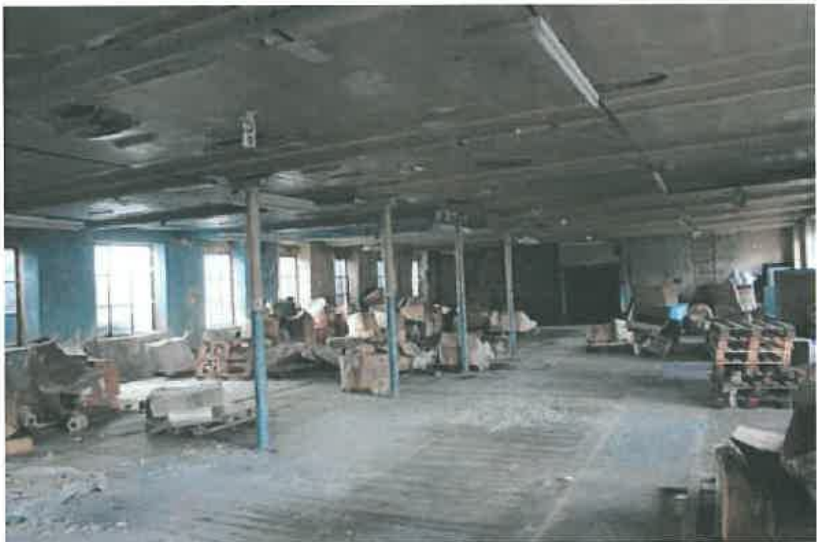
Plate 19: General view of second floor with replacement columns, and scars for original double row of columns
