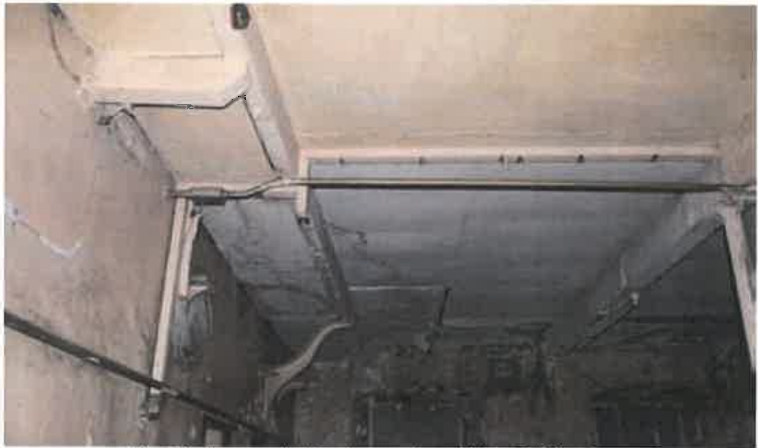
Plate 42: Swan-necked bearing carrying additional ceiling beam
