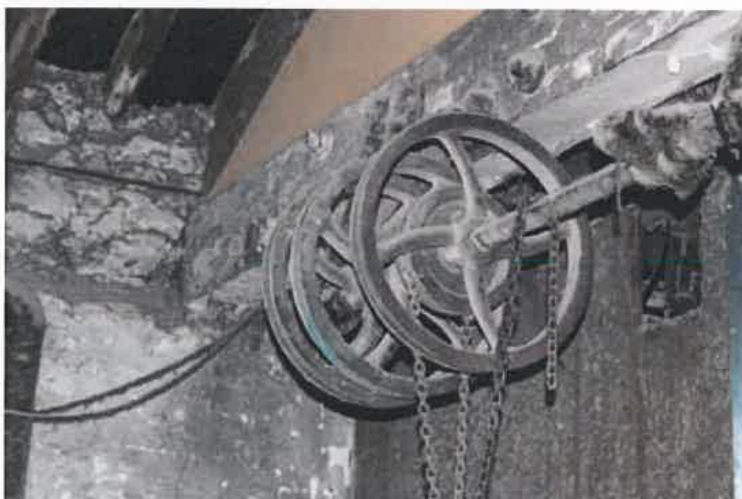
Plate 71: Line shaft with slender rope wheels, possibly for safety chain for hoist
