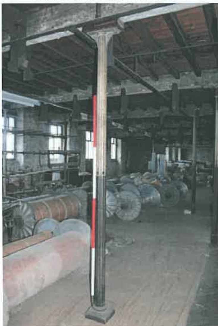
Plate 53: Fluted column on second floor of New Mill
