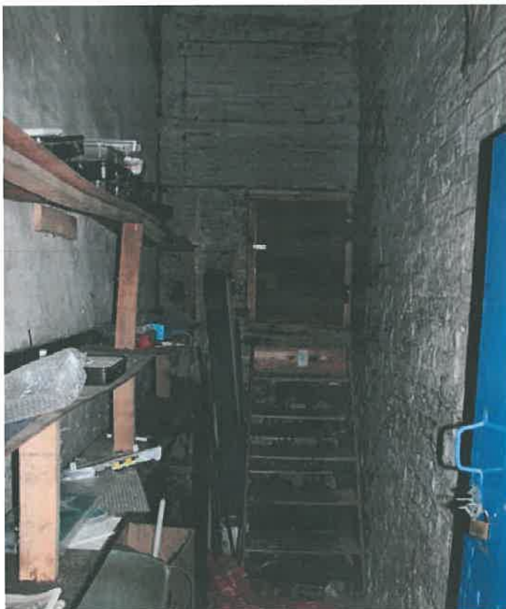
Plate 48: Store to west of stairwell, with roof access at second-floor level
