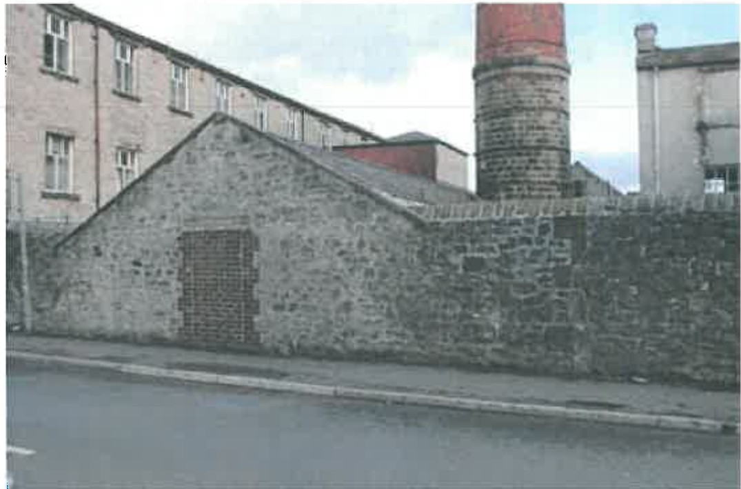
Plate 104: Single-storey warehouse, with blocked access from Woone Lane
