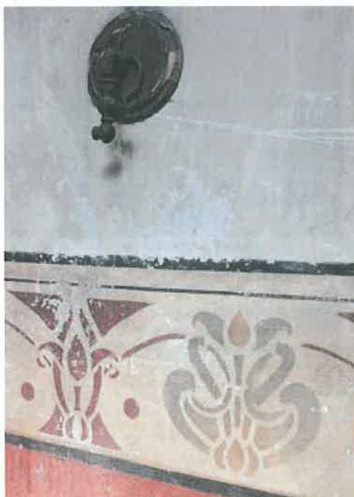
Plate 96: Painted plasterwork and extant gas tap in engine house
