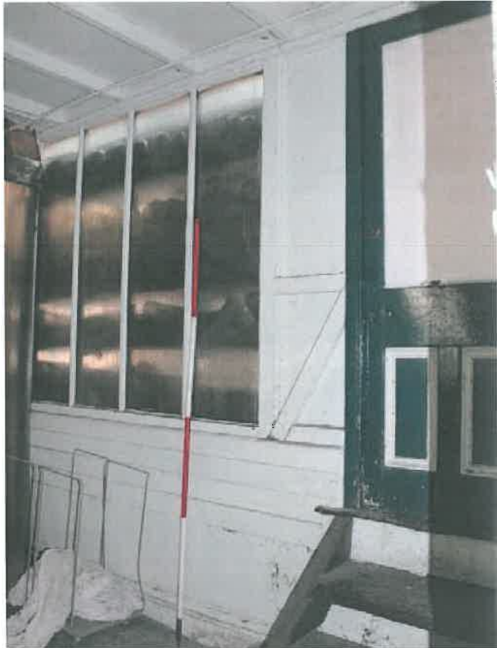
Plate 93: Timber partition and door into engine house
