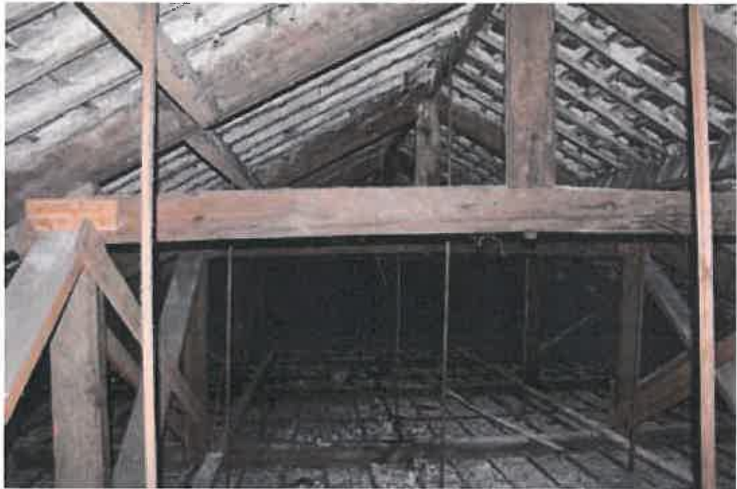
Plate 39: Roof structure within original spinning block
