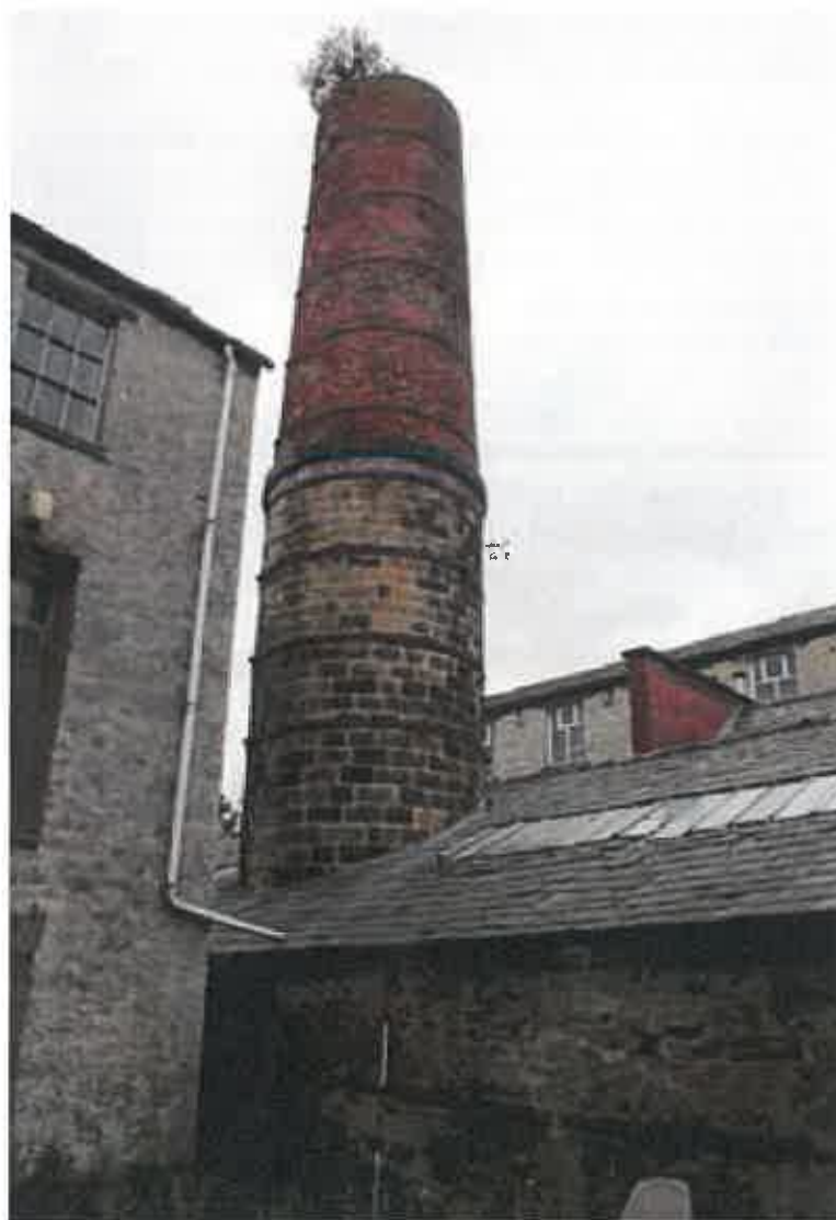
Plate 84: Two-phase chimney, with sandstone flag capping of original flue visible within wall
