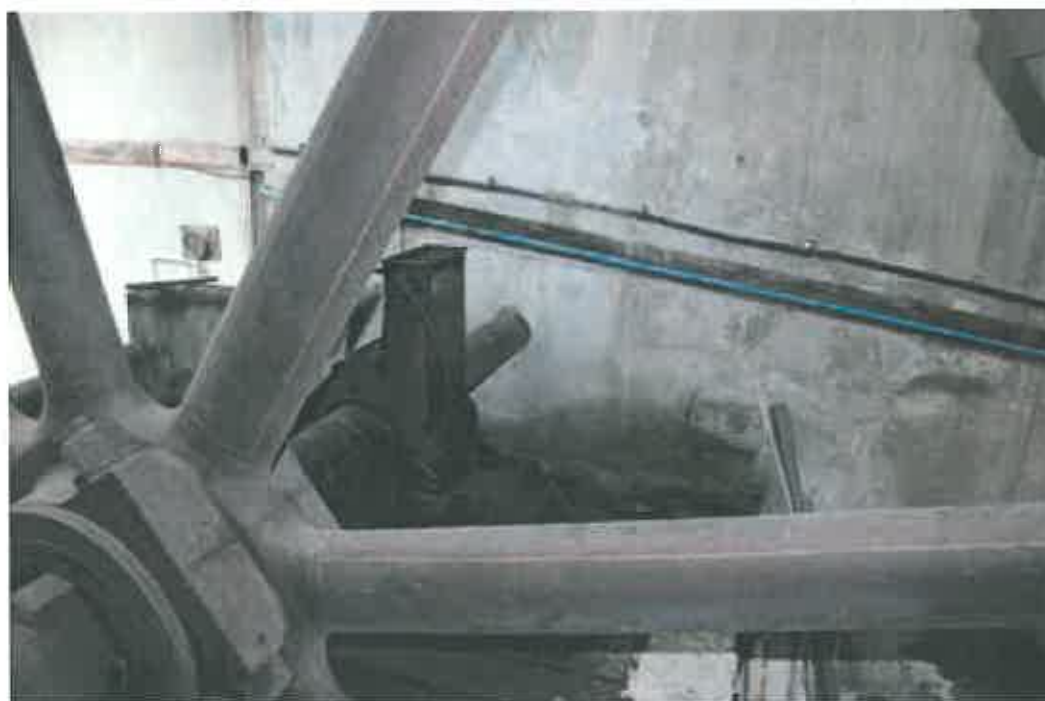
Plate 102: Secondary motion shaft, and corbel for earlier boiler house truss
