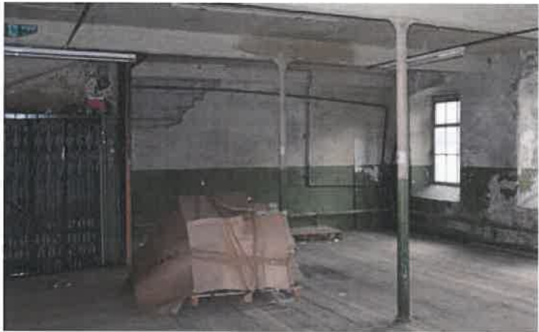
Plate 10: Internal view of west gable of 1823 mill, with door to privy tower (right), and inserted hoist, (left)
