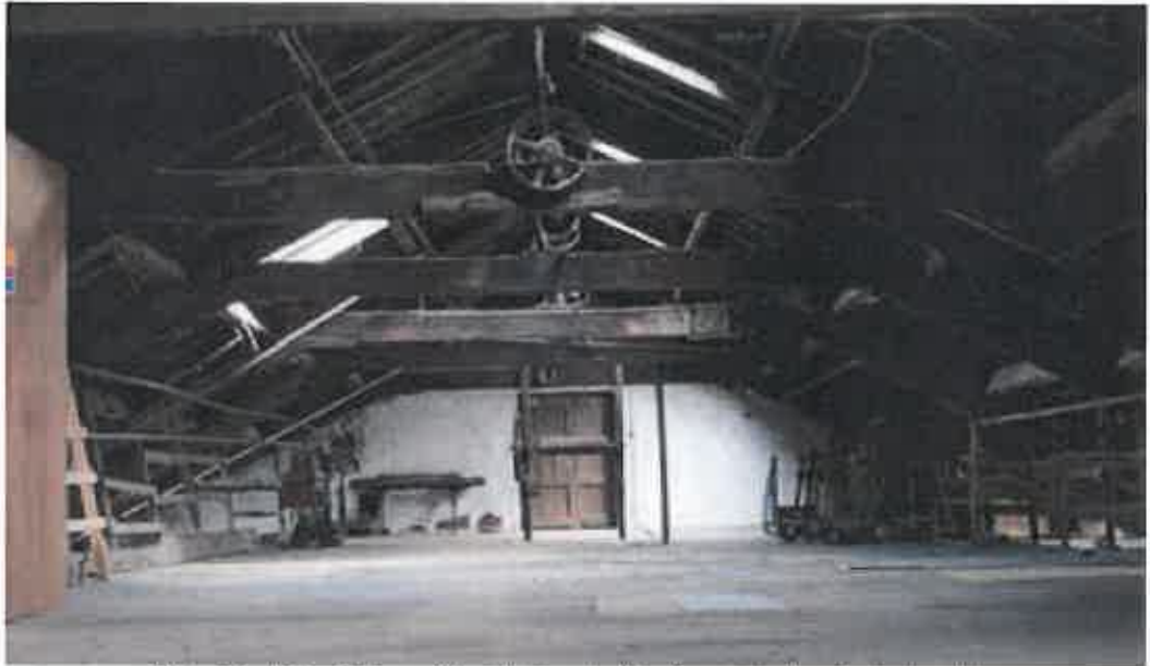
Plate 56: Attic of New mill, with line shaft adjacent to its original position
