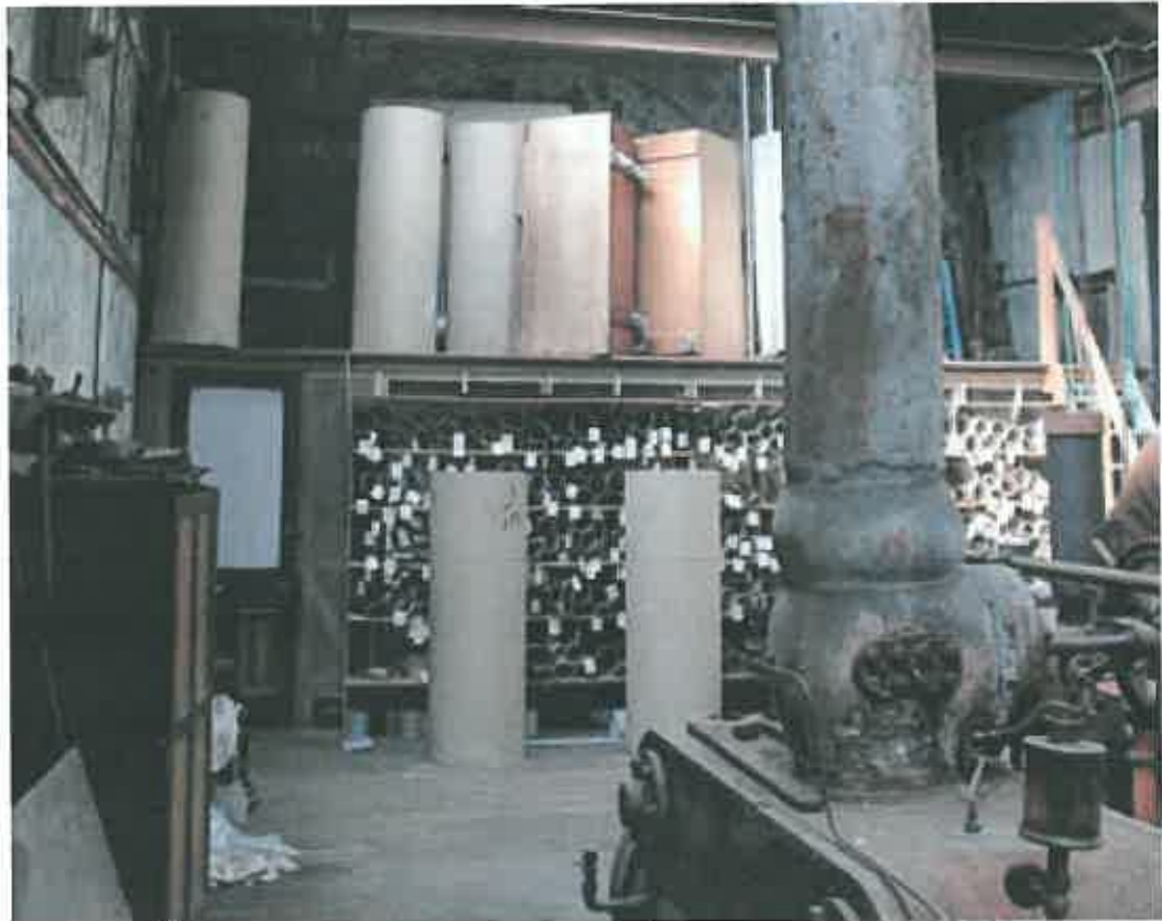
Plate 98: Pigeon holes against timber partition in west bay of engine house
