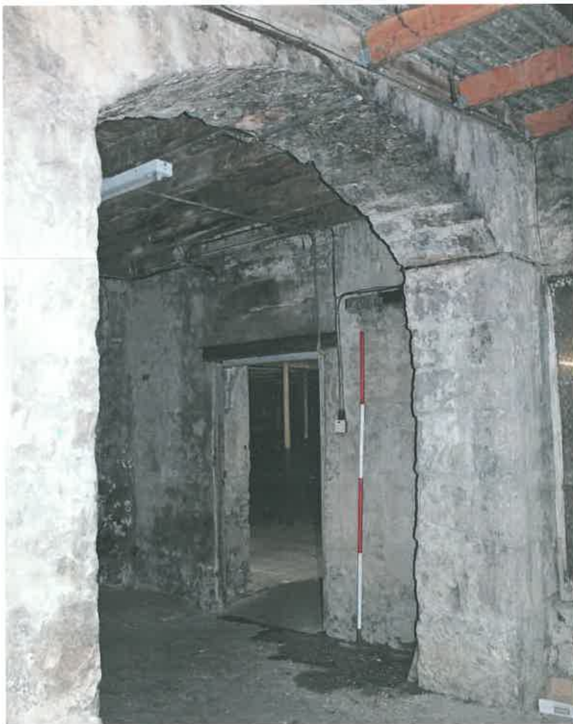
Plate 35: Arched doorway into northern side of hoist tower
