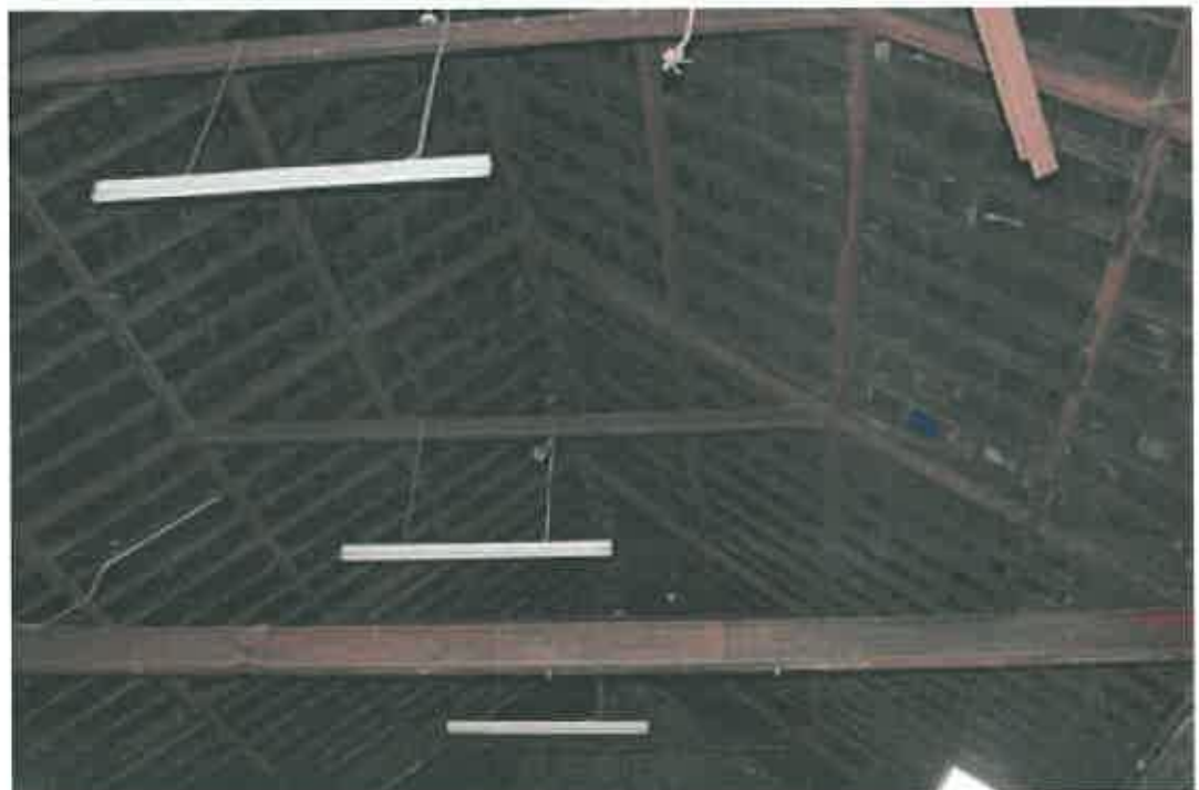
Plate 87: Roof of boiler house
