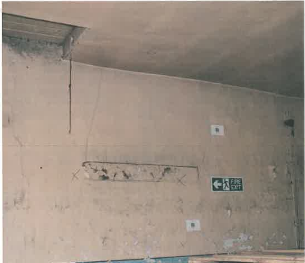
Plate 27: Sandstone pad projecting through wall between engine house and original mill
