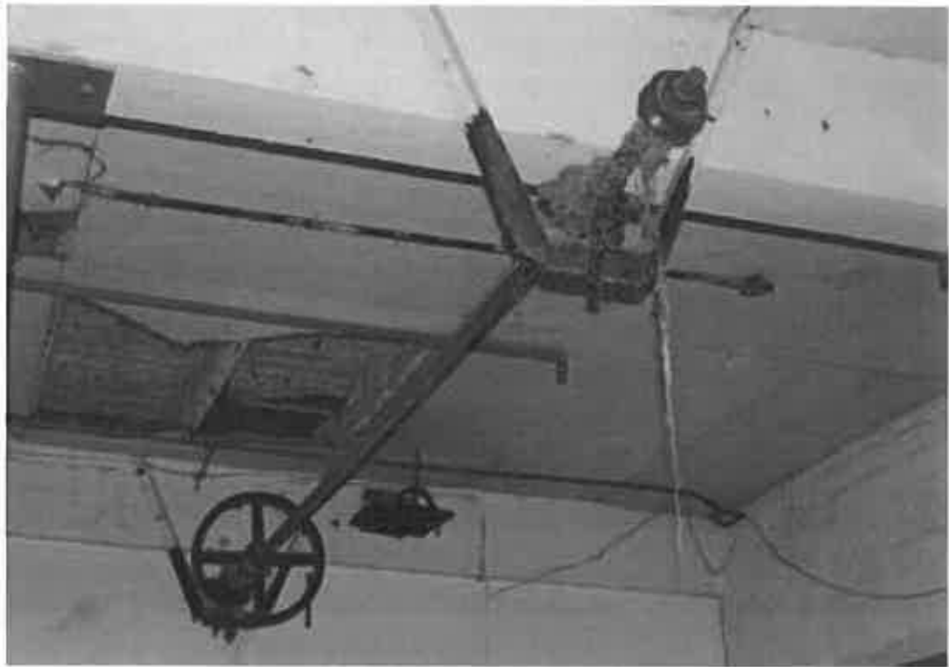
Plate 60: In-situ slender line shaft, ground floor, New Mill
