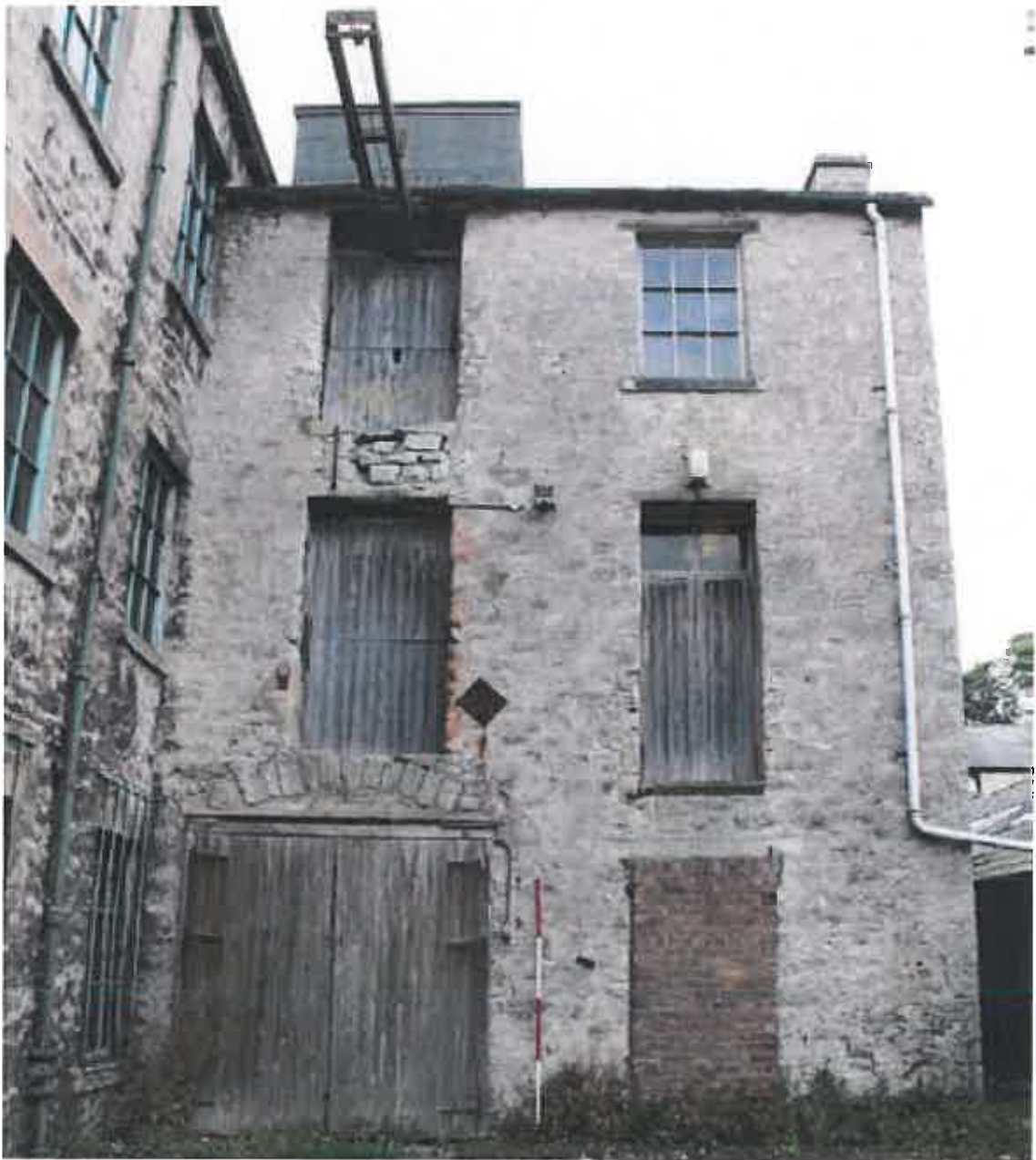
Plate 34: Hoist tower extension to original spinning block
