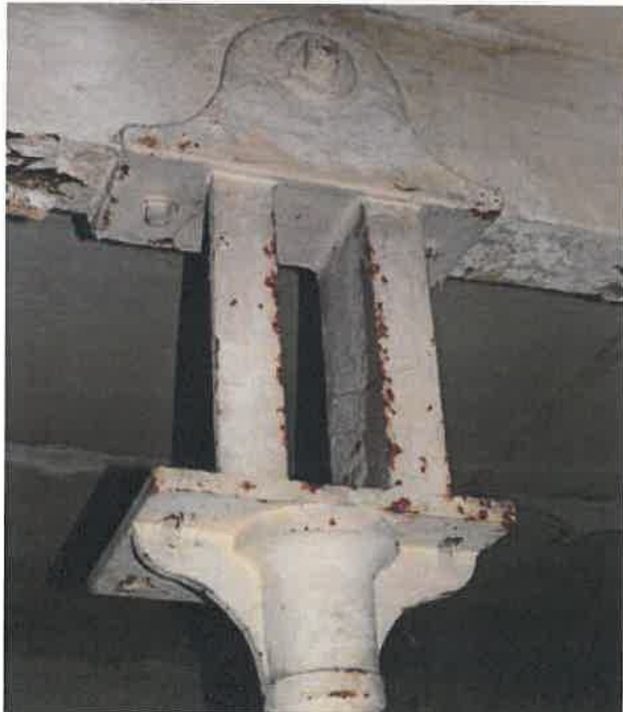
Plate 23: Inserted column with vertical struts allowing shaft to pass through column head
