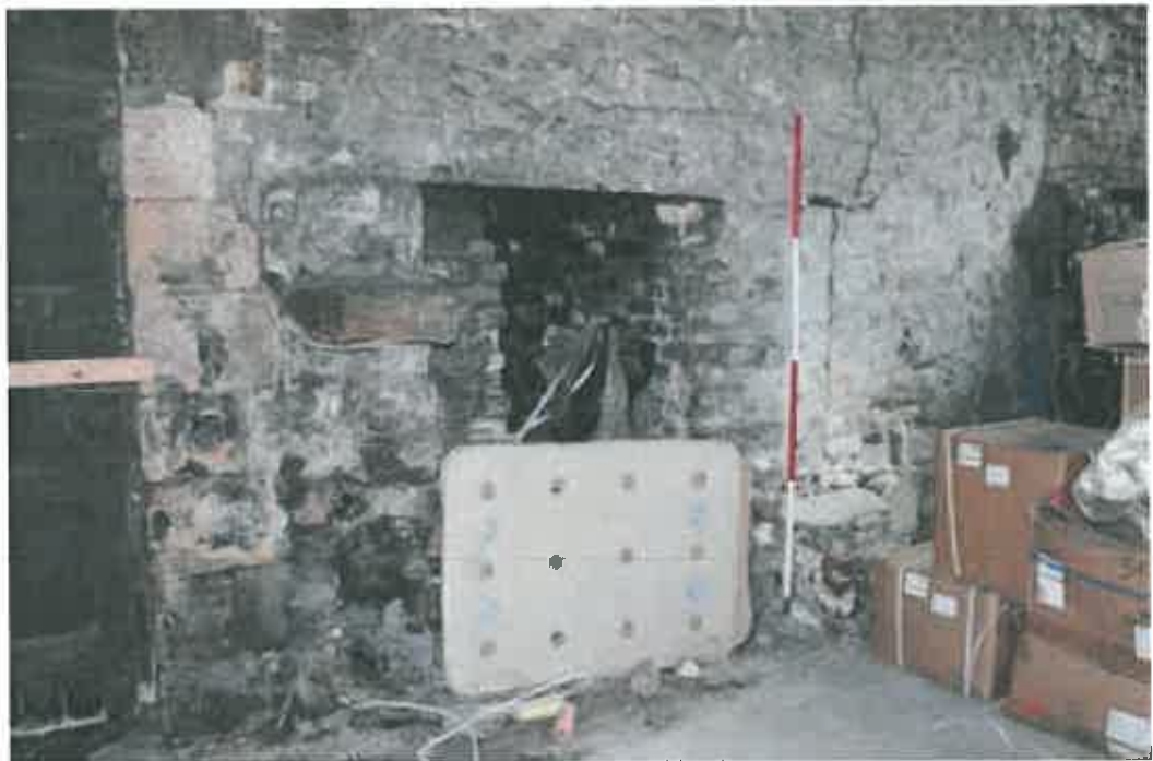
Plate 86: Flue at southern side of boiler house, with spine wall of Lancashire boiler to right
