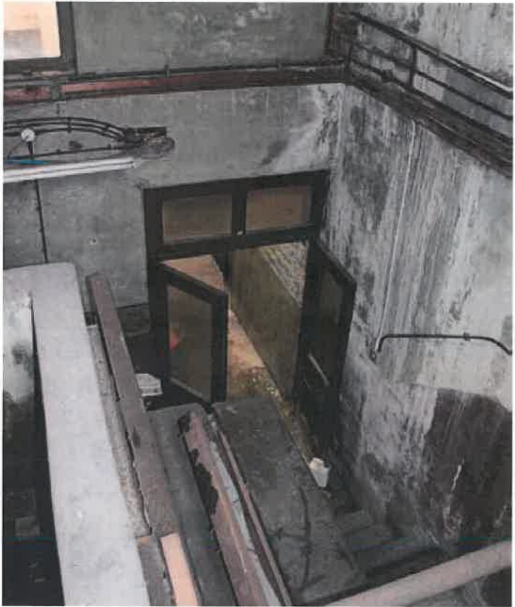
Plate 94: Door and corridor into extension to east of engine house
