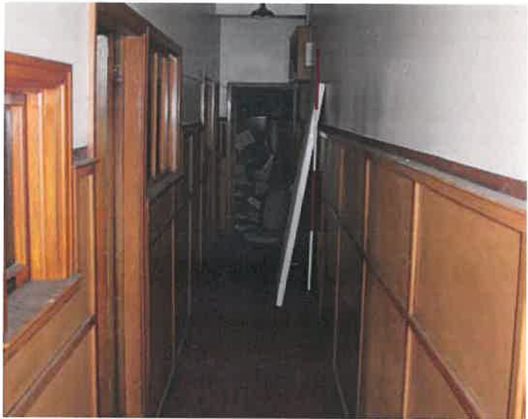
Plate 31: Corridor inserted into first floor of former boiler house
