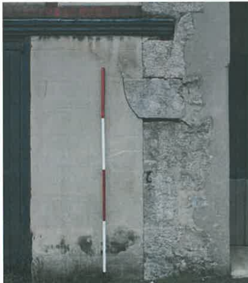
Plate 80: Dressed impost for arched aperture of original boiler house
