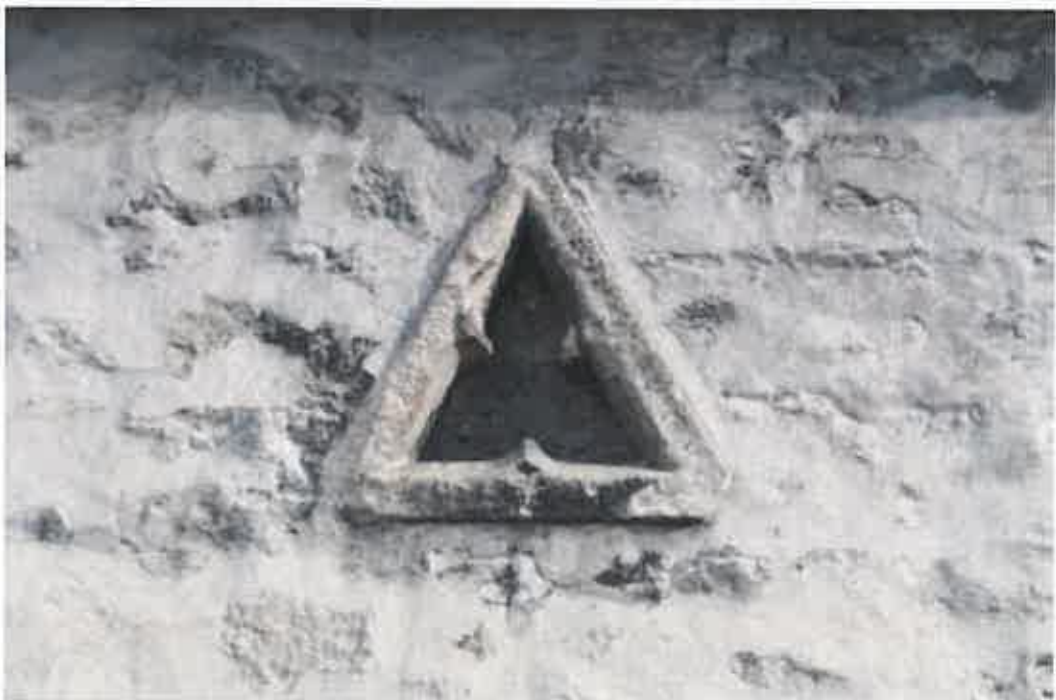
Plate 111: Triangular vent in weaving shed gable
