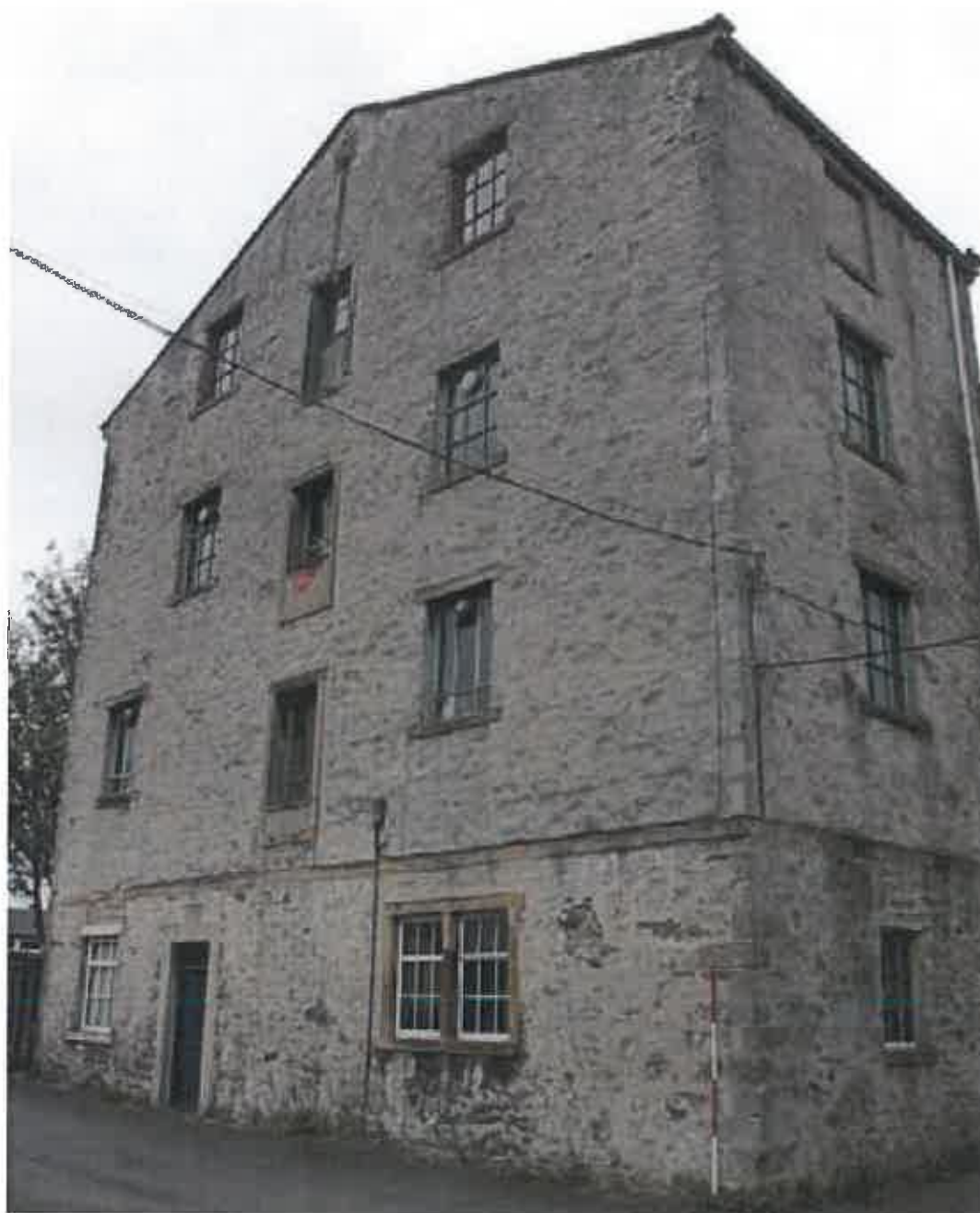
Plate 12: Four-storey tower at east end of 1823 mill
