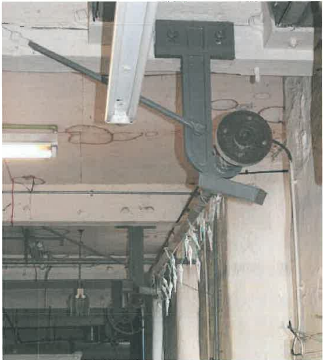
Plate 59: In-situ line shaft and hangers, ground floor, New Mill
