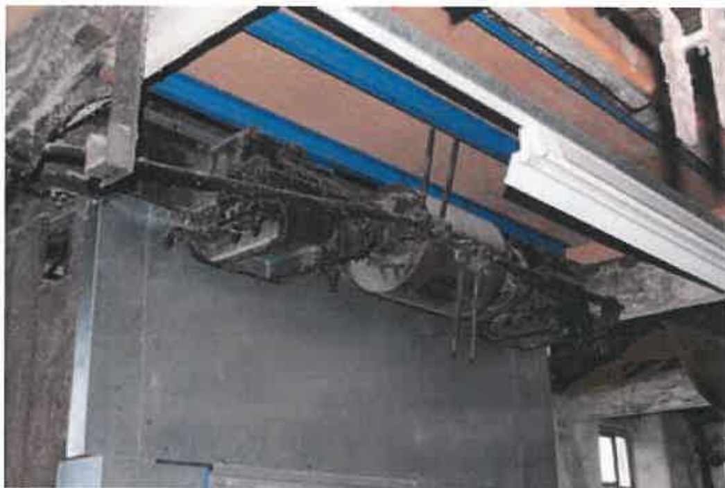
Plate 70: Line shaft for internal hoist tower
