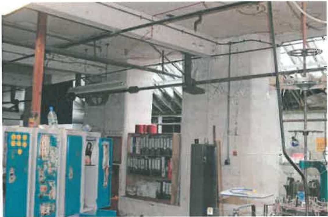
Plate 55: Remodelled apertures in south wall of ground floor in New Mill
