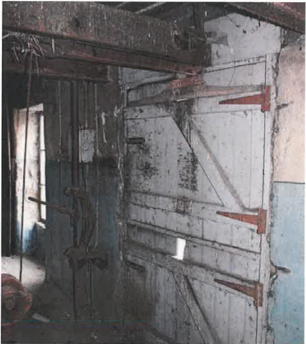
Plate 36: Double door in hoist tower, with original opening mechanism intact
