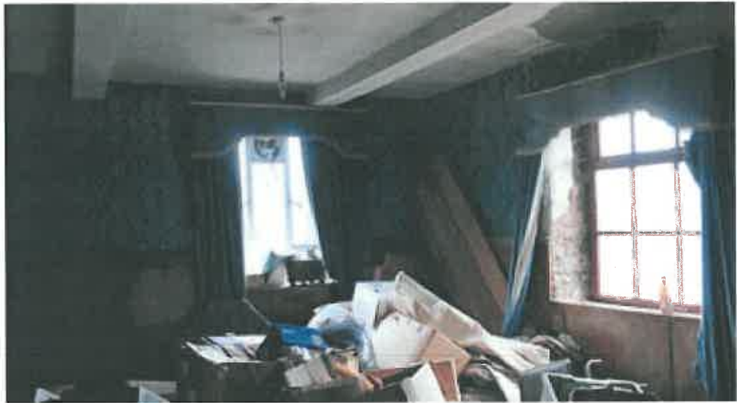
Plate 33: Manager's office above former boiler house
