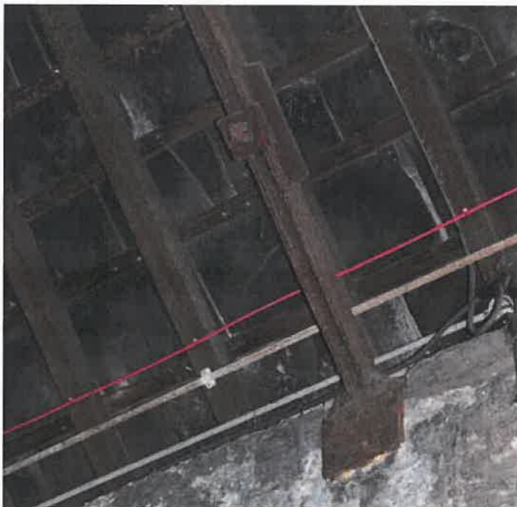
Plate 88: Detail of metal roof truss within boiler house
