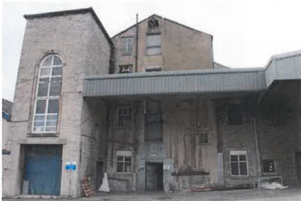
Plate 47: New Mill stair tower and engine house, with infilling to either side of stair tower
