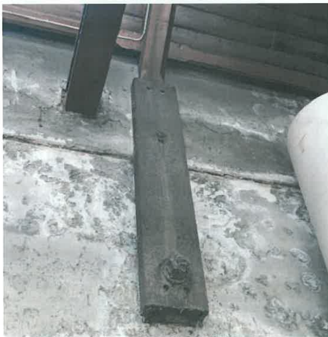
Plate 90: Wall bracing to trusses in south wall of engine house
