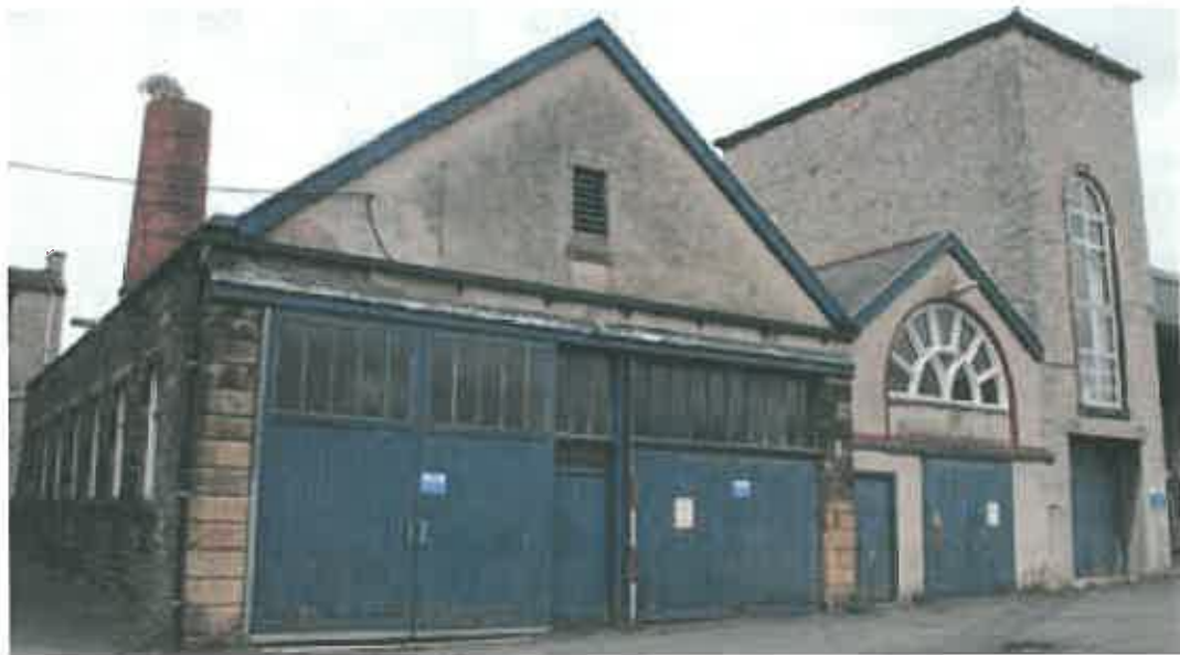
Plate 77: New Mill power plant, comprising boiler house, two engine houses and chimney
