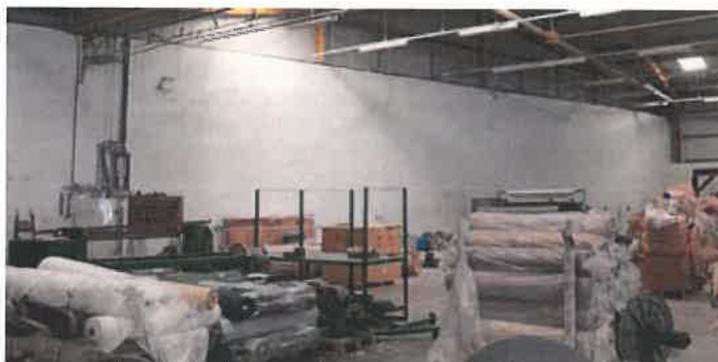
Plate 114: Roof scar for multi-span, saw-toothed roof of weaving shed
