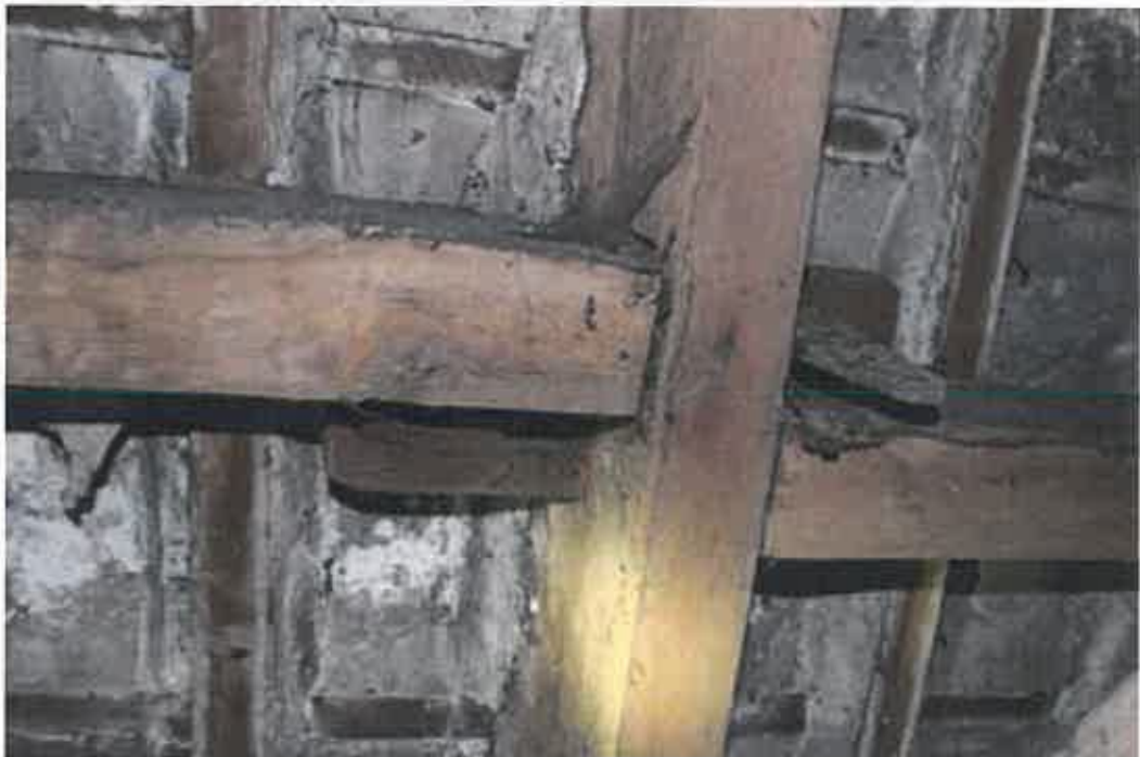
Plate 40: Tusk-tenoned purlins in original mill roof
