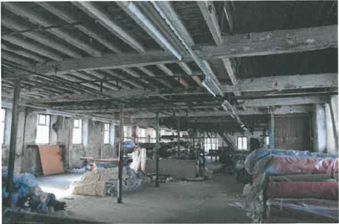
Plate 68: General view of second floor, New Mill, with internal hoist on right
