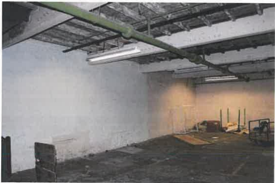
Plate 54: Blocked windows in north wall of New Mill following addition of weaving shed
