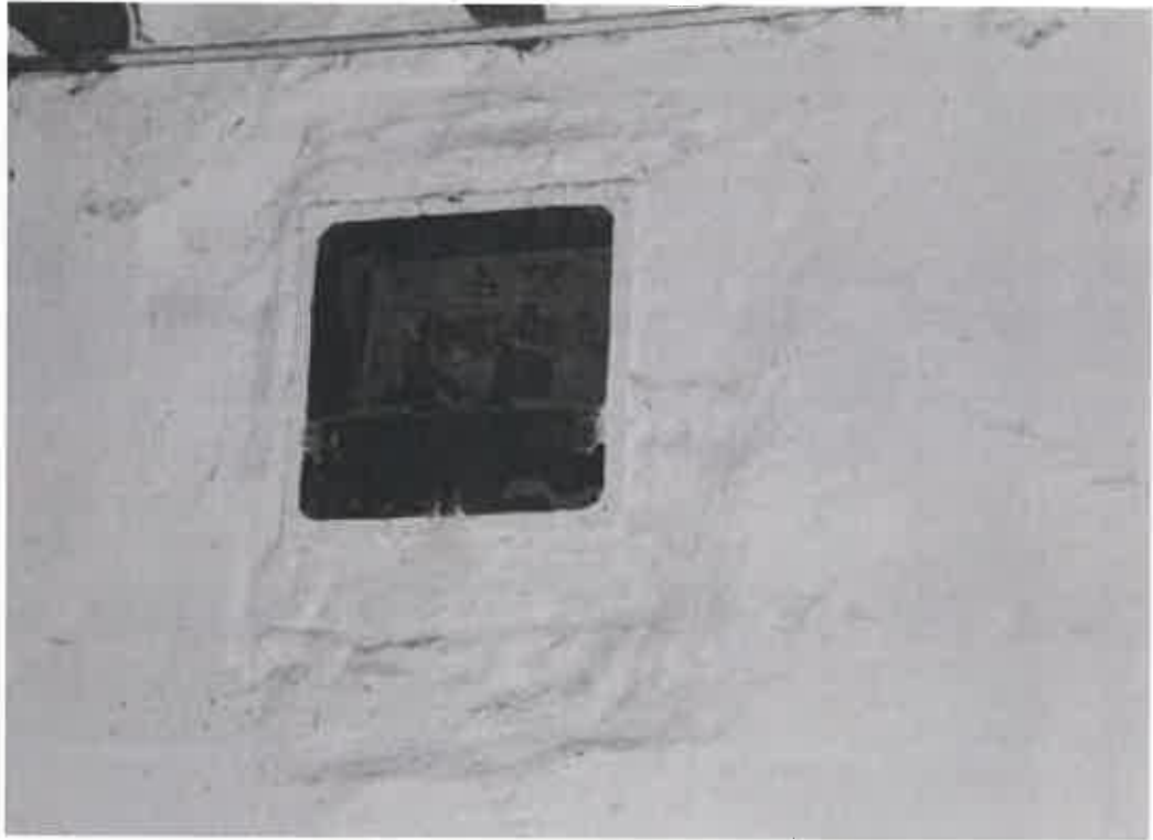
Plate 67: End bearing box, first floor, New Mill
