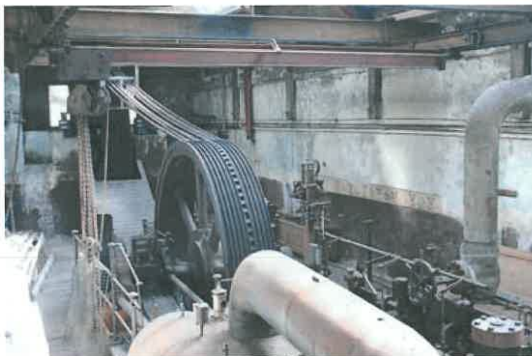
Plate 95: General view of engine house looking south-east
