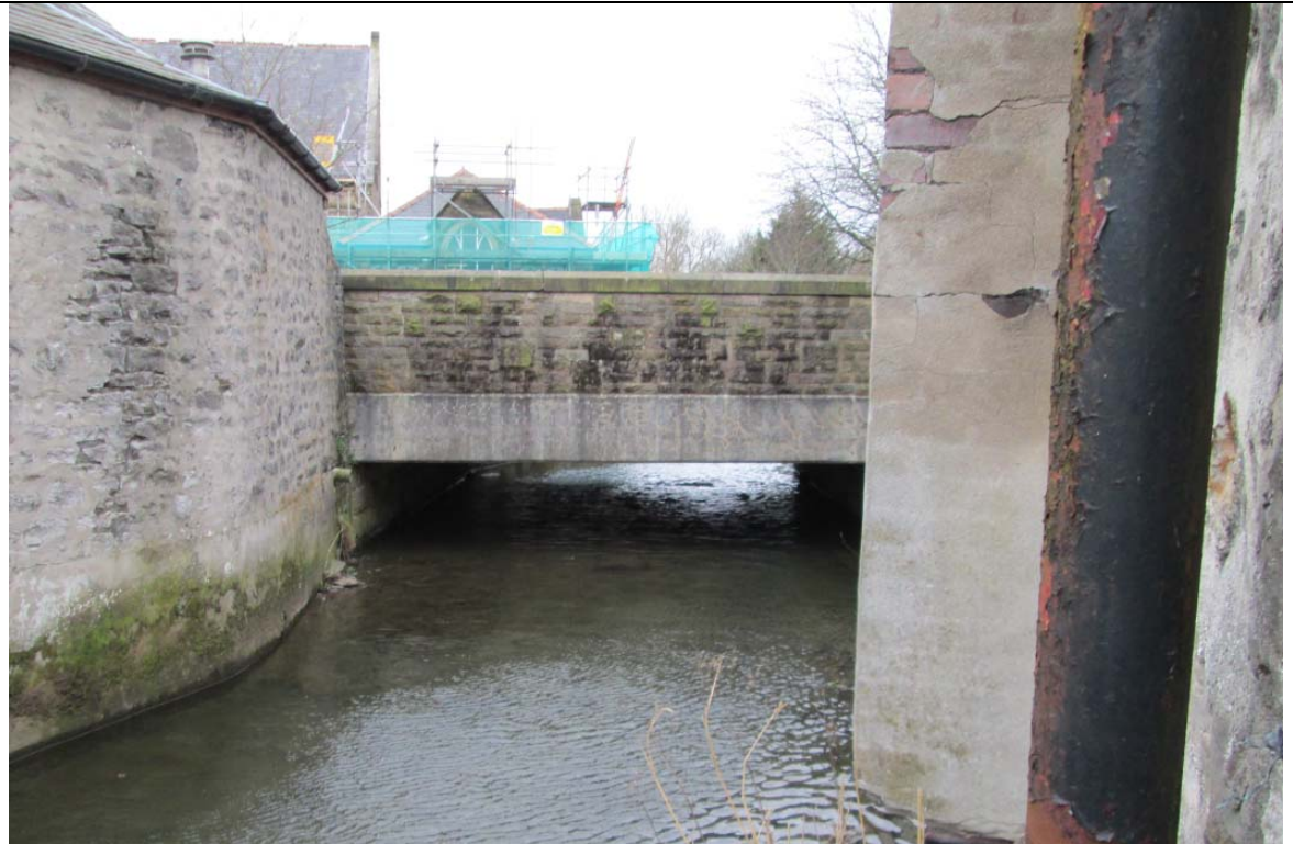
Figure 5.3: Greenacre Street Bridge (Looking downstream from the development site)
