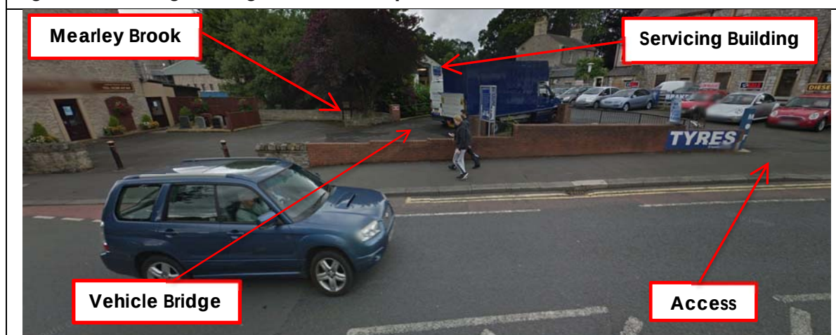
Figure 3.1: Existing Buildings Within Development Site
