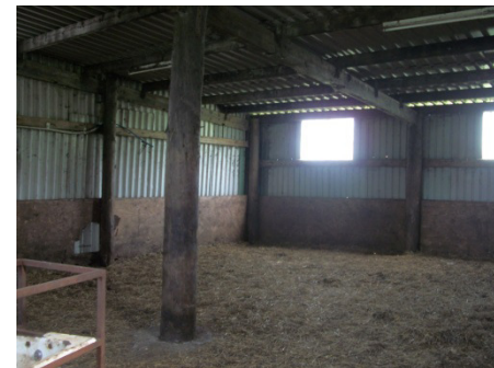
Figure 10: view inside Barn B
