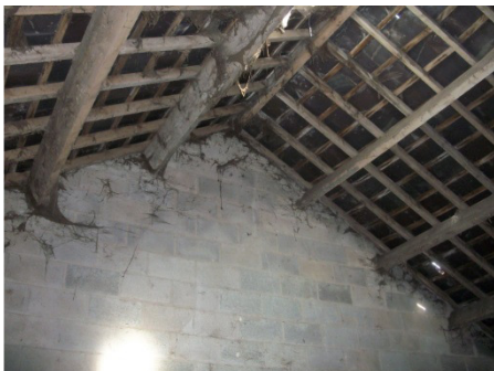
Figure 9: Barn A - roof detail
