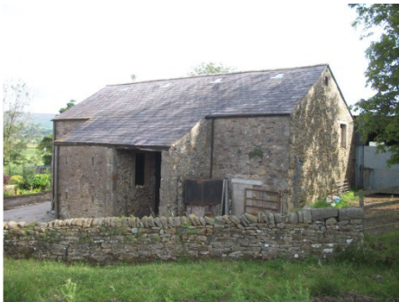
Figure 6: Stone barn - building A
