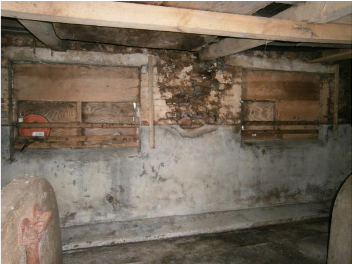
Photo 25 – North east elevation – internal in lower section
