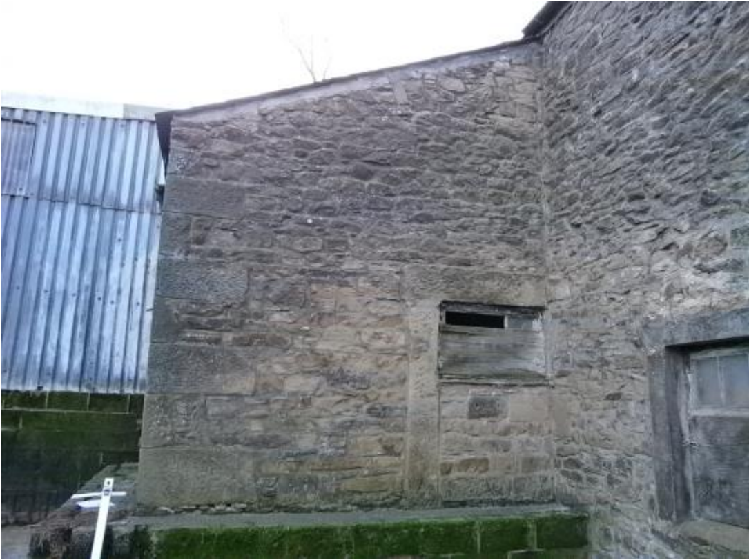
Photo 5 – North East Elevation – Damage at corner with gable
