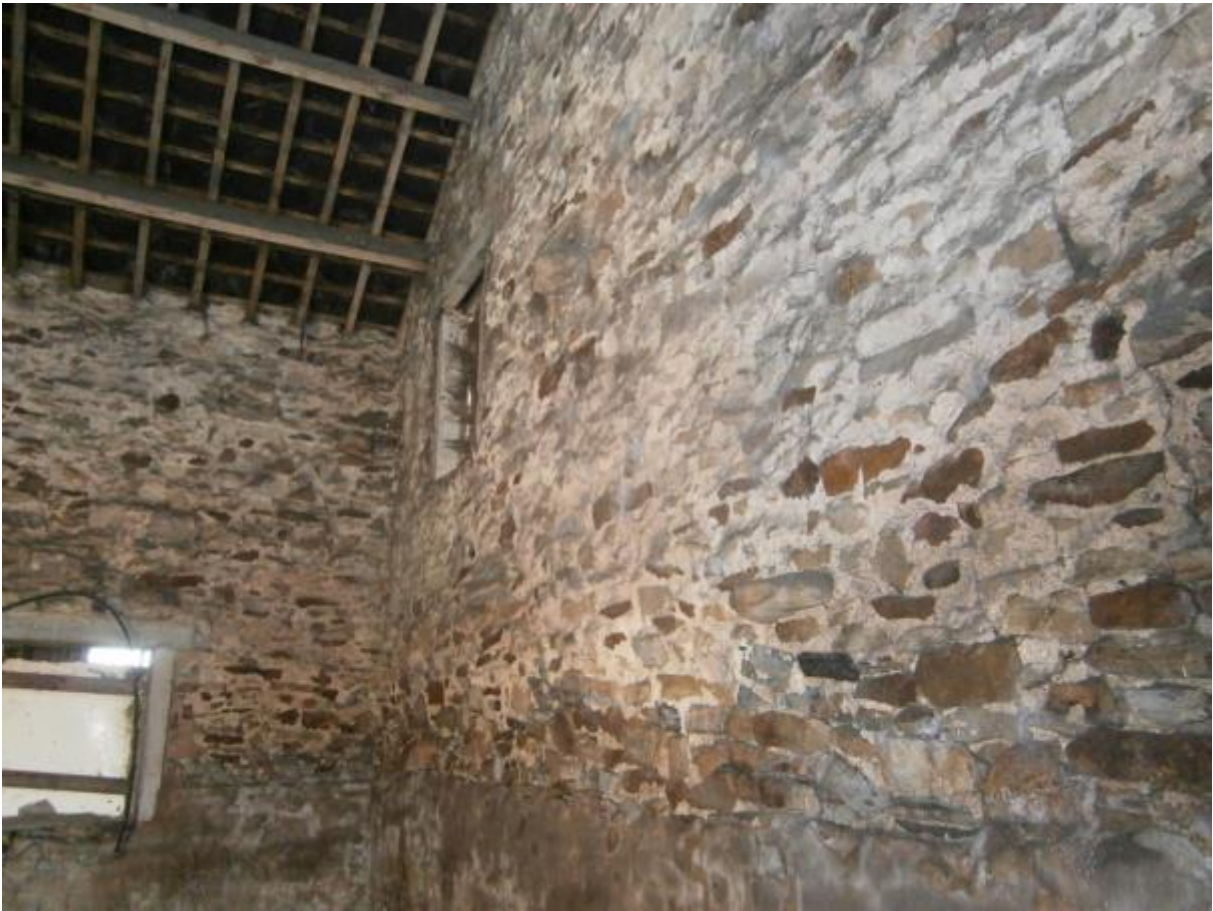
Photo 32 – Internal of South East gable
