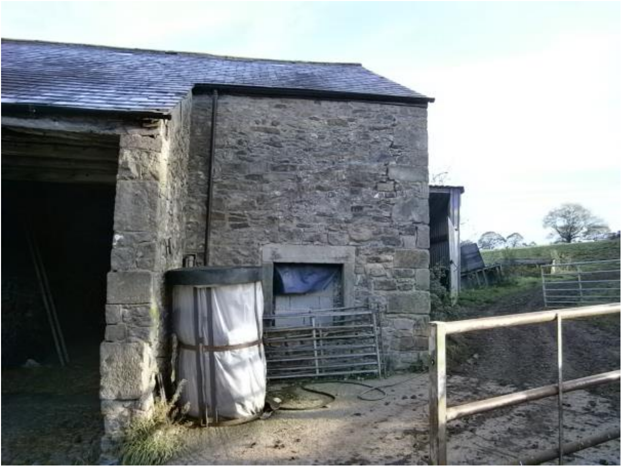
Photo 16 - South West Elevation – upper section
