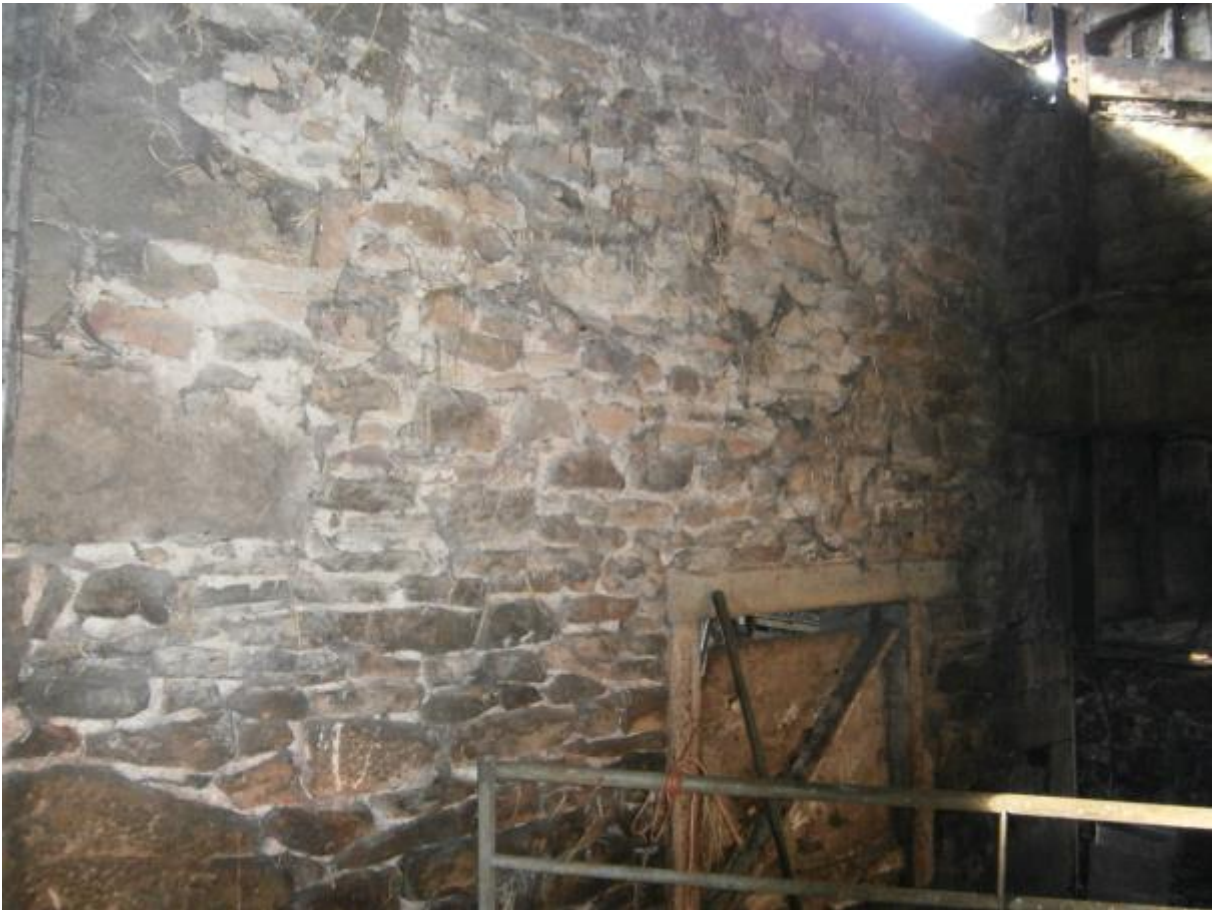
Photo 23 – North East Elevation – upper section (inside lean-to)
