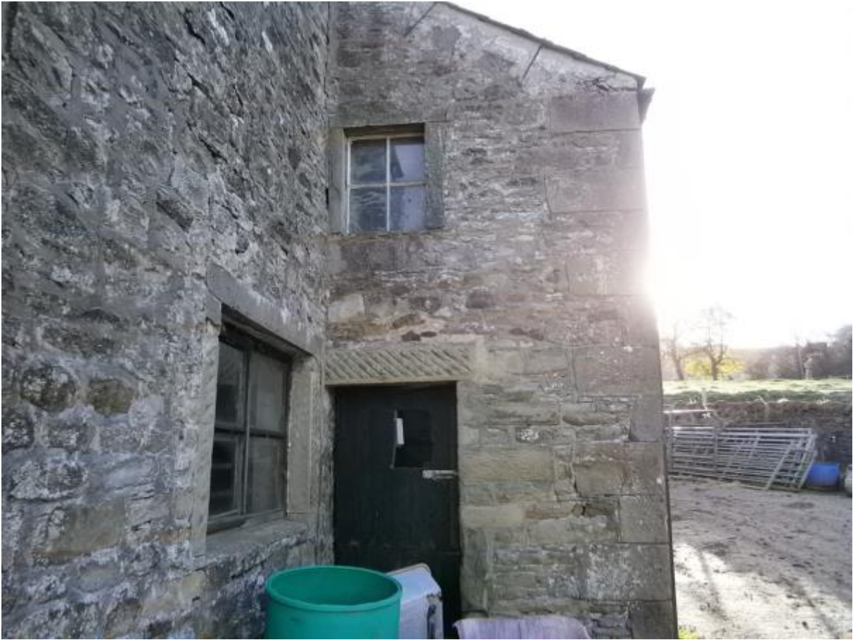
Photo 12 – South West Elevation - outrigger
