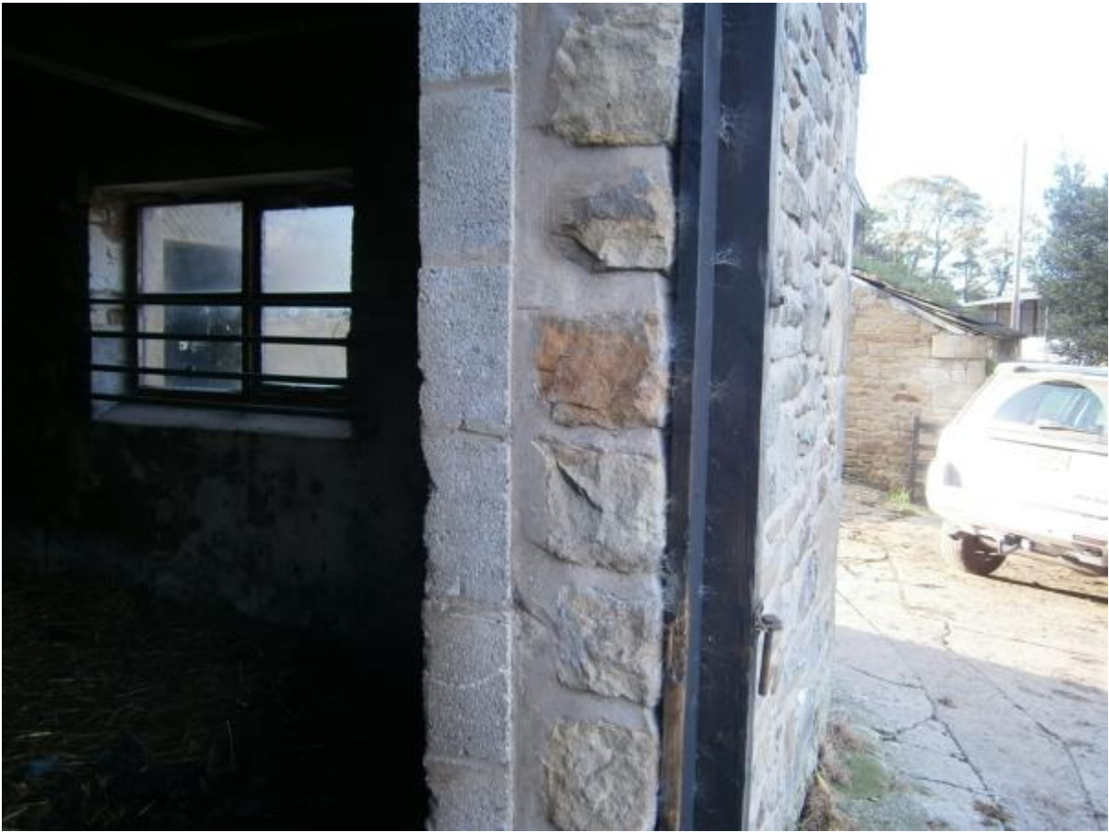
Photo 3- North West Elevation – Re-built wall detail
