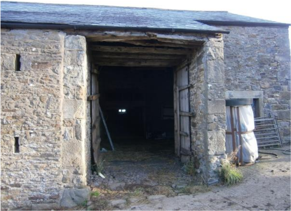
Photo 14 - South West Elevation – mid section
