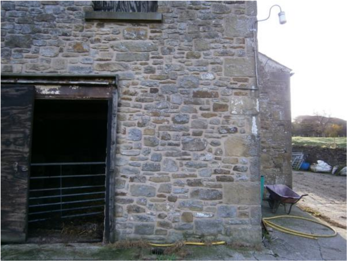
Photo 2 – North West Elevation
