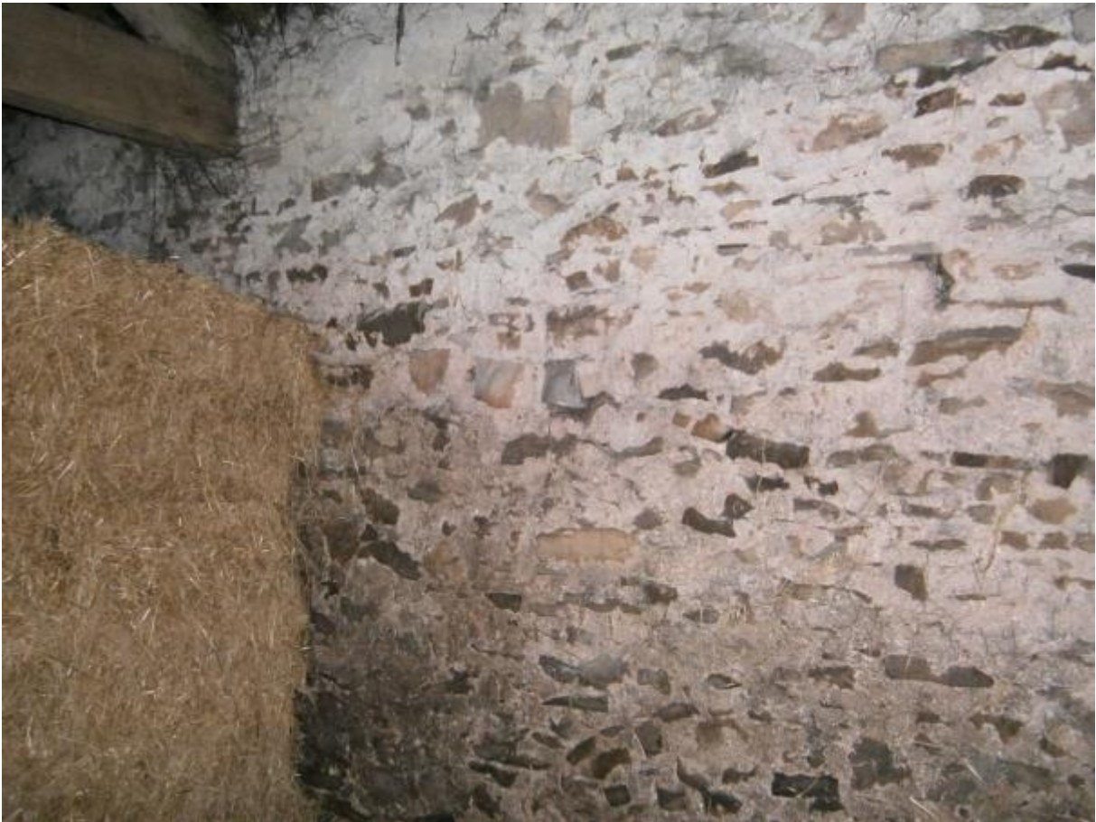
Photo 31 – Upper section of North East internal
