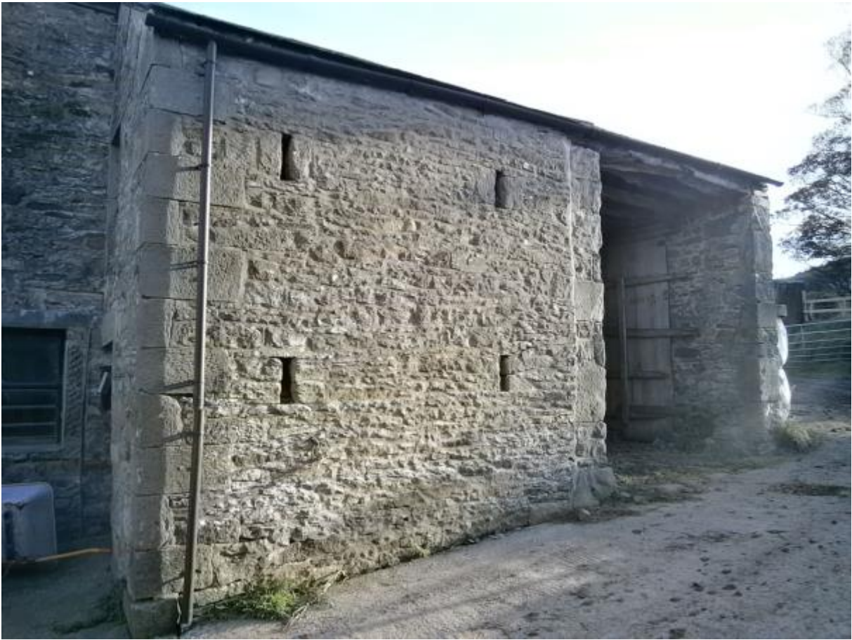
Photo 13 – South West Elevation – mid section
