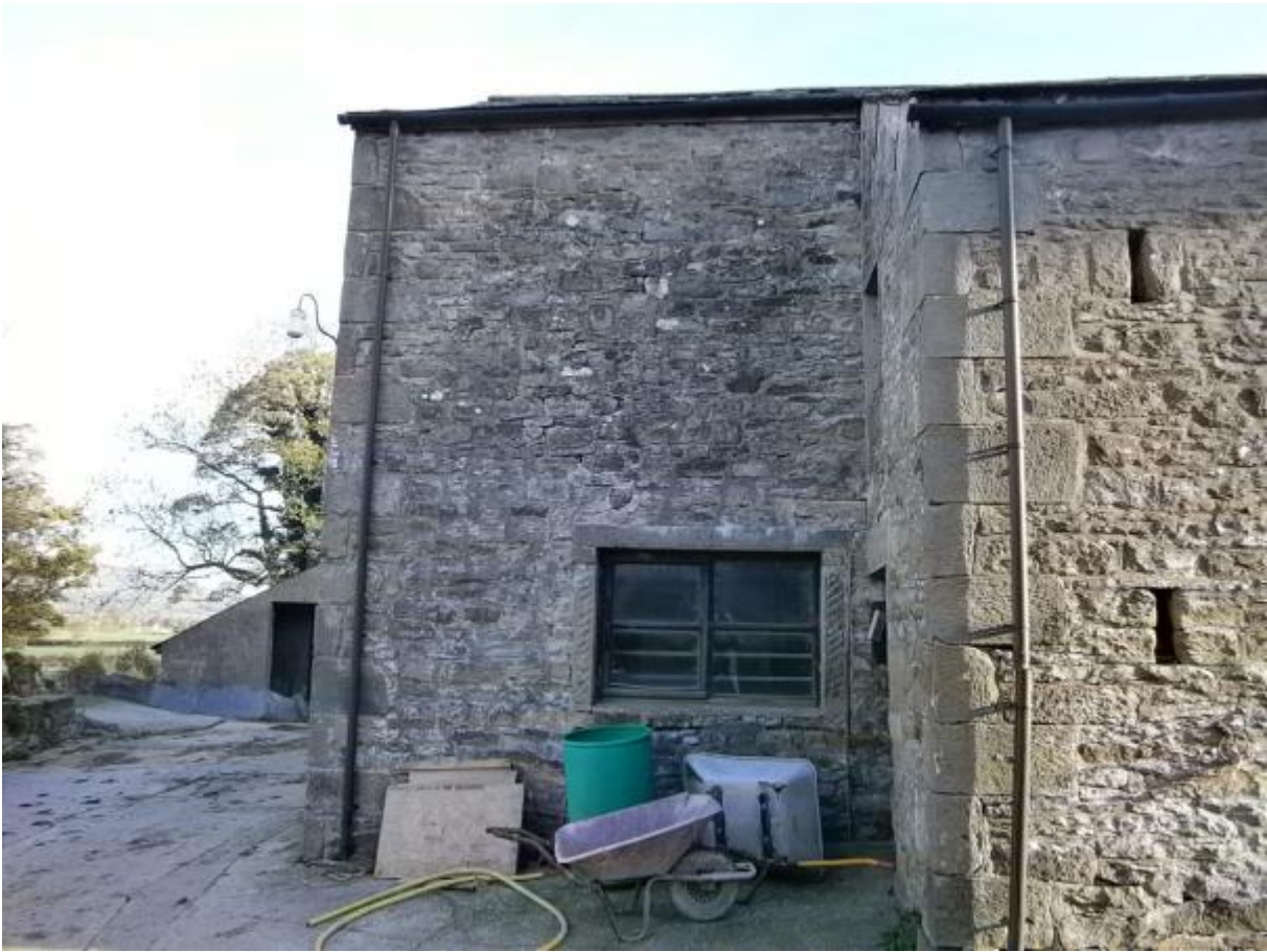
Photo 9 – South West Elevation – lower section
