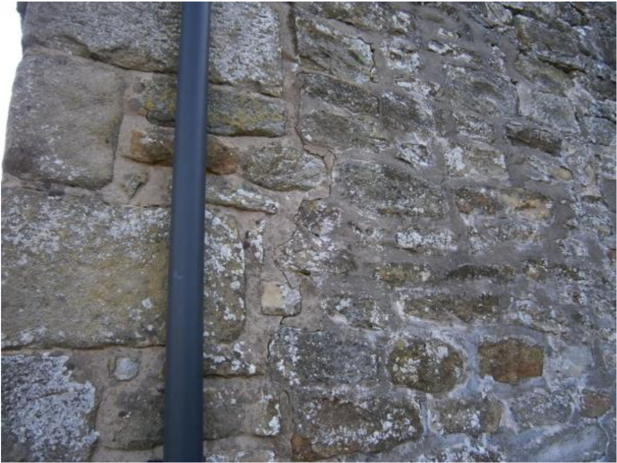
Photo 11 – South West Elevation – joint to re-built gable
