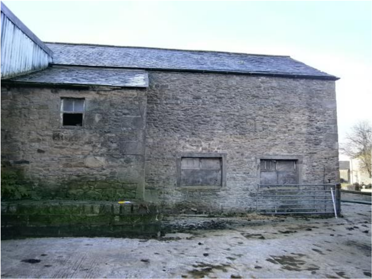
Photo 4 – North East Elevation
