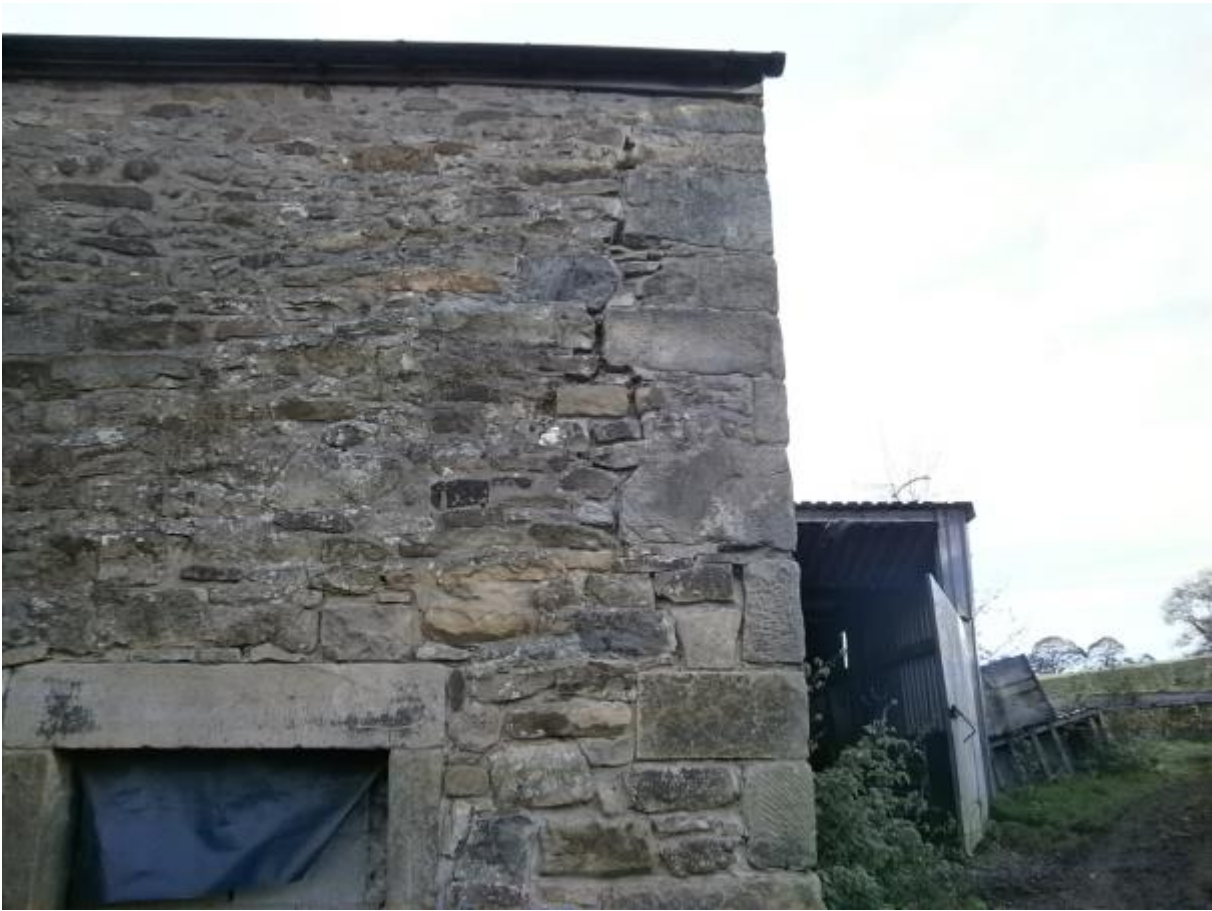
Photo 17 - South West Elevation – upper section
