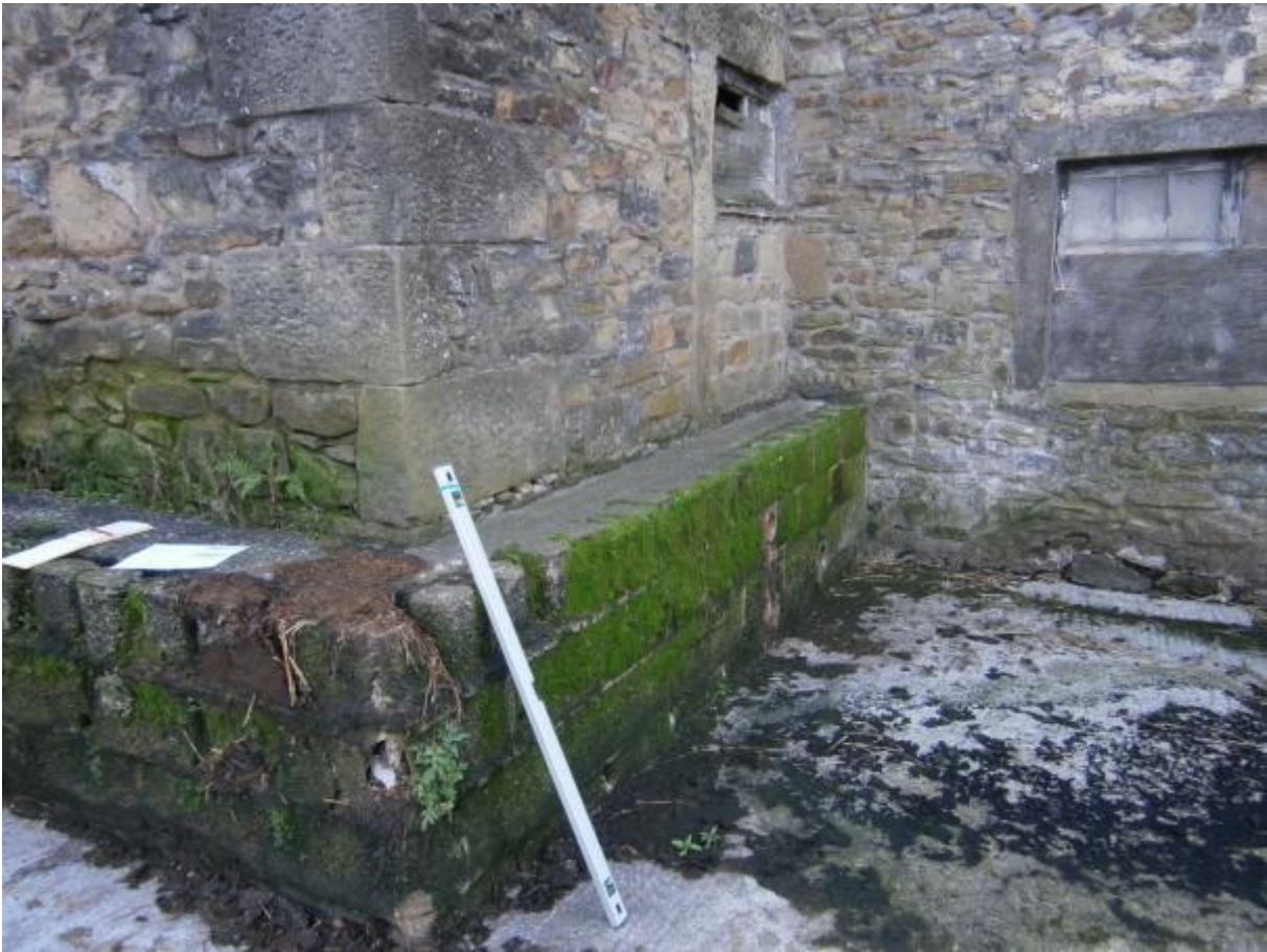
Photo 8 – Outrigger to North East Elevation – block/concrete cladding
