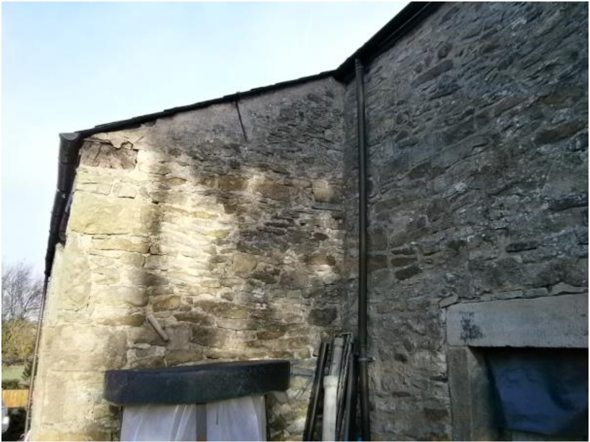
Photo 19 - South West Elevation – outrigger
