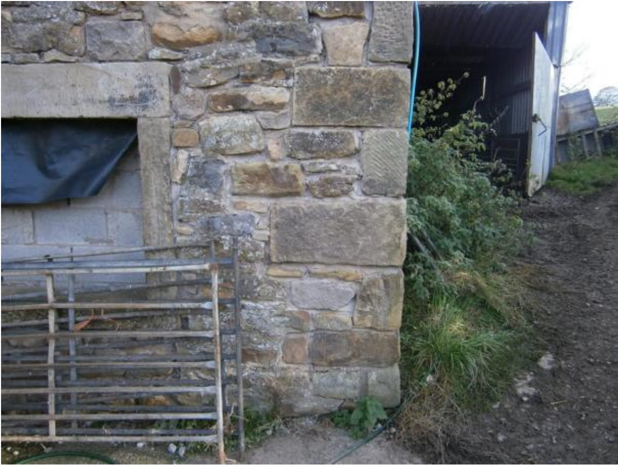
Photo 18 - South West Elevation – upper section – re-built corner
