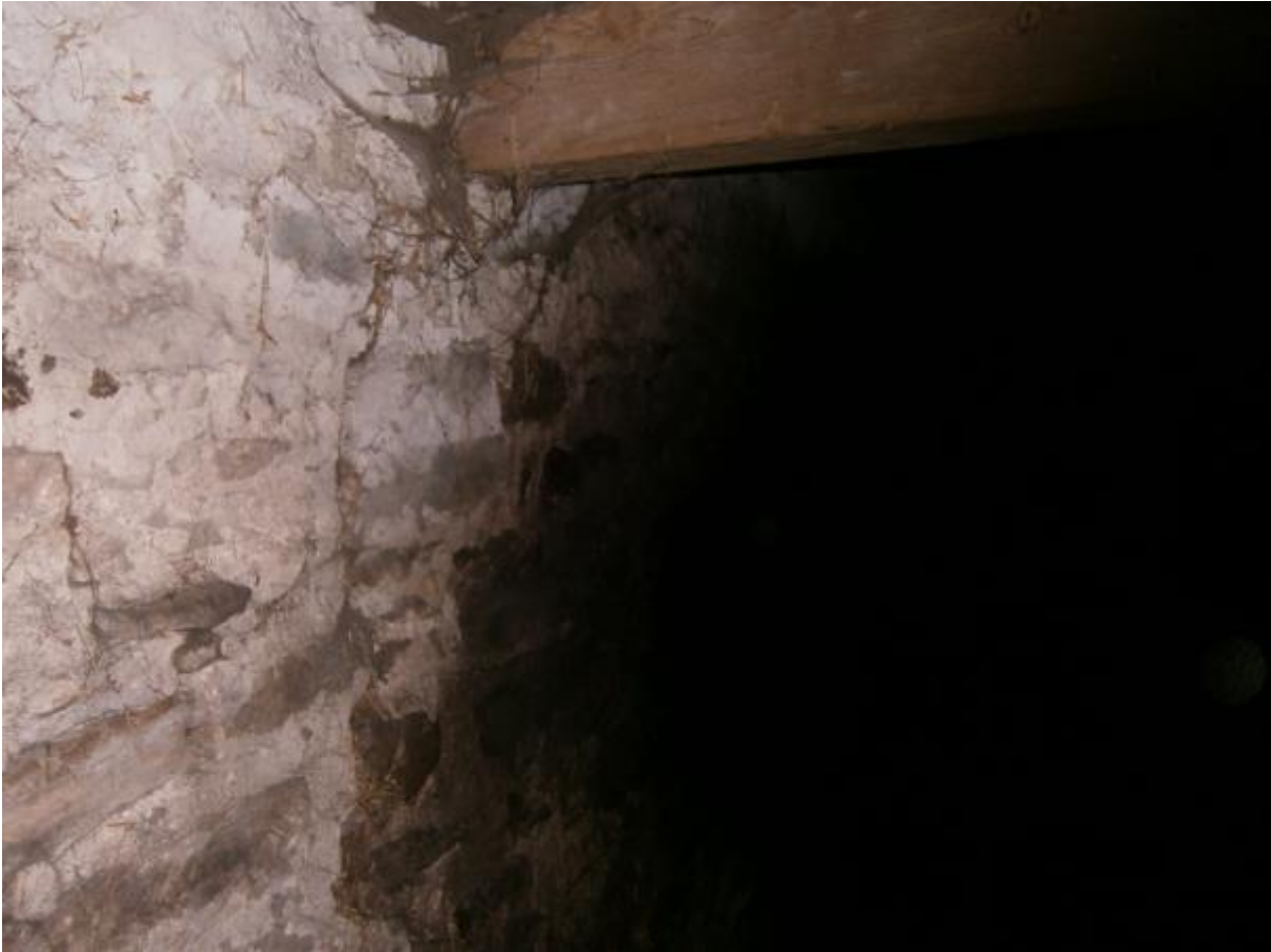
Photo 29 – Truss sat on walls – no cracking or movement
