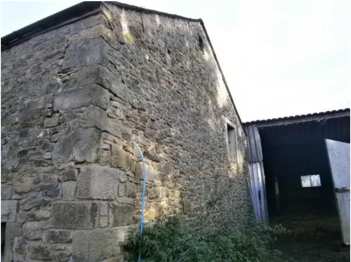
Photo 20 – South East Elevation
