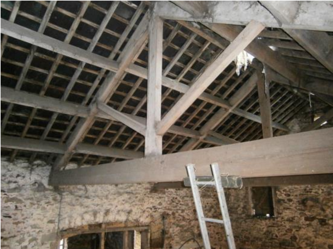
Photo 30 – Truss and purlins – North East and south east walls
