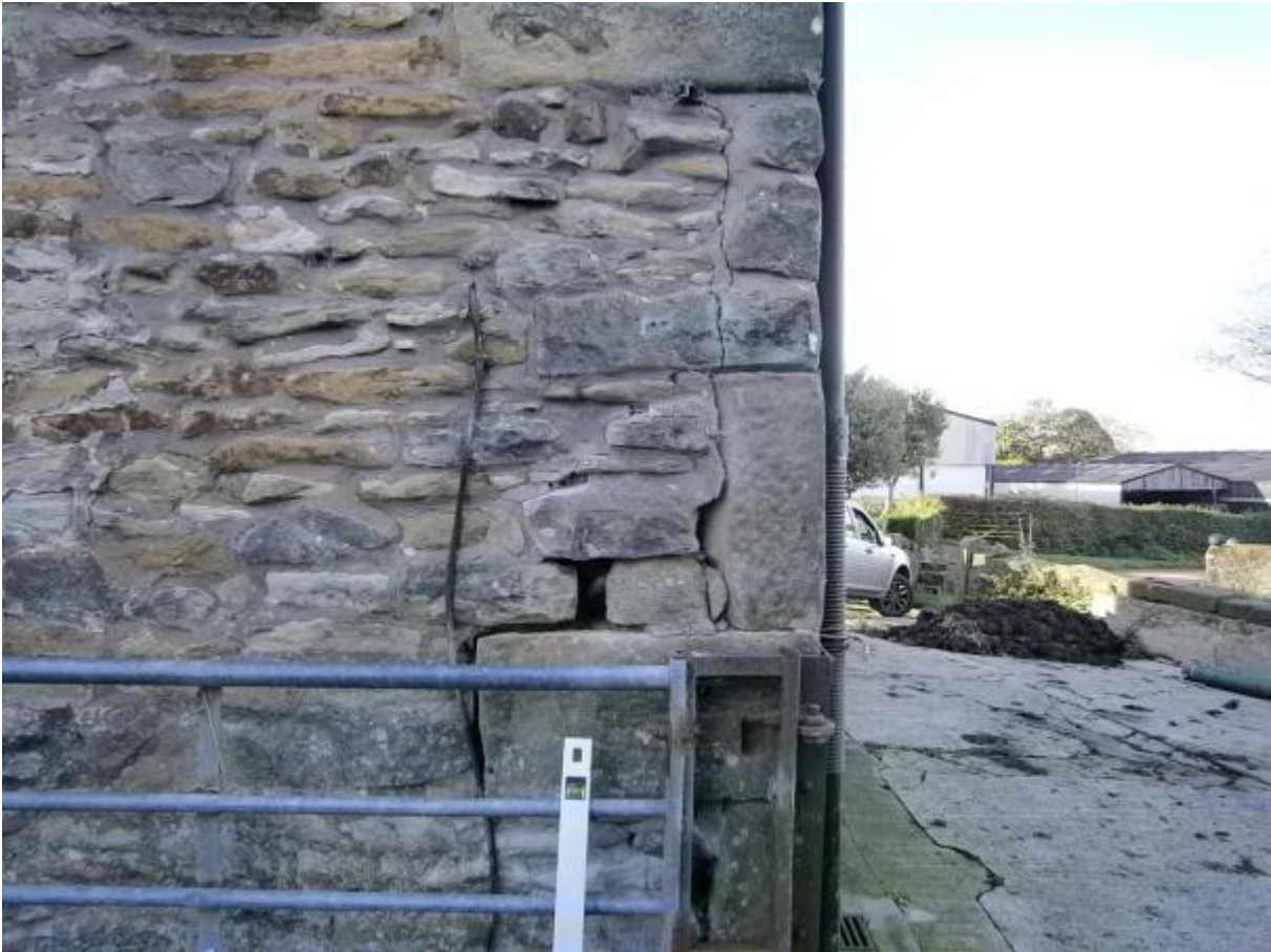
Photo 5 – North East Elevation – Damage at corner with gable
