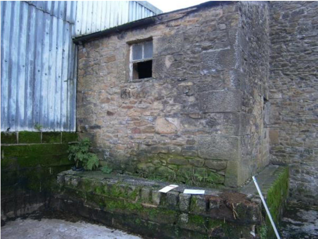
Photo 7 – Outrigger to North East Elevation
