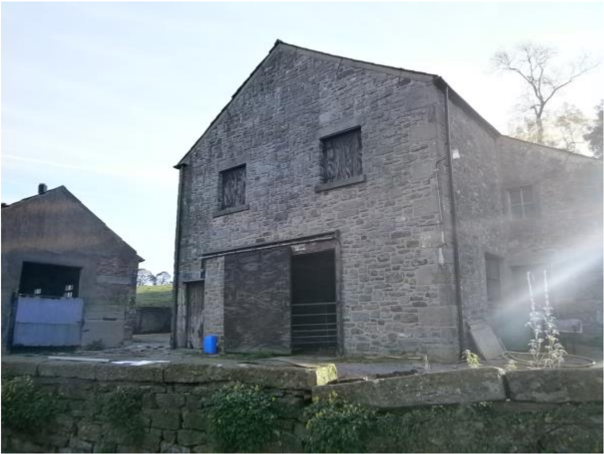
Photo 1 - North West Elevation
