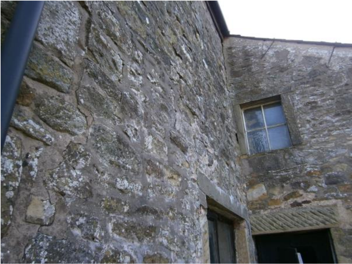
Photo 10 – South West Elevation – lower section – bow over window
