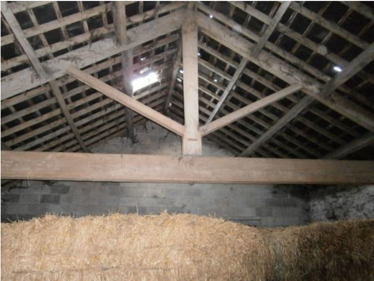
Photo 27 – Roof structure and North West Gable
