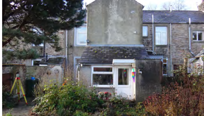
View of Carlton Cottage, from back garden, showing original 2-storey outrigger and single storey lean-to section.
