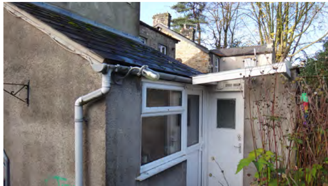
View of existing lean-to Section towards back door and external WC.
