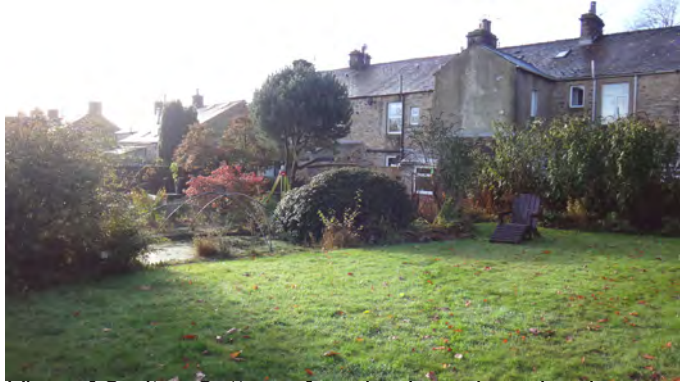
View of Carlton Cottage, from back garden, showing original 2-storey outrigger and adjacent single storey lean-to extensions.
