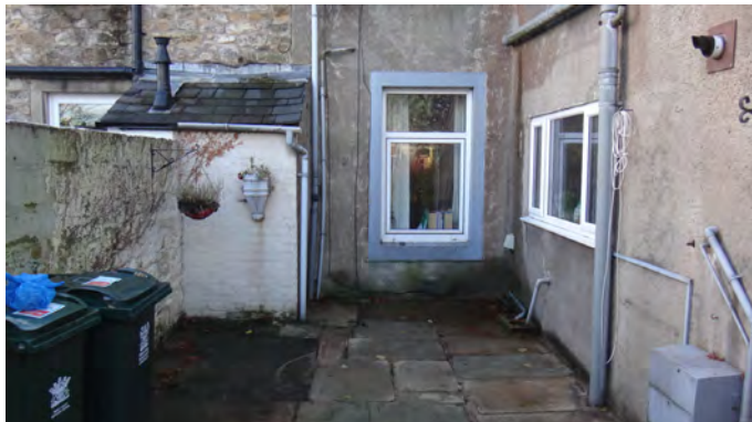
View of yard area, towards rear Living Room window.
