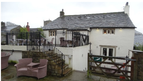
Figure 3: rear elevation showing paved veranda
