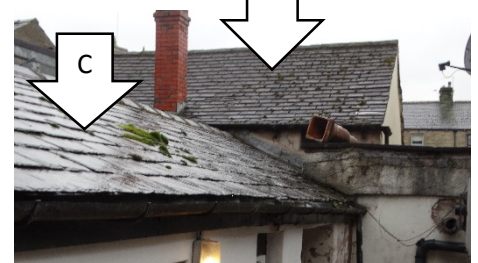
Figure 5: kitchen roof 'C' and dining area roof 'A'
