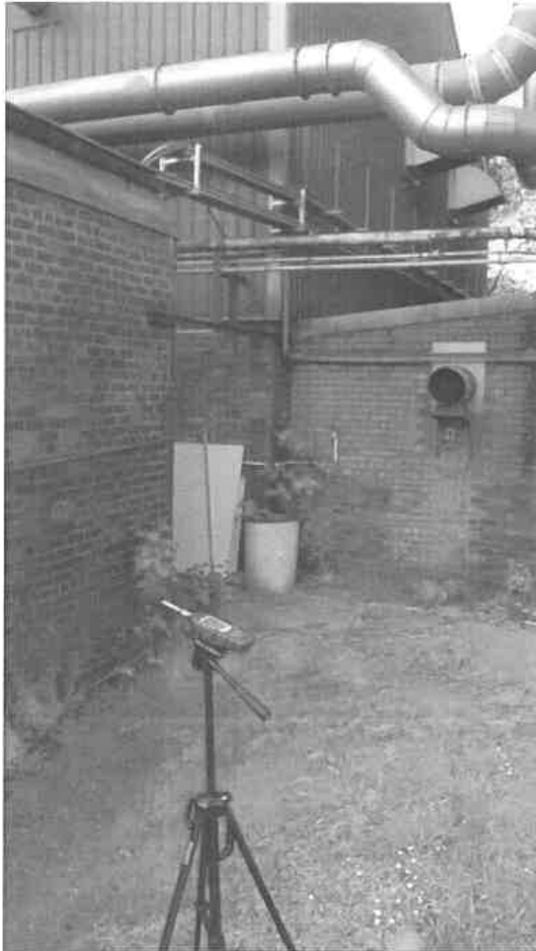
External Monitoring Location No1 By the corner of the building and adjacent to the newer metal clad building
