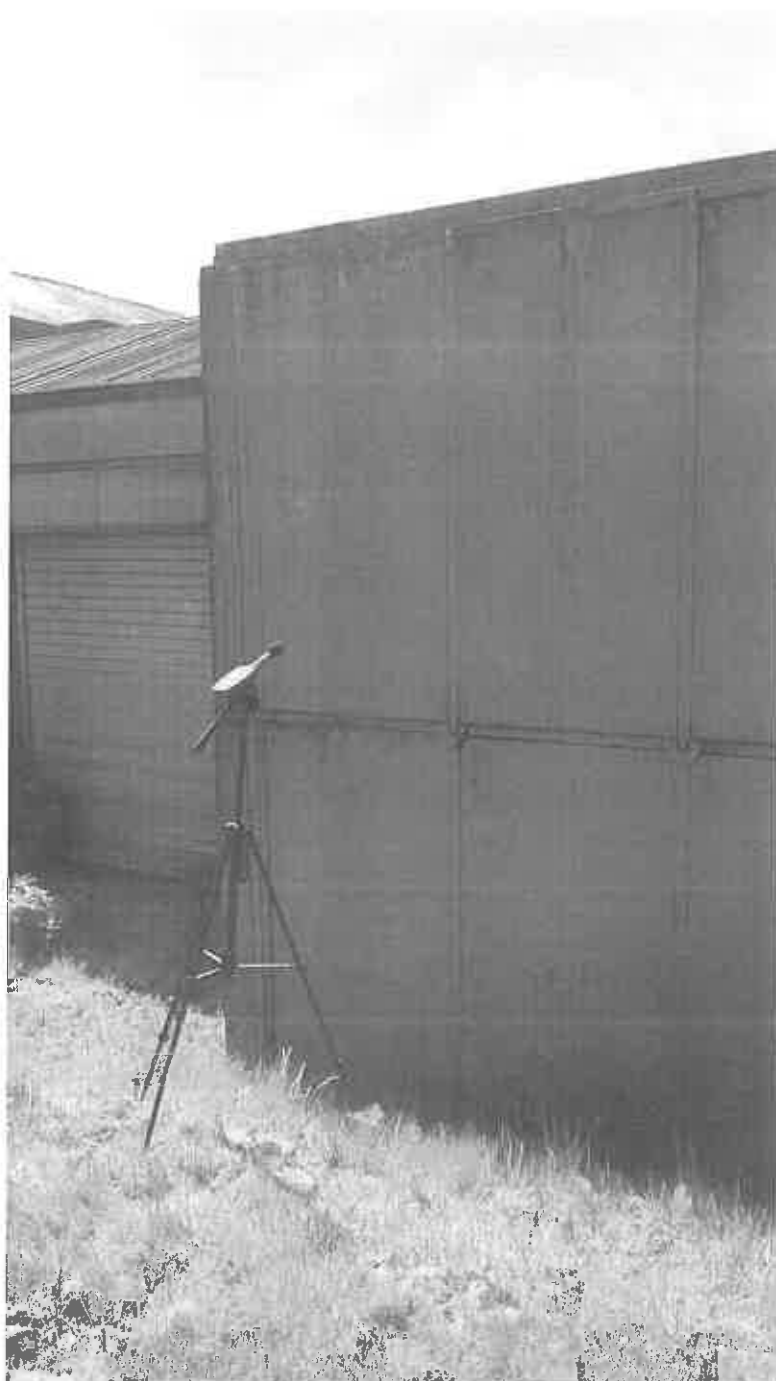
External Monitoring Location No3 By enclosed extraction filter unit
