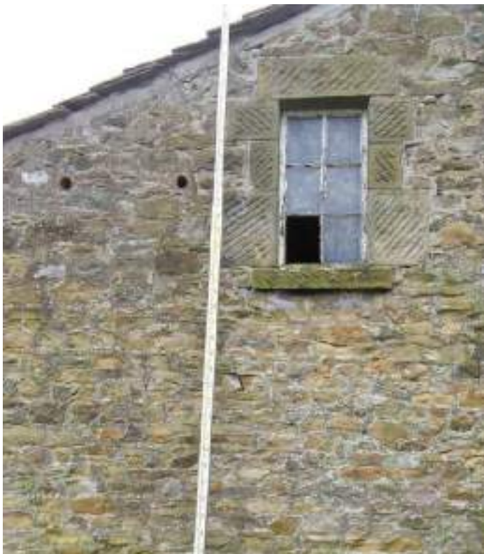
18 Detail of first floor window opening.
