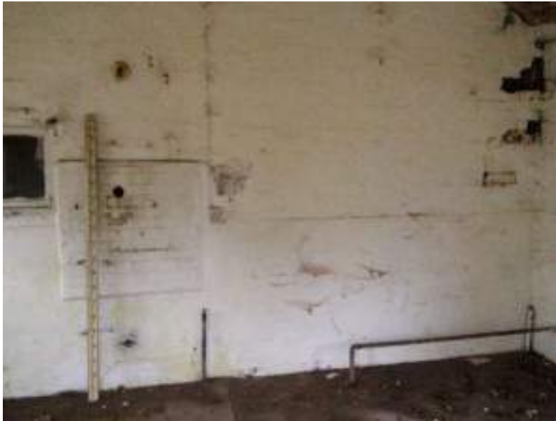
Figure 14 Internal view of the brick dairy
