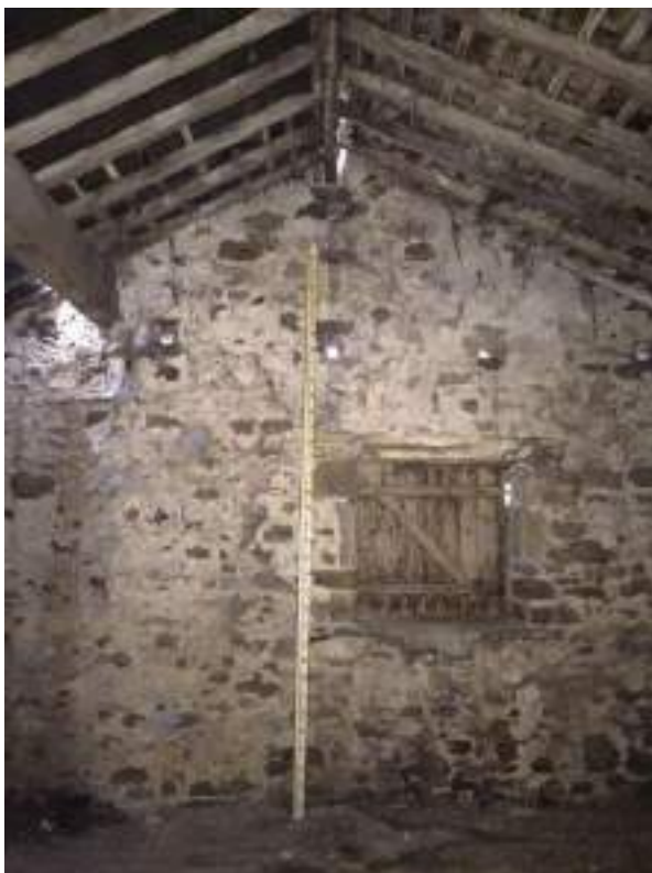
Figure 17 Internal view of the first-floor hayloft
