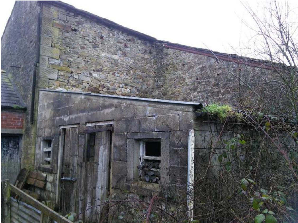
23 Rear (south west) corner showing lean to building (no access possible)
