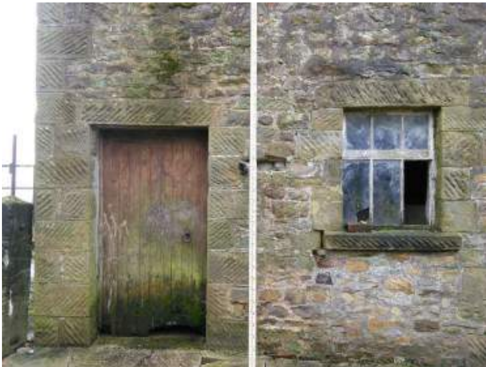
12 Door and window detail, note quoins to corner of the barn
