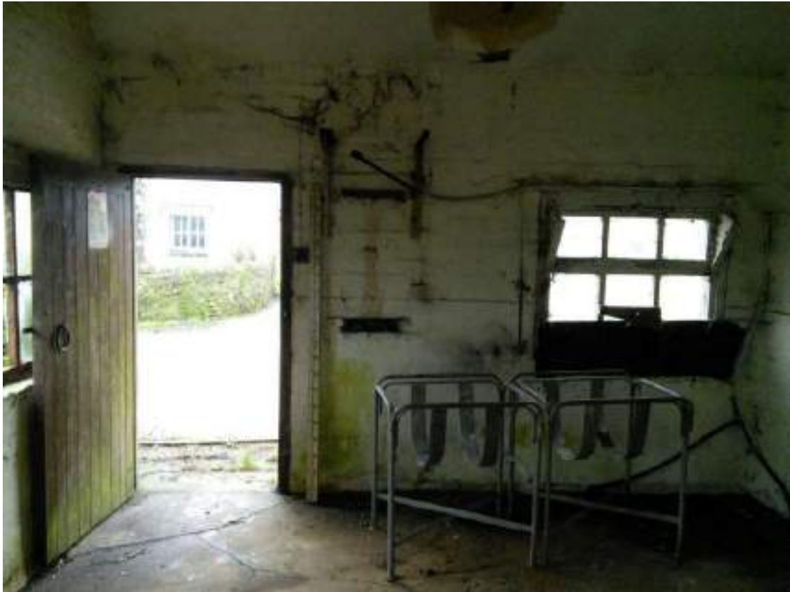
31 Internal view showing access door and window; Front wall.
