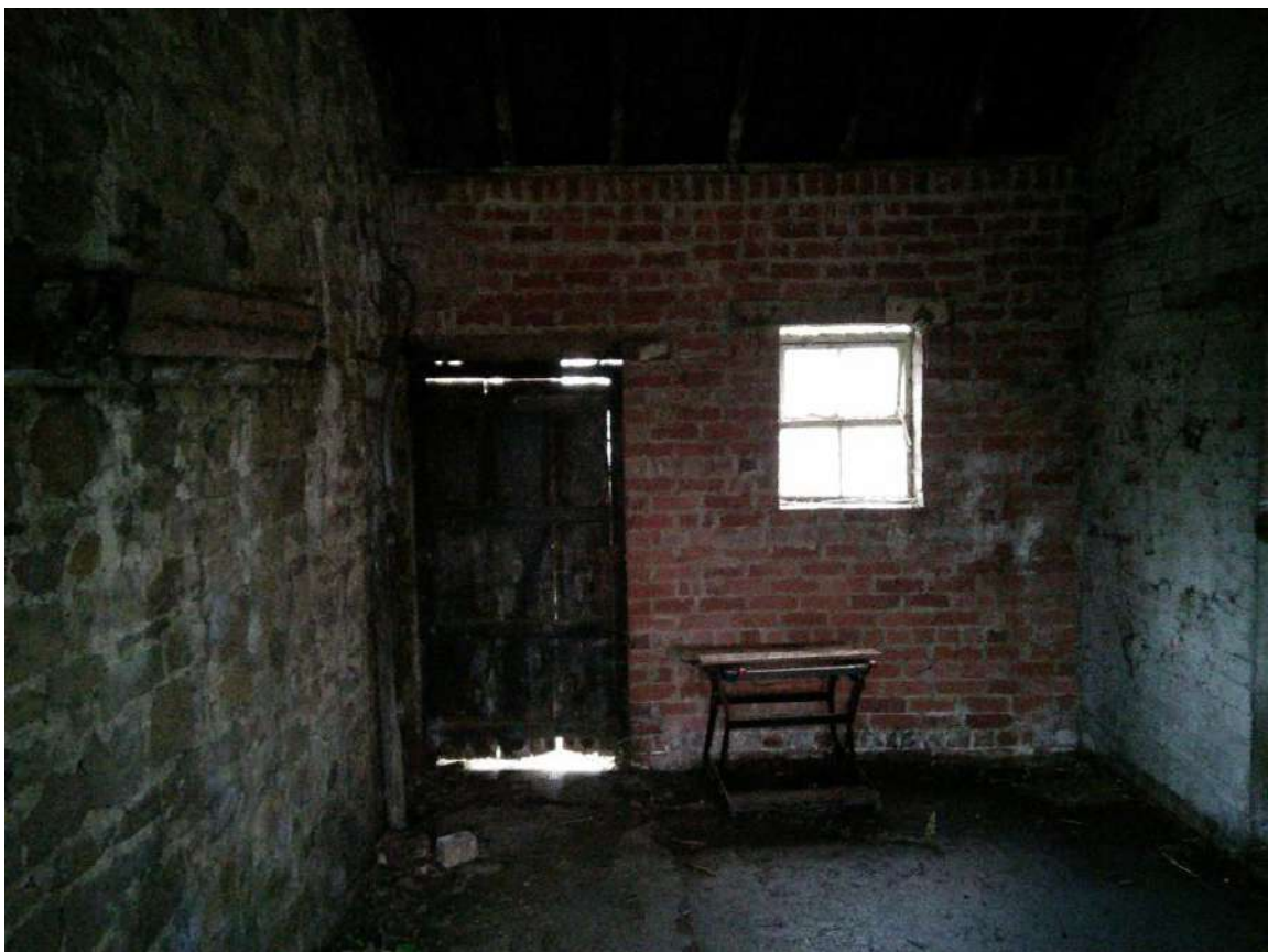
38 Rear wall to store showing timber door and window detail.
