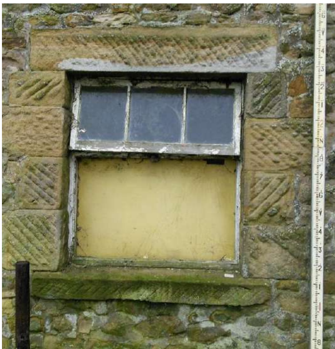
16 Window detail showing fenestration and stone quoins, head and cill.
