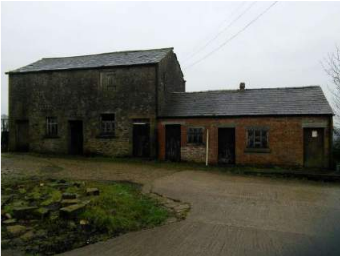
1 Front (north east) elevation showing the single storey dairy and original two storey barn
