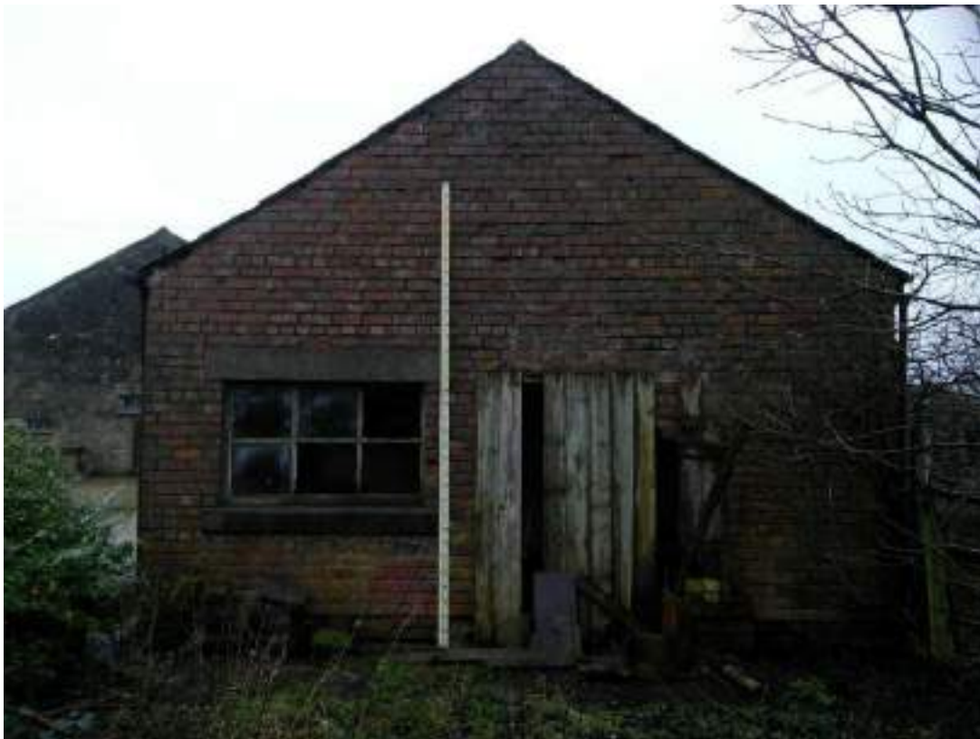
28 South west elevation showing gable to single storey dairy.
