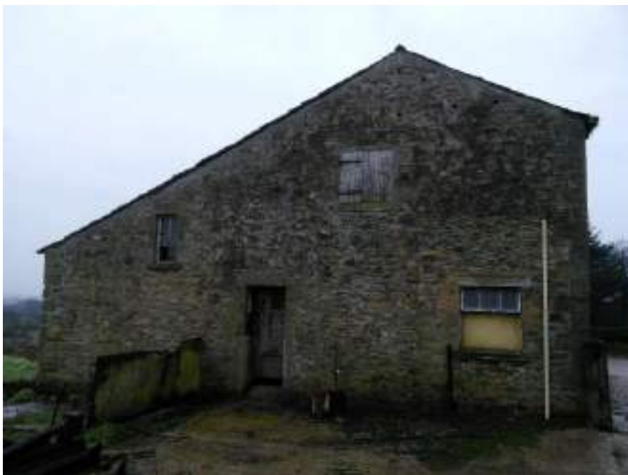
Figure 9 The north-east elevation of Barn One showing the access door.
