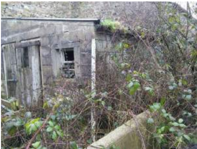
Figure 19 View of single storey lean to structure to rear of barn
