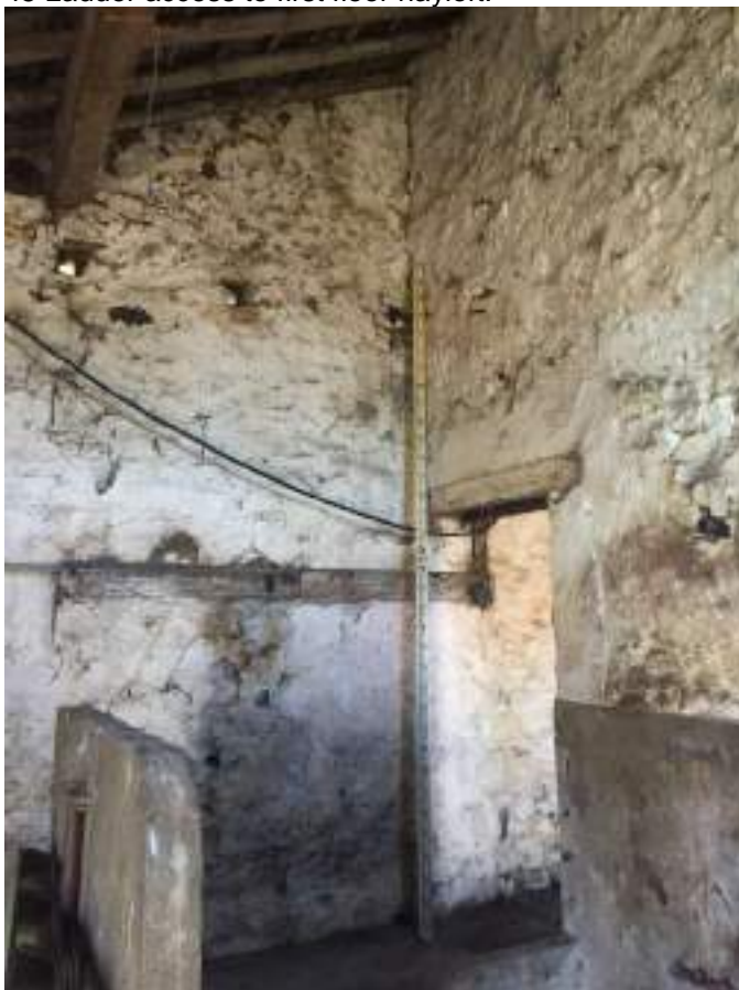
46 View of concrete cattle stalls and separating wall to rear shutout.
