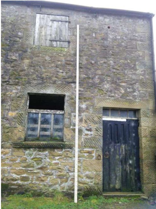
7 Detail of doorways and window, note quoins, heads & cills with boasted detail to surfaces
