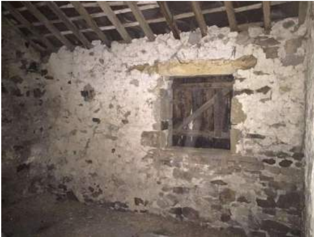
51 Access door to front elevation
