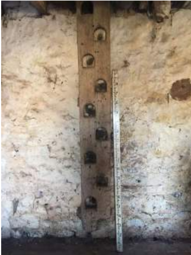
45 Ladder access to first floor hayloft.
