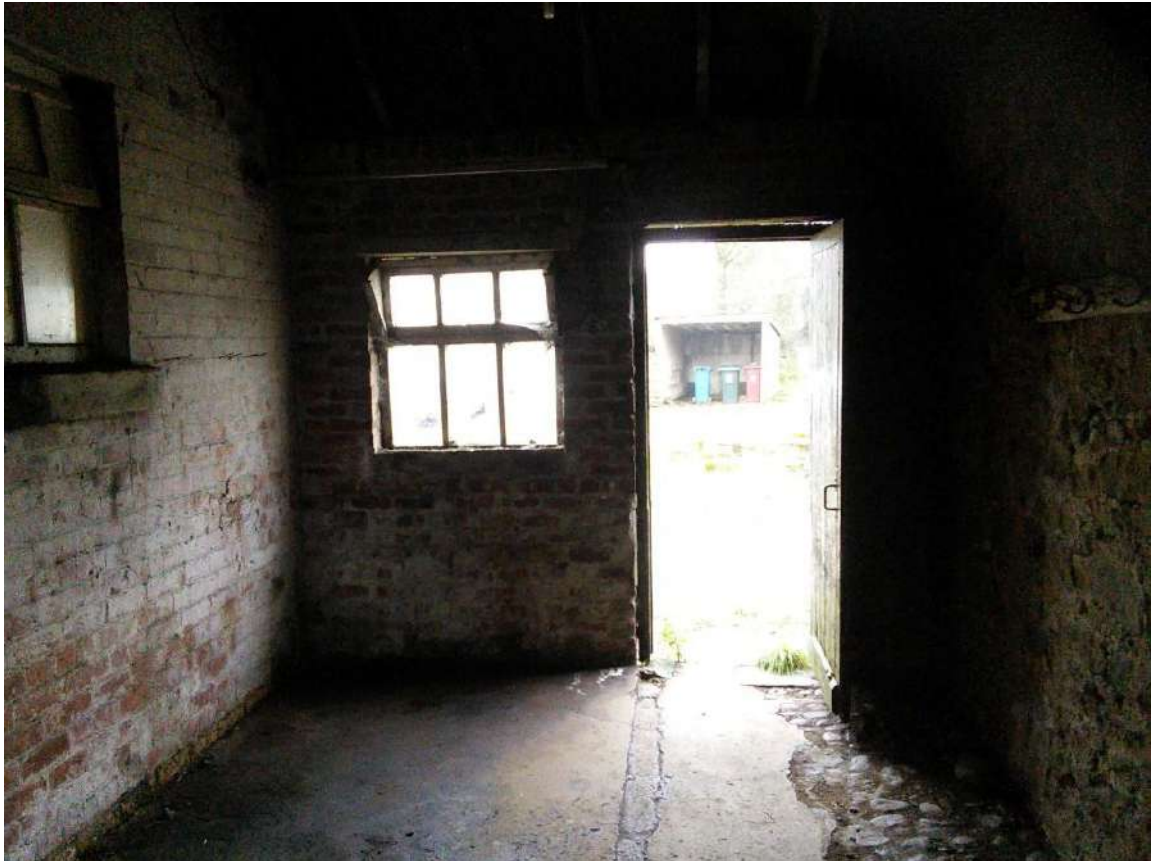
37 View of front wall to store, note change to floor finishes
