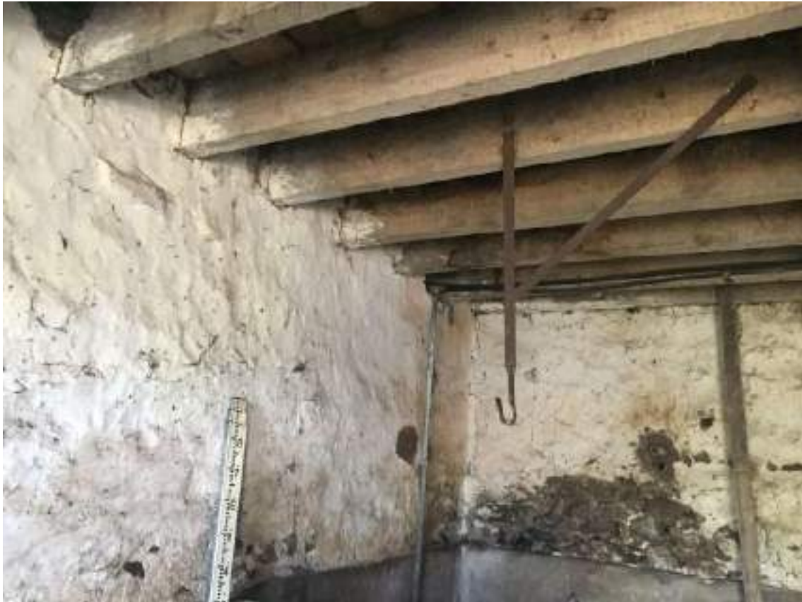
43 Steel hooks fixed to ceiling joists over cattle stalls.
