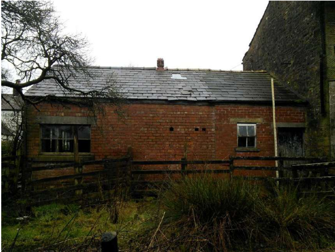
25 Rear view of dairy building showing ridge vent to roof
