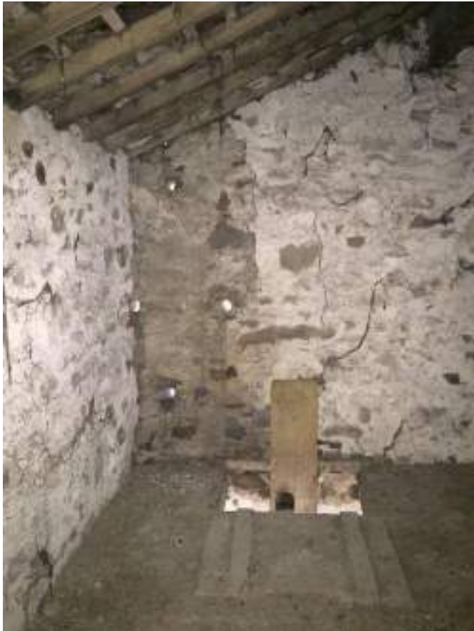
53 Access hatch and ladder. Note ventilation holes to wall
