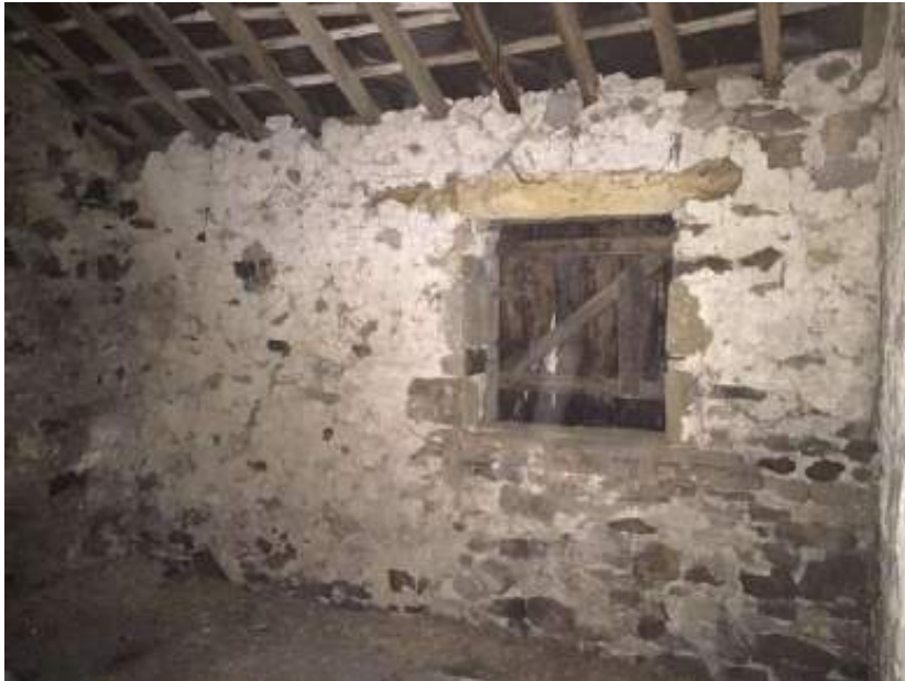
Figure 18 Internal view of the first-floor hayloft and access opening
