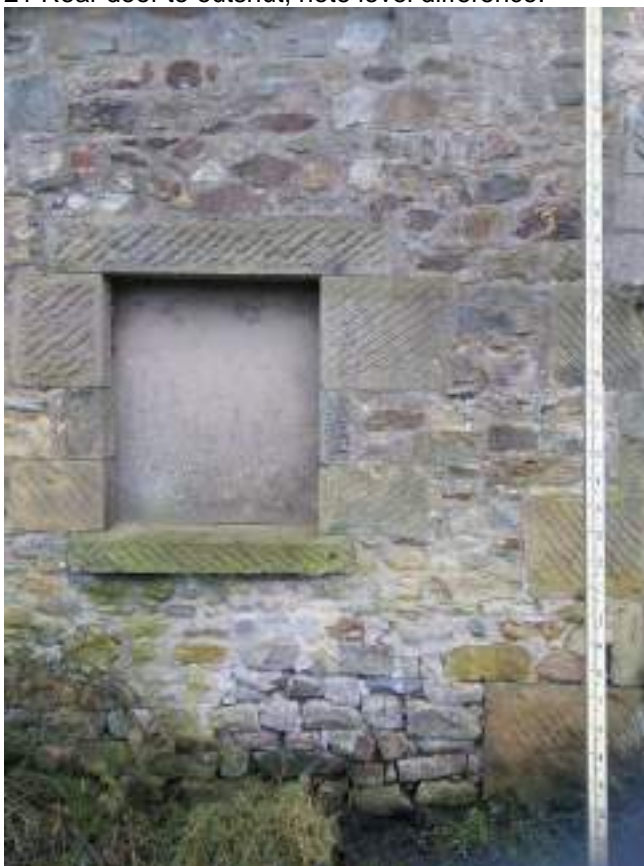
22 Rear elevation window detail.
