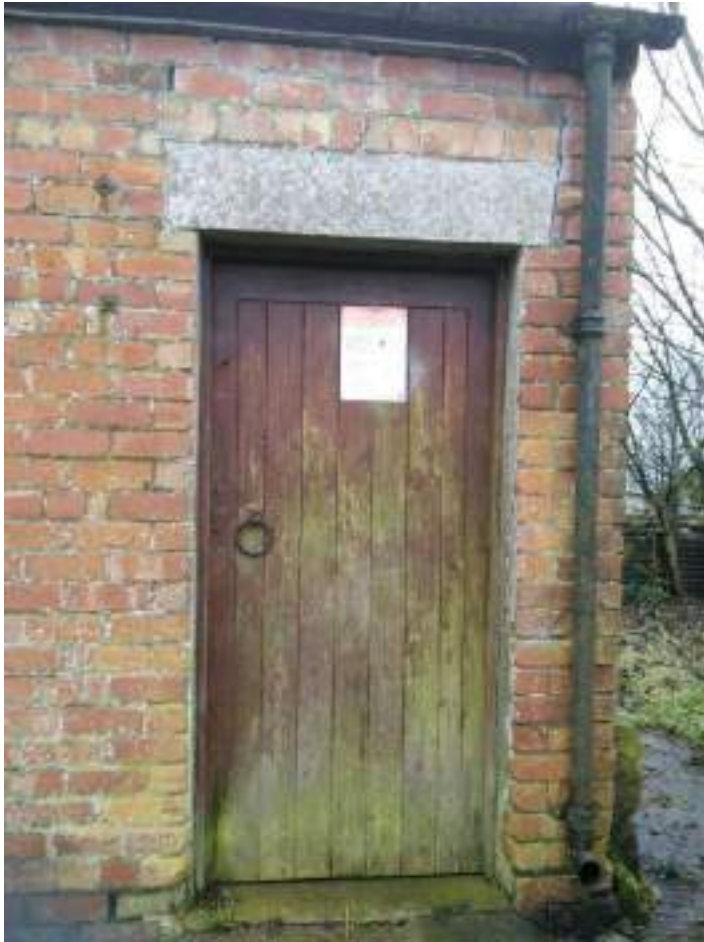
5 Modern timber door to dairy and cast iron rainwater goods.
