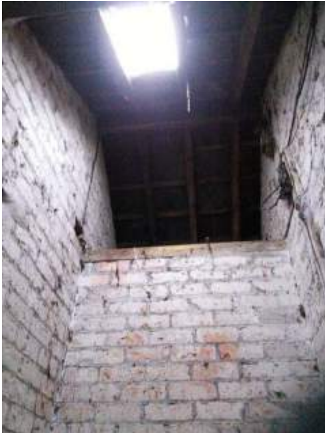
35 View above oil store showing roof construction
