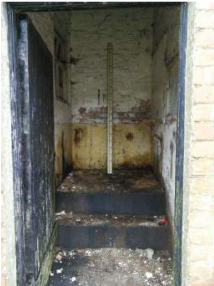
34 Oil store with raised floor.
