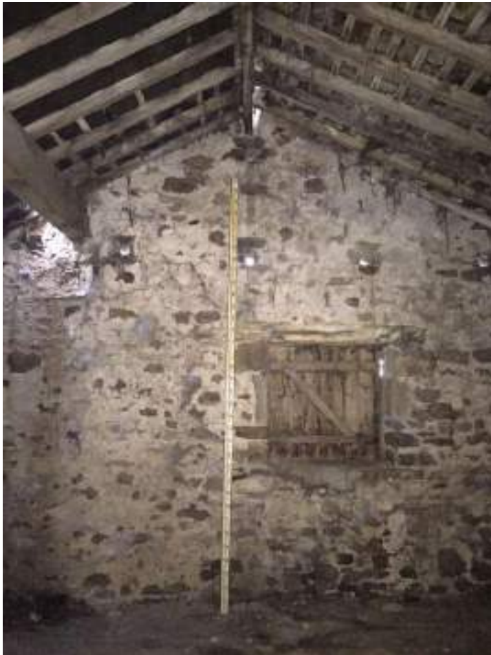
52 Access door to side elevation and detail of roof construction.
