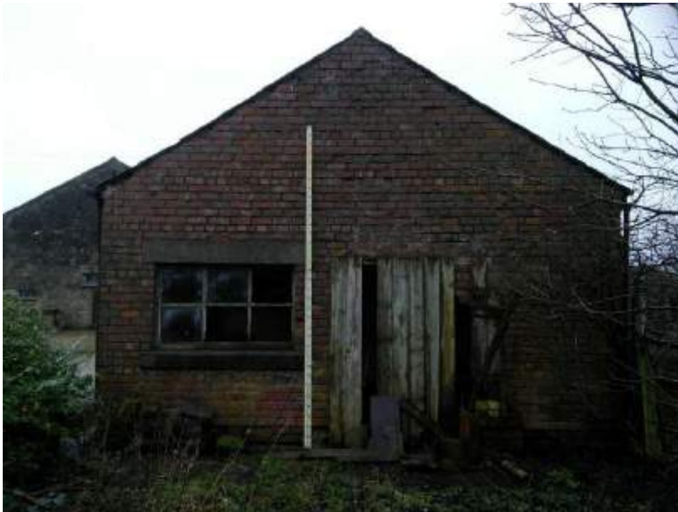
Figure 13 The south west elevation of Barn One showing end gable of the brick dairy.
