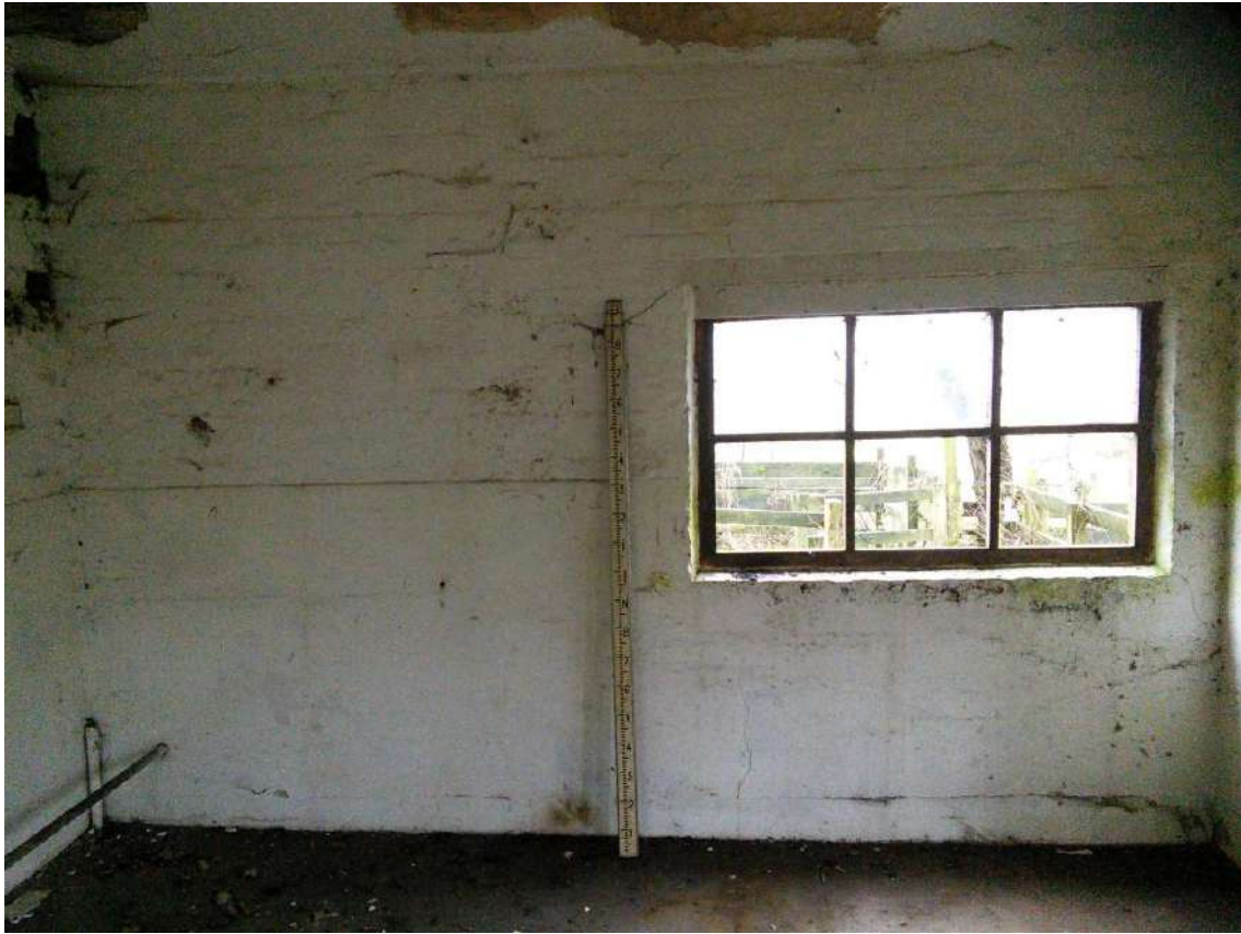
33 Rear wall and window to dairy
