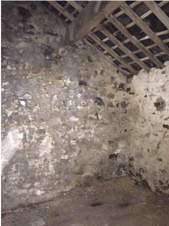
54 North west corner showing wall and roof construction.
