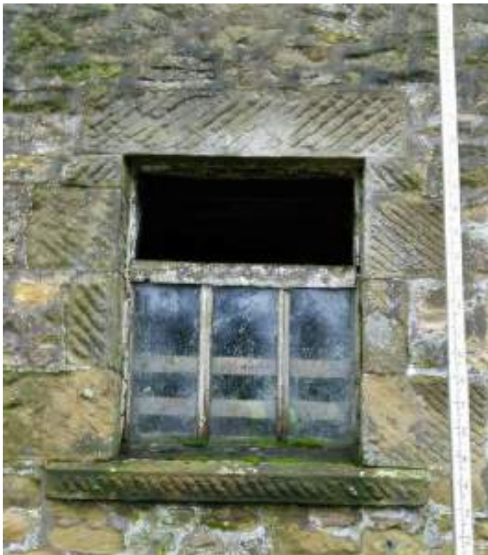
8 Window detail showing stone detailing and timber window frame
