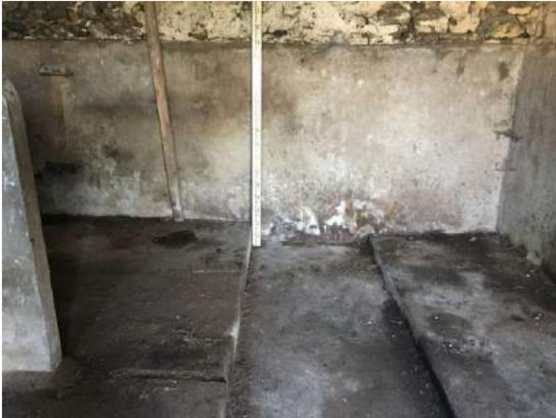
41 View of part rendered wall and concrete floor with channels, note metal rings to stall for tethering.
