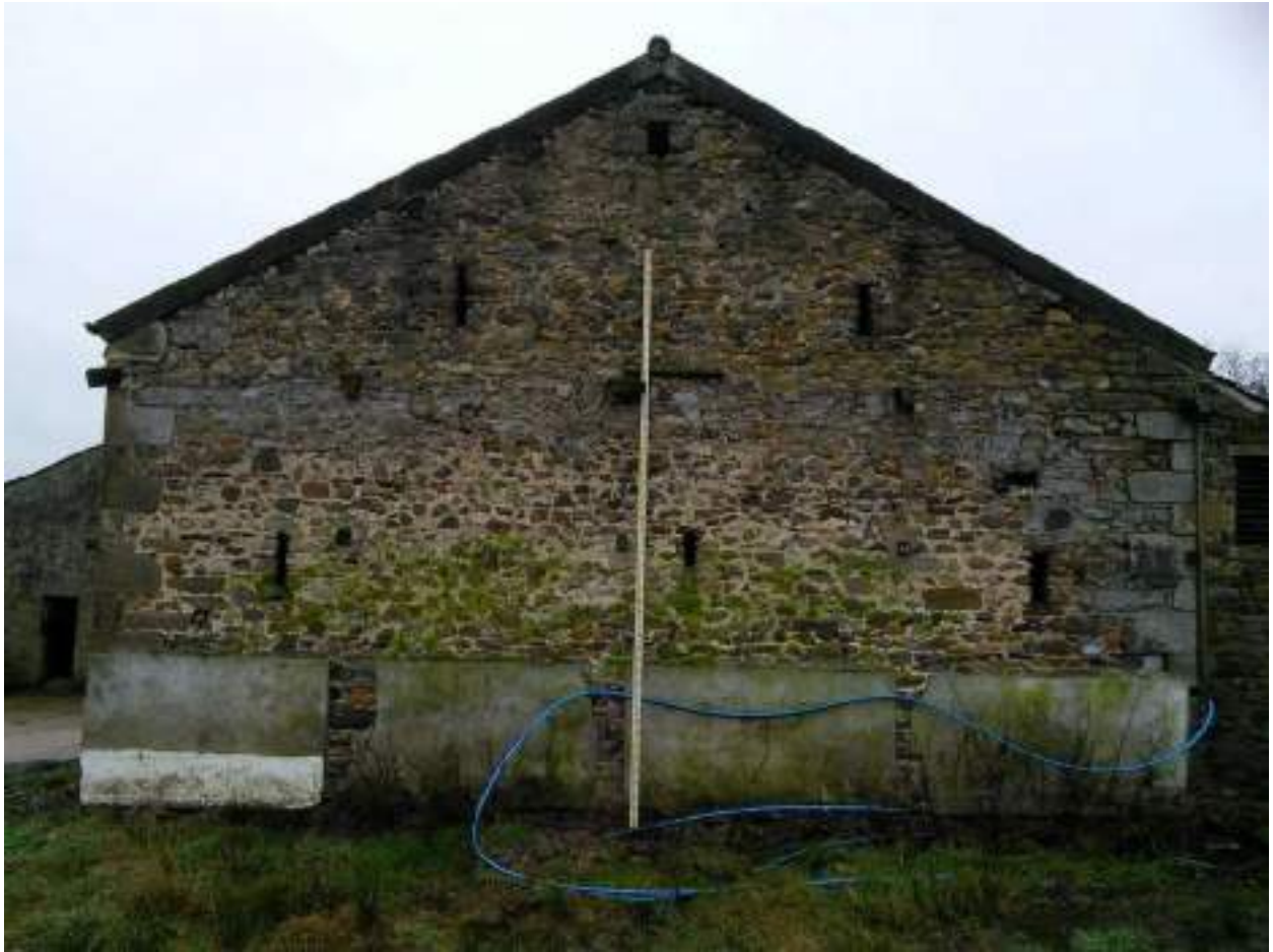
27 Northeast elevation showing gable openings and render panels at ground floor level.
