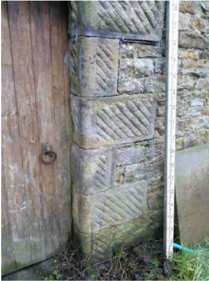
17 Curved corners to door quoins. Note boasted finish to quoins.
