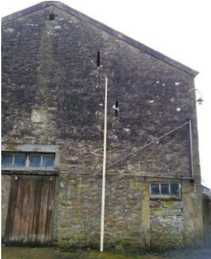
11 Owl hole and ventilation slits to gable.
