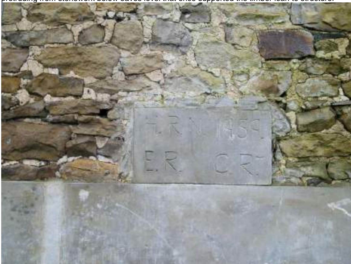
8 Initials etched into render denoting date when lean to was constructed.
