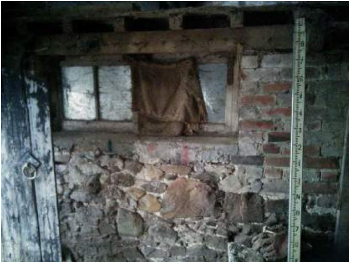
38 View of left hand side internal window to shippon partition.
