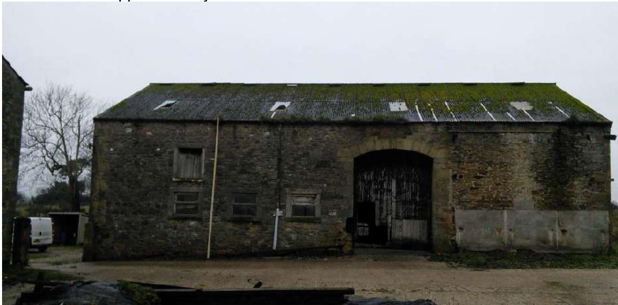
Figure 8 The south-east elevation of Barn Two showing the corrugated roof and cart entrance.
