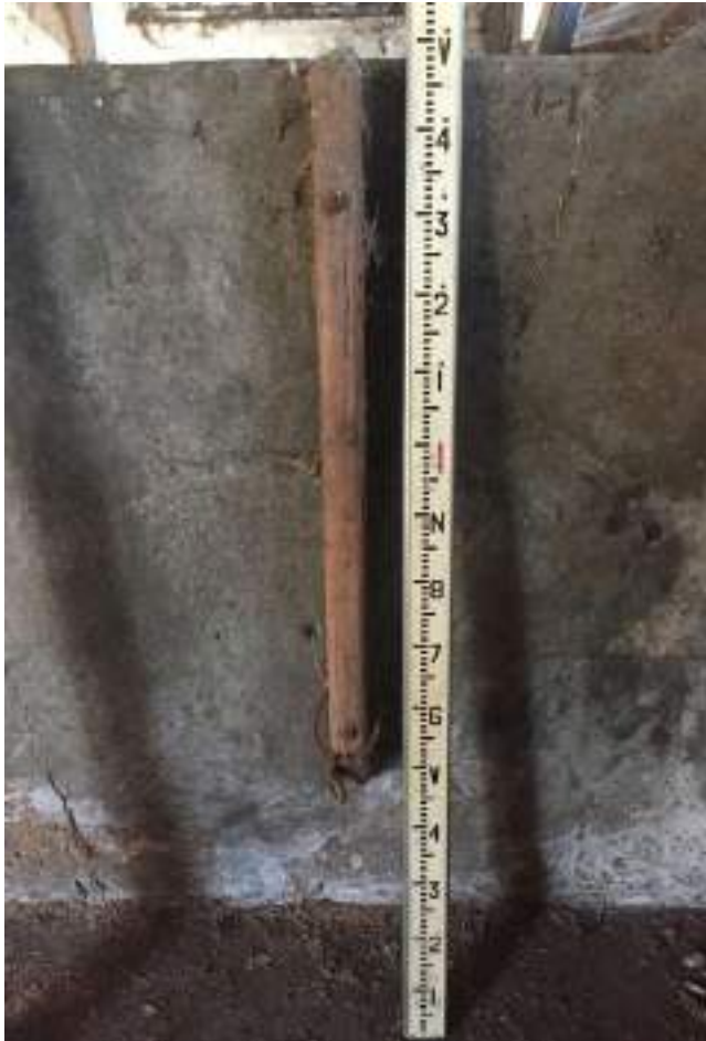
51 Detail of timber tethering post to cattle stall.
