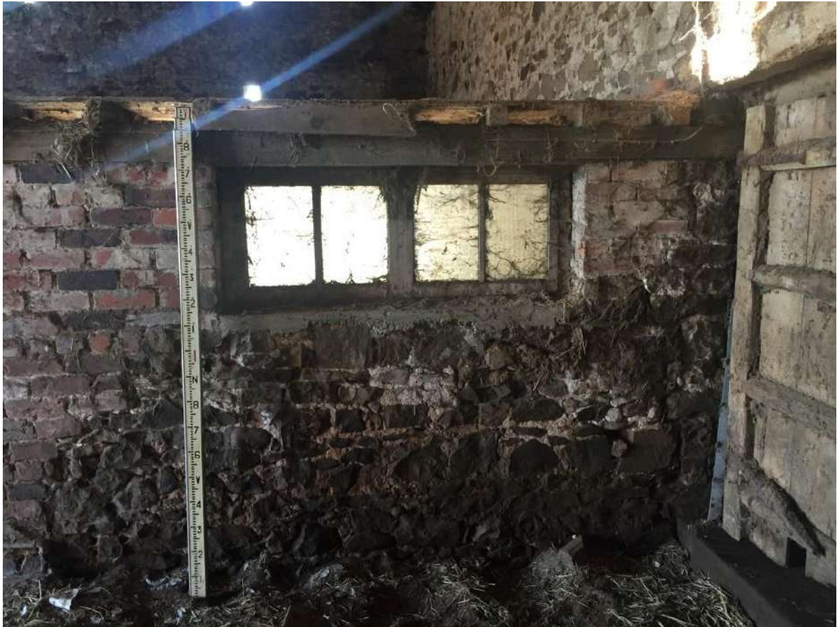
39 View of right hand side internal window to shippon partition.
