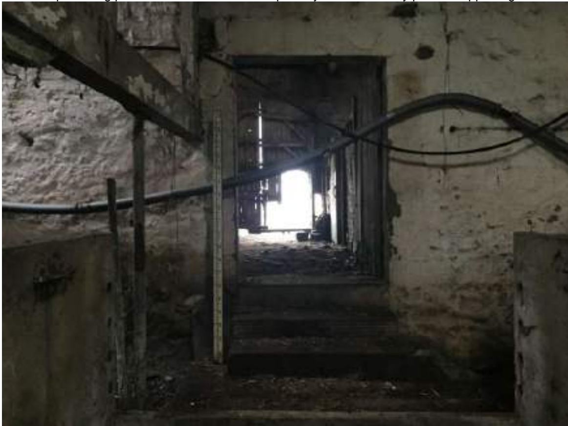
56 Door opening between outshut / shippon and main barn.
