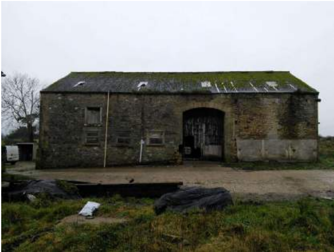
1 Front (southeast) elevation showing cart entrance.
