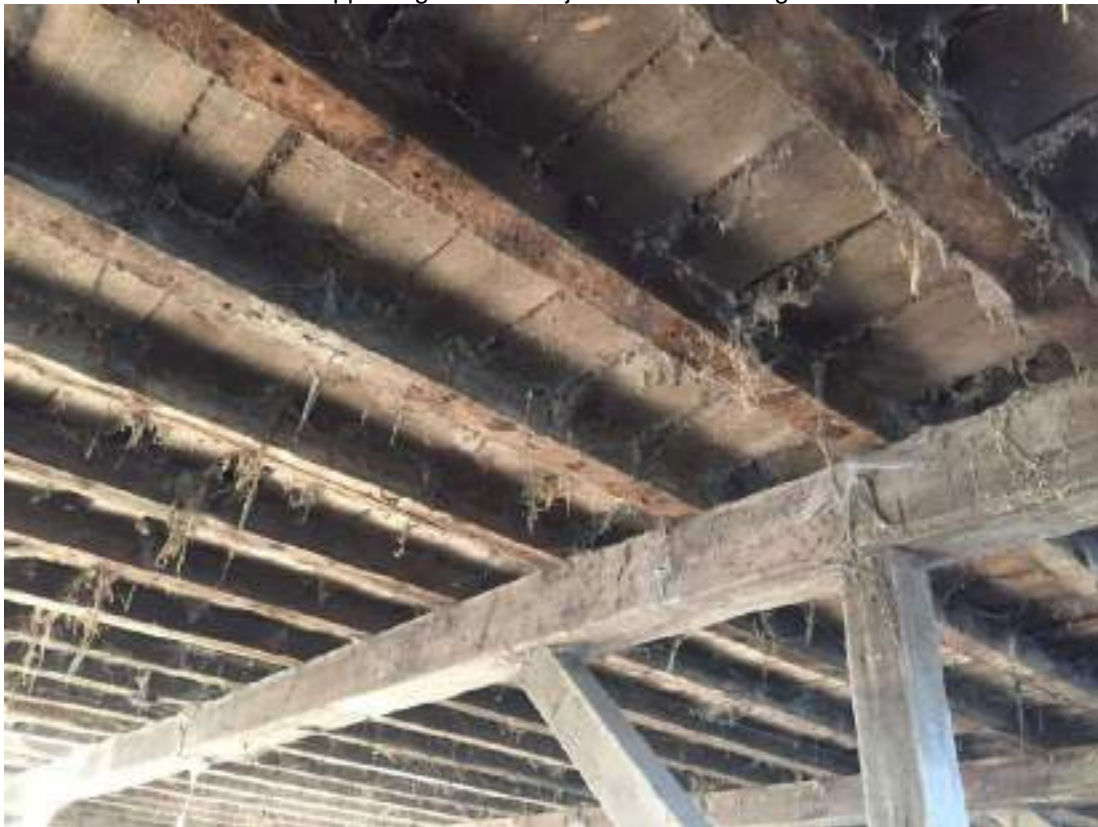
50 View of timber deck ceiling showing floor joists and supports.
