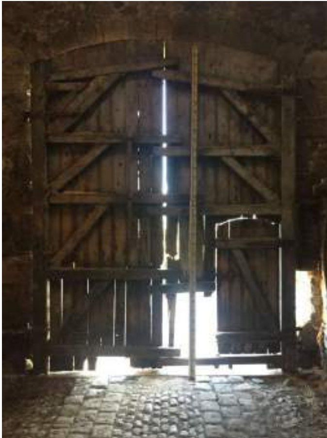
33 Cart entrance door
