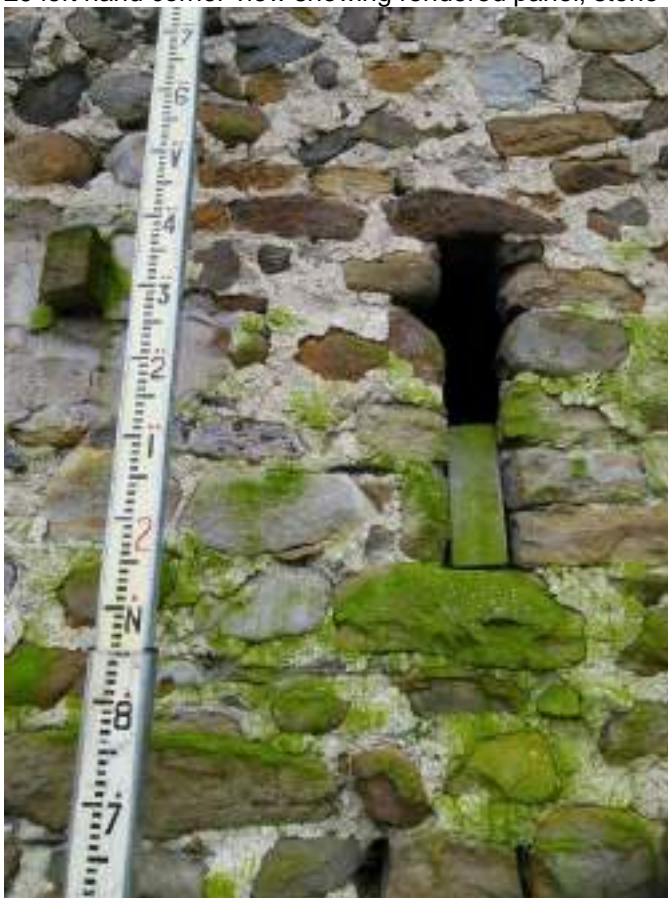
30 Detail of ventilation slit to gable wall.
