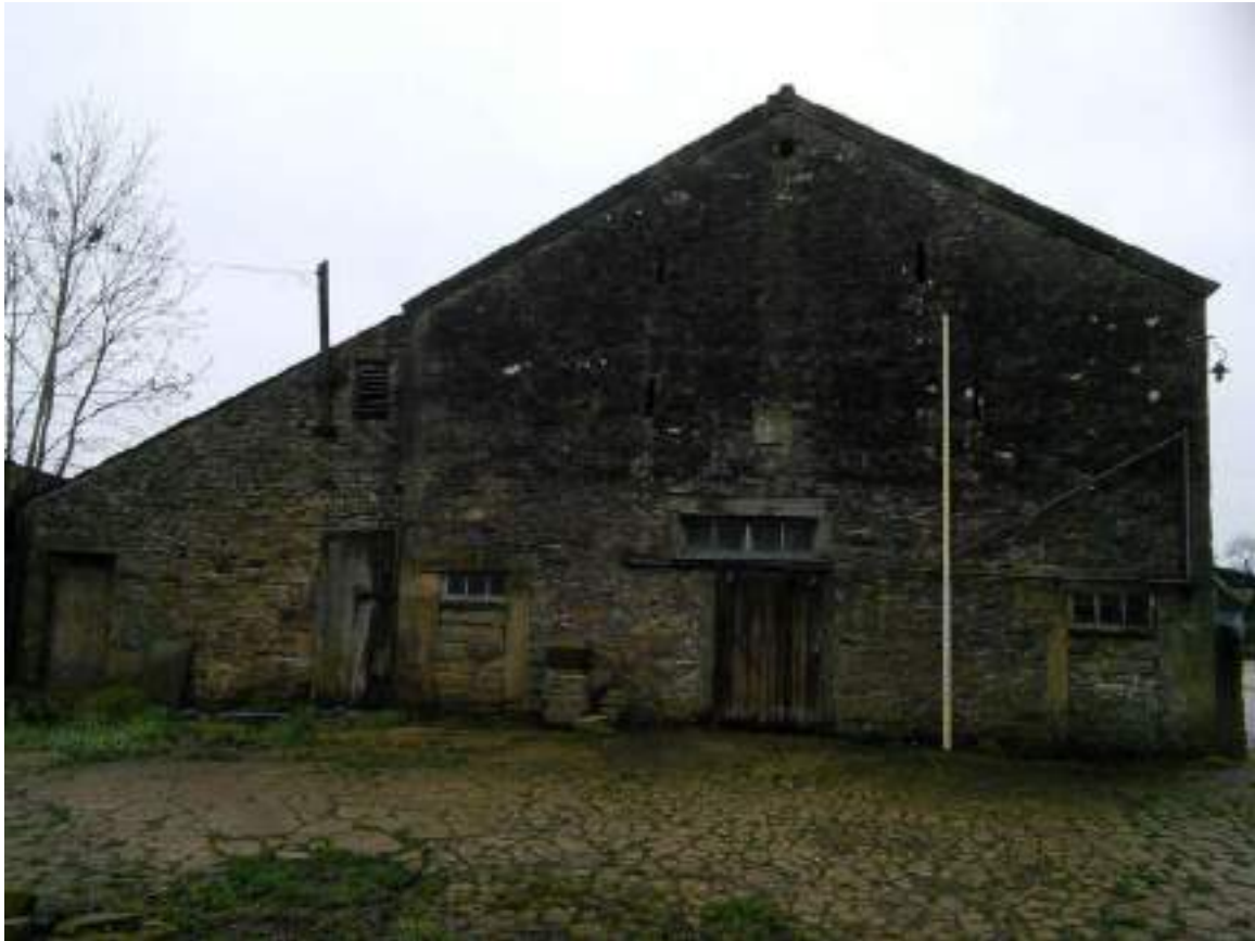
9 View of side (southwest) elevation
