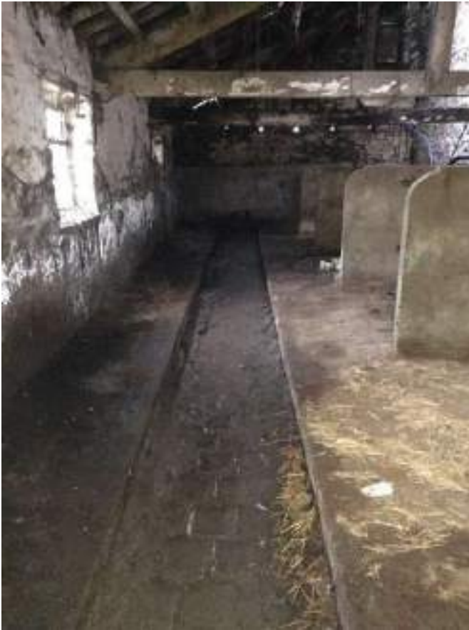
57 View of manure channel to stalls. Note manure channel is comprised of stone setts
