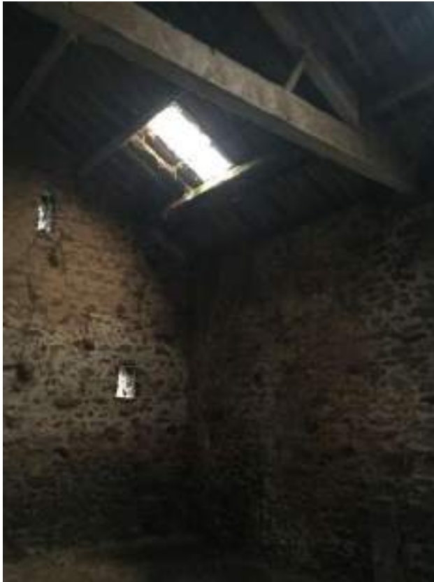
Figure 20 Internal view of the southeast corner showing rooflight and ventilation slits.
