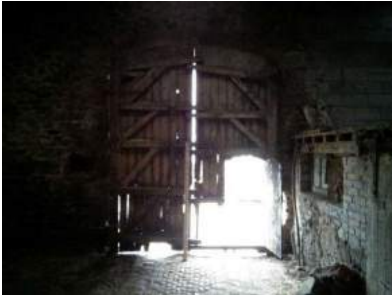
Figure 18 Internal view of the cart entrance doors
