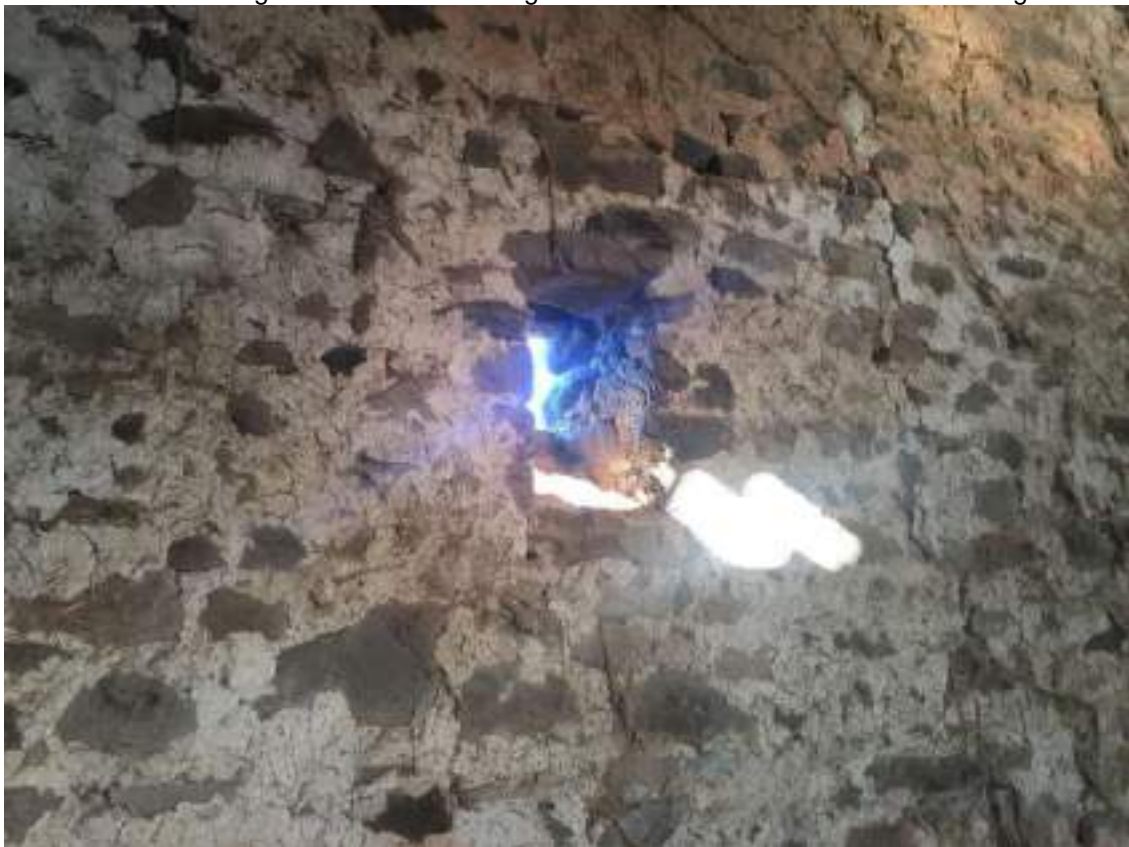
44 typical view of ventilation slit within stone gable, note splayed reveals.
