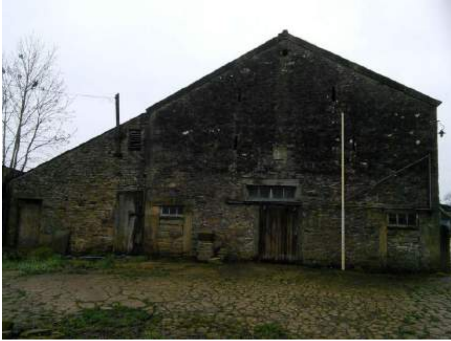
Figure 12 The south west elevation of Barn Two showing the access doors to the shippon and outshut. Note the fanlight over the central doorway and the blocked up former doorways.
