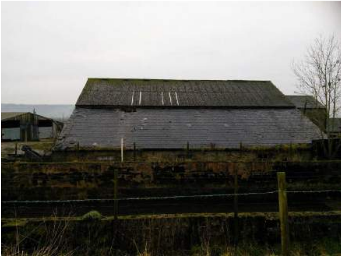
19 Rear (northwest) elevation showing slurry tank in foreground and roof of barn.
