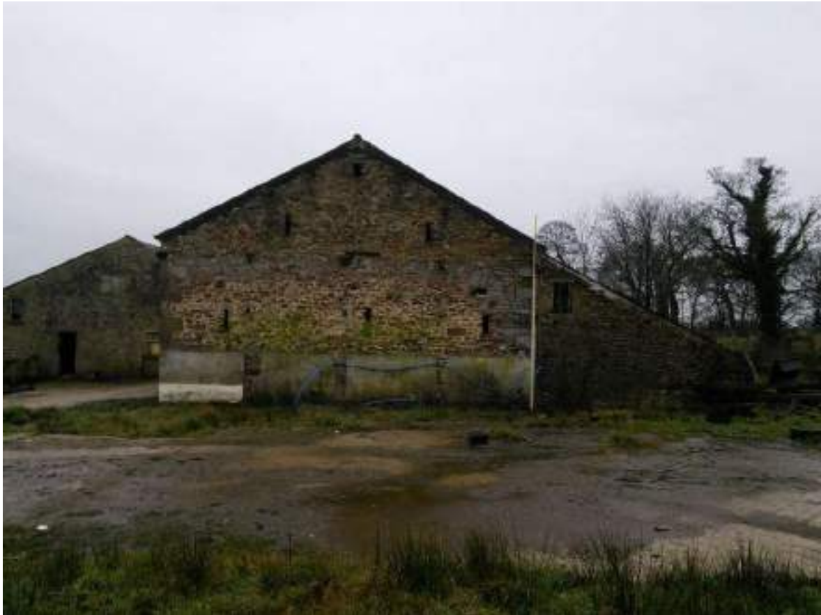
25 Side (northeast) elevation showing single storey outshut in context with main barn structure.
