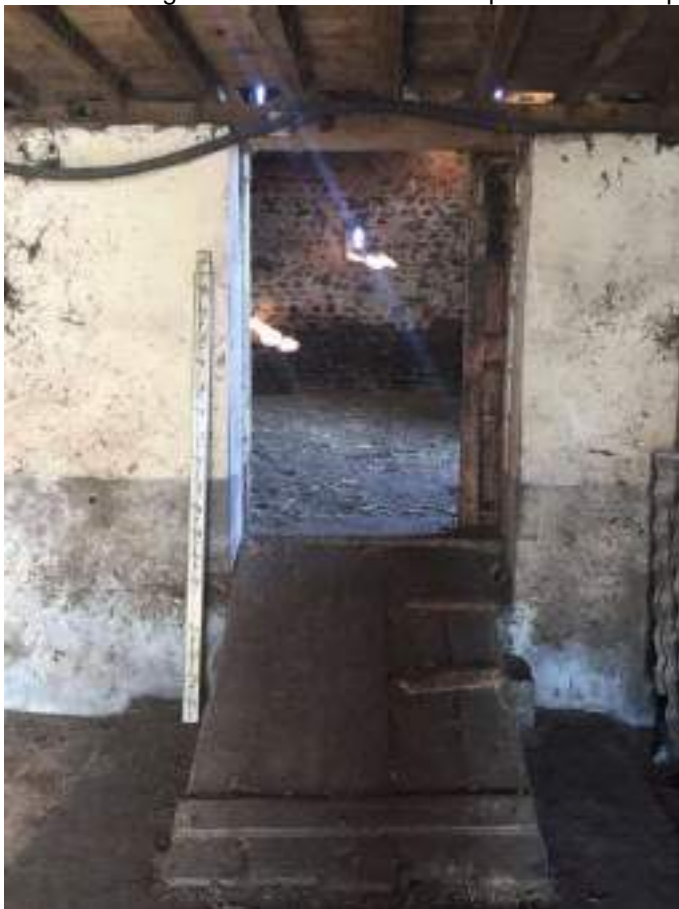
48 View showing timber ramped access and doorway.
