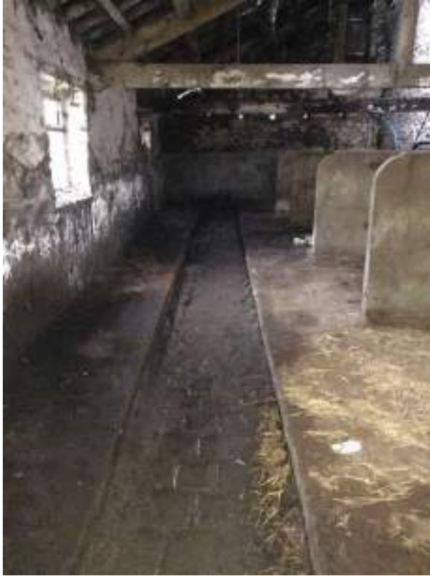
Figure 27 View along rear shippon passageway showing manure channel and concrete cattle stalls.
