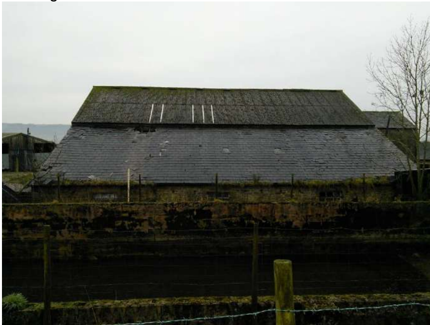
Figure 14 The north-west elevation of Barn Two showing the rear outshut structure and disused slurry tank directly to the rear of the barn.
