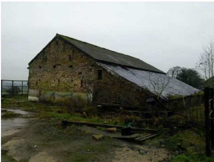
Figure 16 The north-east elevation of Barn Two showing the rear outshut.
