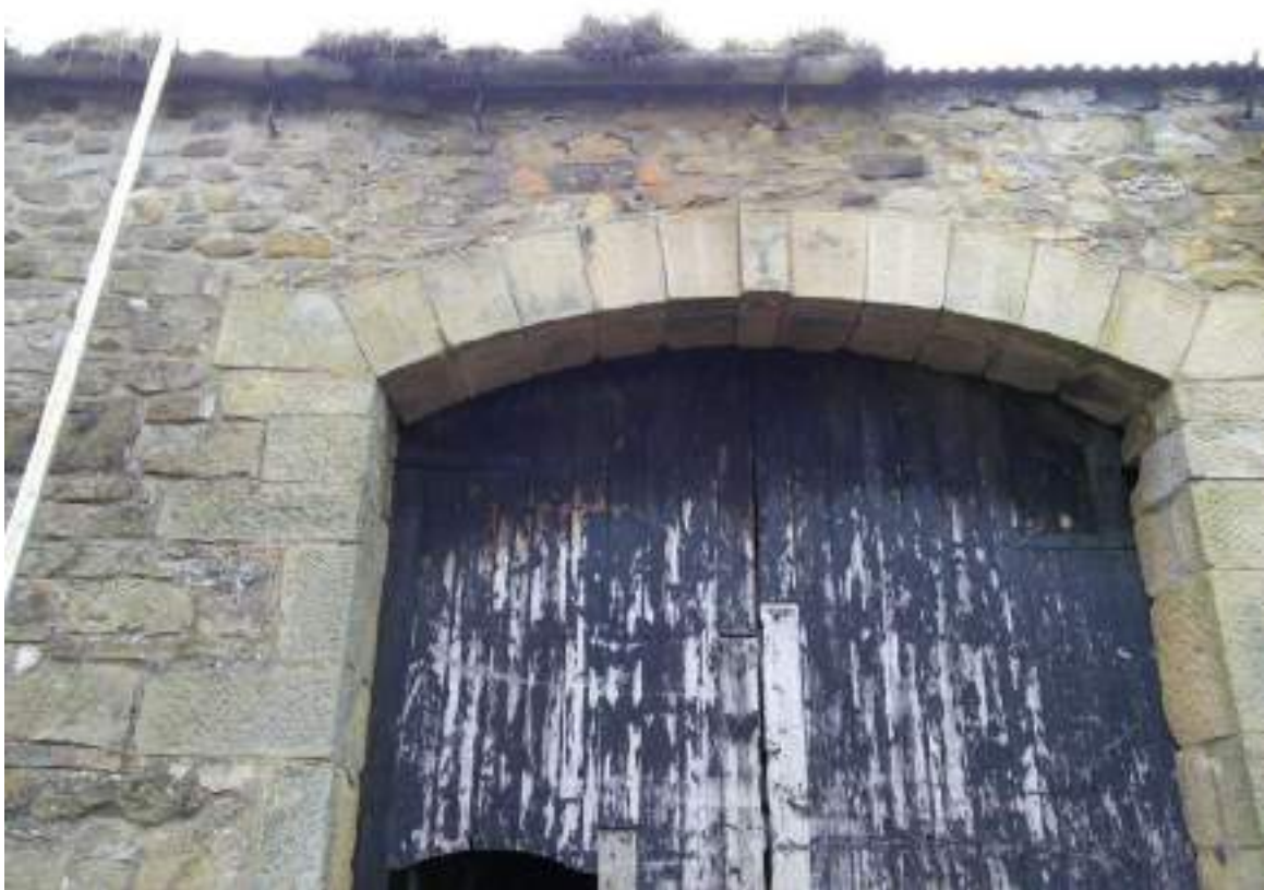
6 Detail of stone archway and timber cart door.
