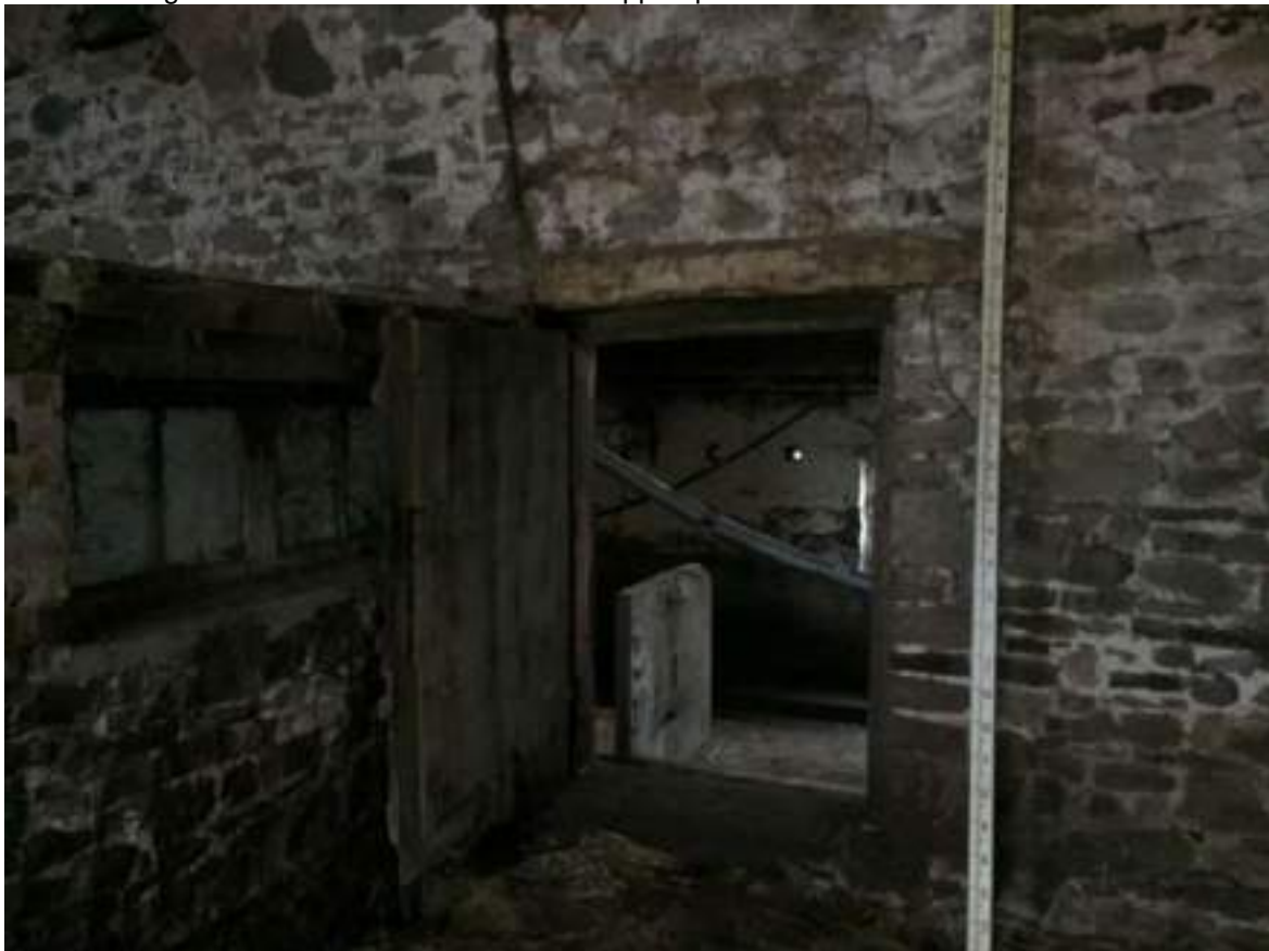
40 view of timber door and opening into rear shutout / shippon
