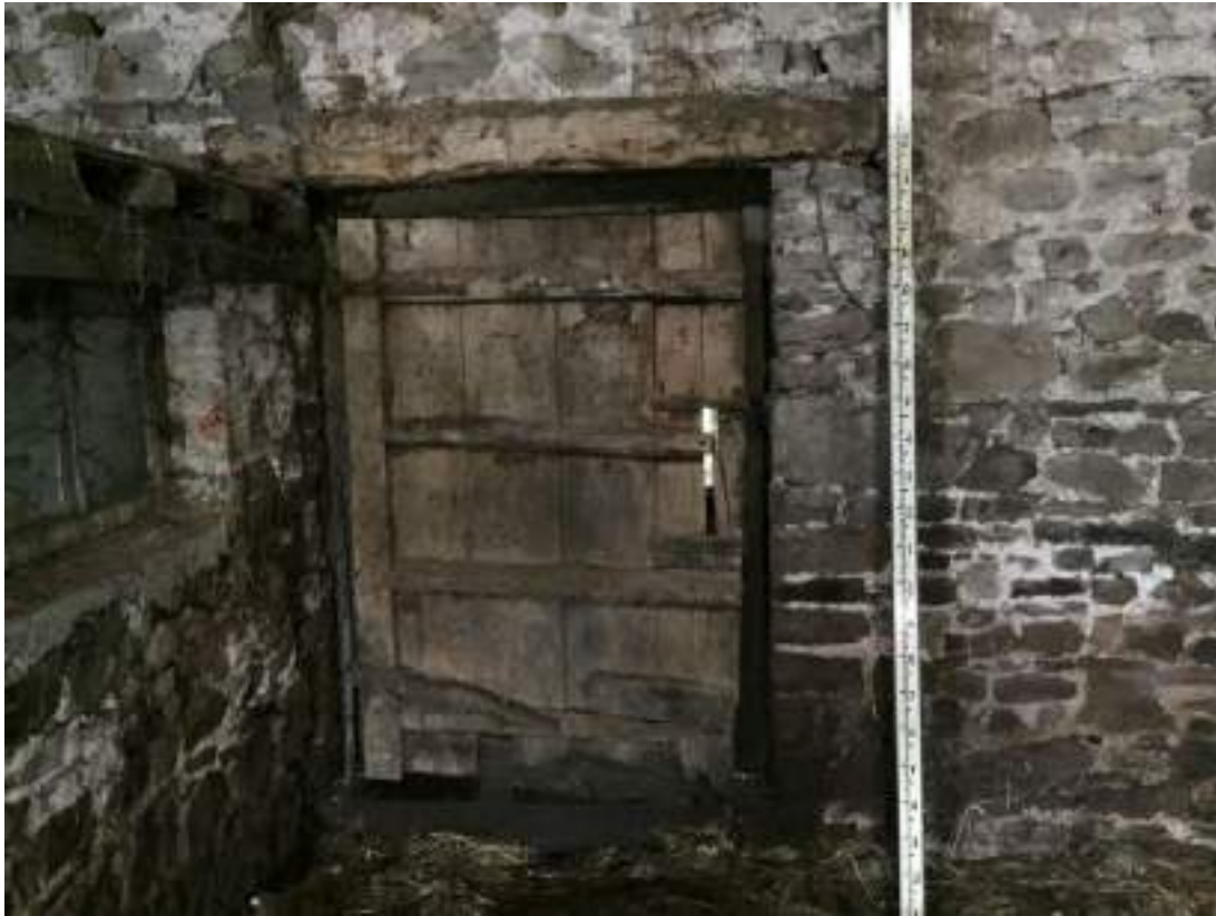
41 View of door closed showing construction and timber lintel above.
