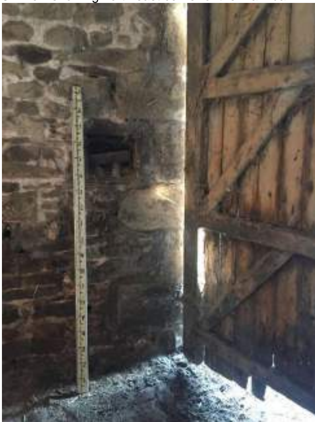
32 View showing internal quoins to cart entrance doorway, note alcove within wall, an adjacent alcove is present on the opposite wall.
