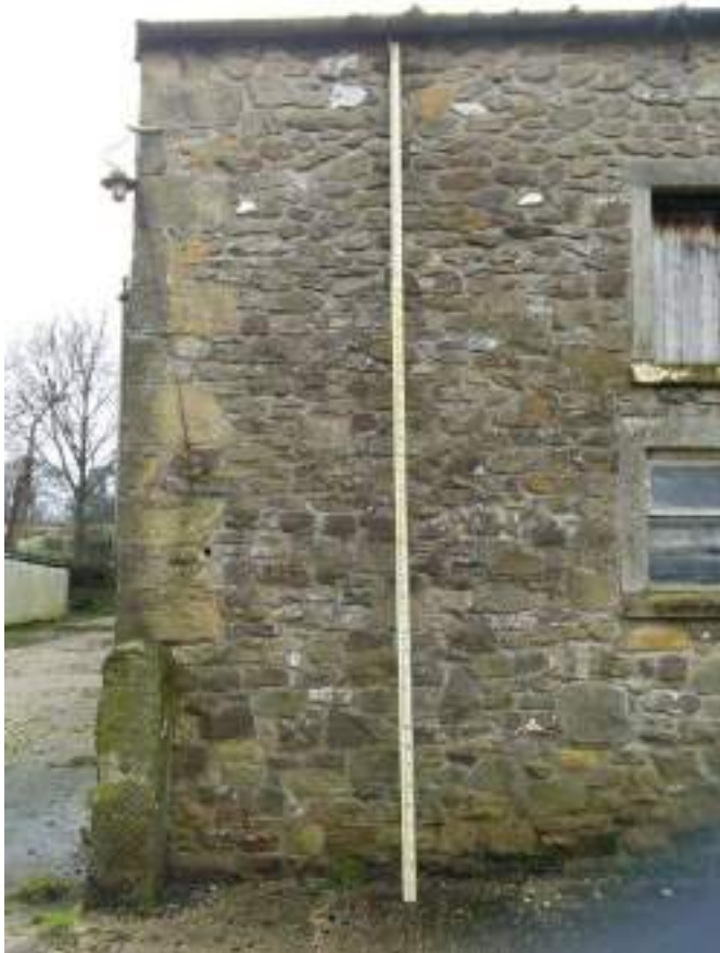
2 Corner quoins and gatepost to southern corner.
