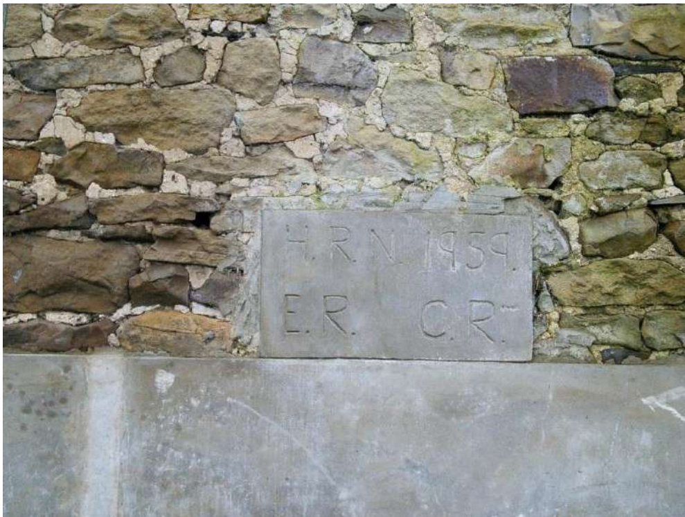
Figure 11 Inscription set into render where the timber structure was removed.
