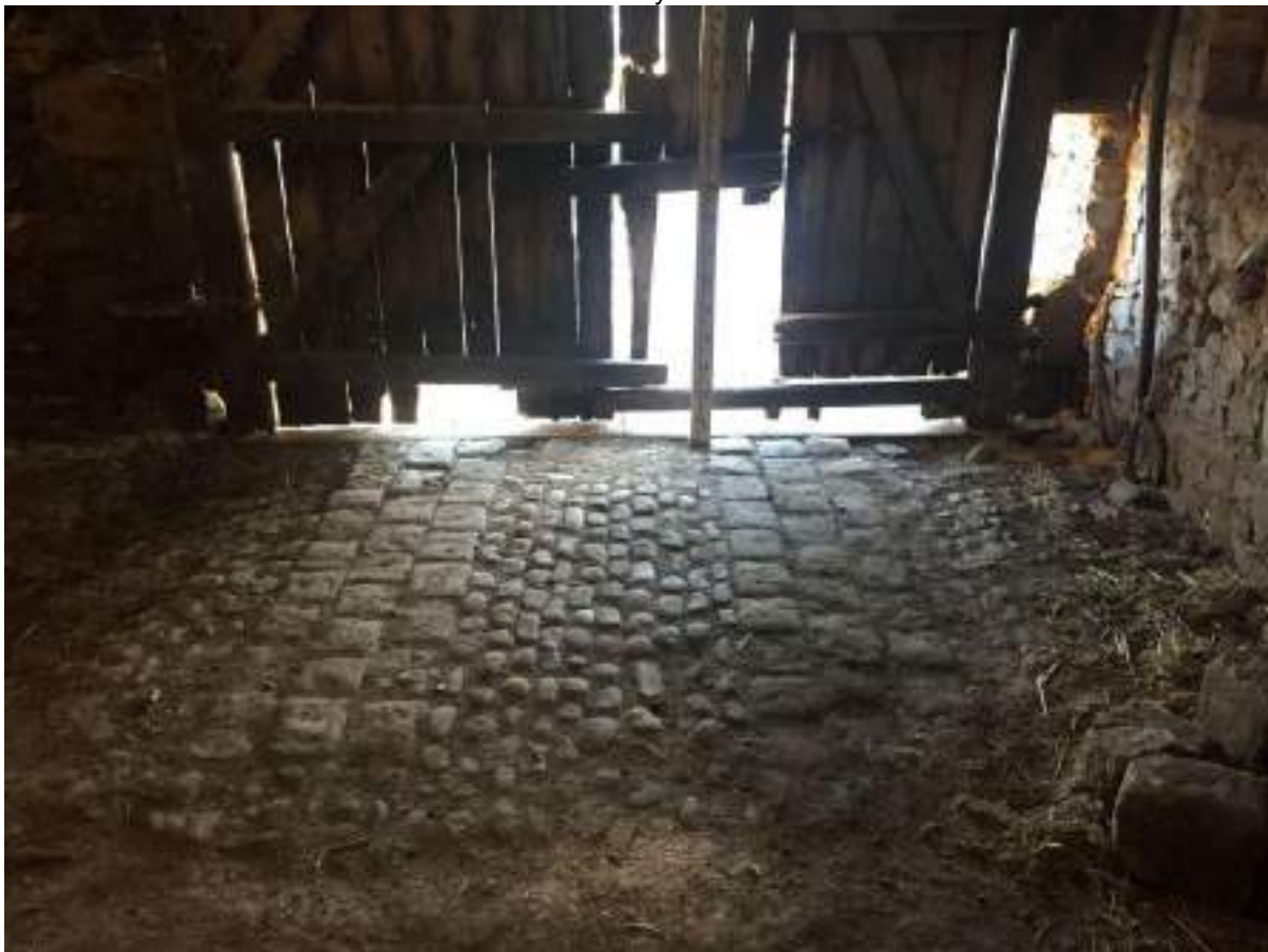
46 Further detail of stone setts
