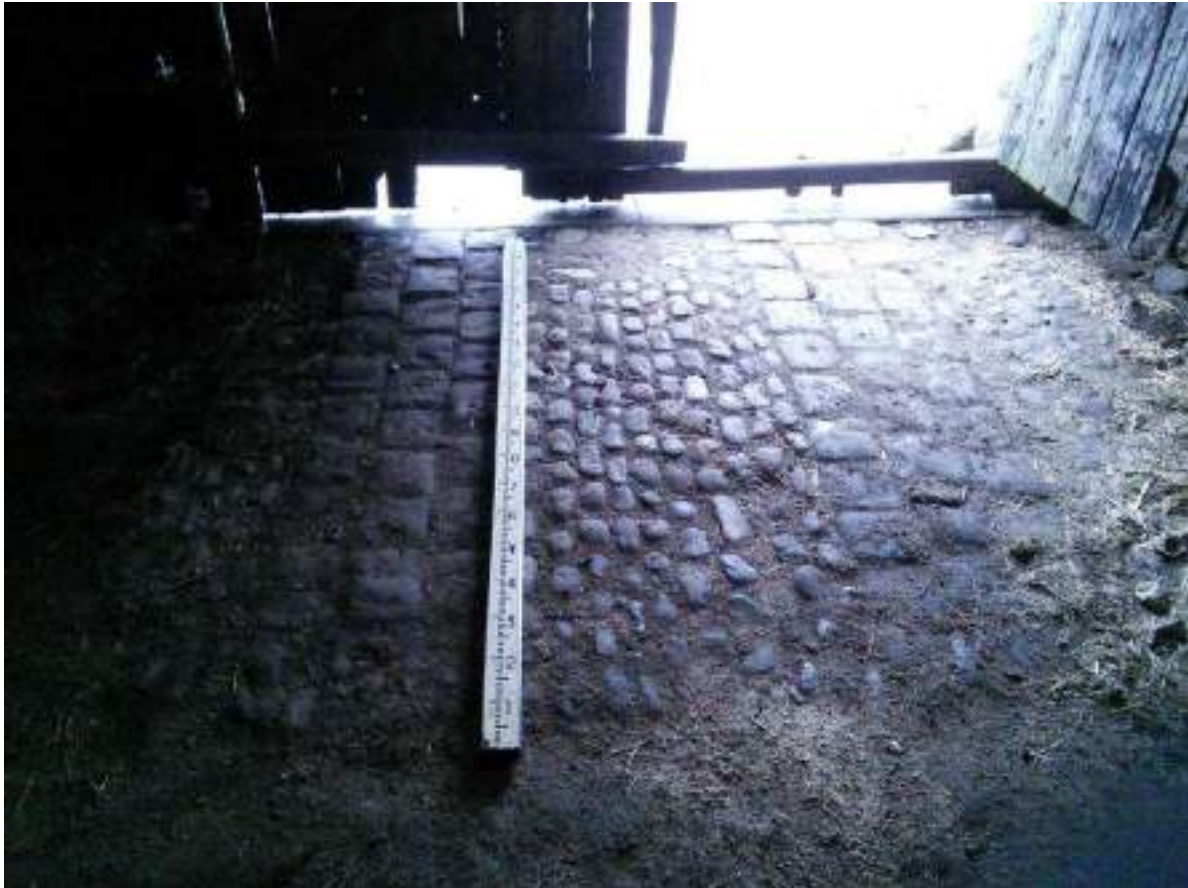
45 Stone setts and cobbles to cart entrance doorway.
