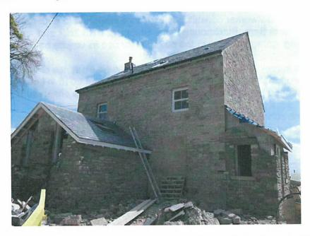
The property is a traditional stone built two storey farmhouse with a double pitched tiled roof. Pointing is in good condition with no cracks or crevices present. Two single storey extensions are present. The property is undergoing renovation and re-roofing has been carried out over the winter of 2016 in keeping with good practice re: timing of works. A separate outbuilding is similarly undergoing repair and renovation.
