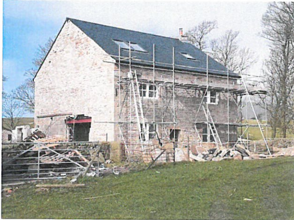
Abbot Barn Farm – view looking north-west.
