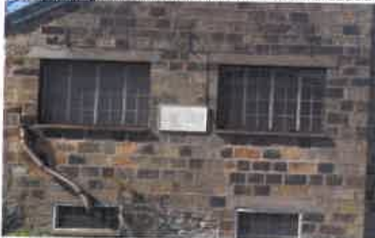
Coursed sawn stone N.E elevation
