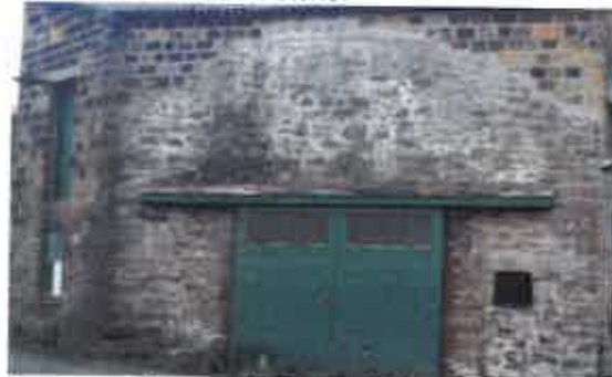
Random and coursed stone on N.W elevation
