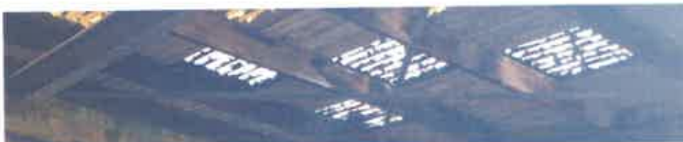
Underside of canopy roof
