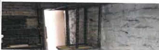
Garage interior walls
