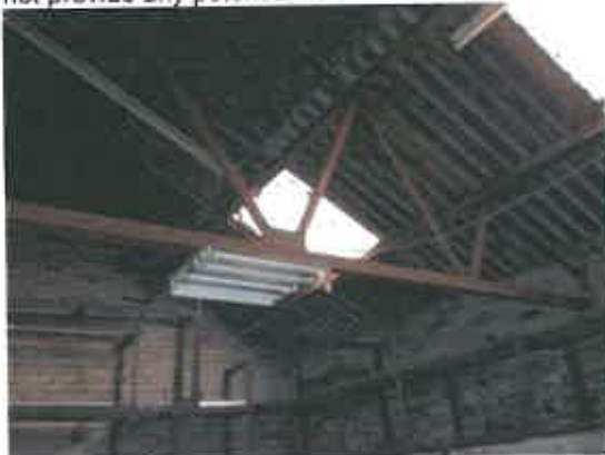
Internal roof space
