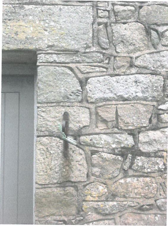
PLATE 1 SUN LOUNGE/NEW OPENING STONE DETAIL TO BE USED AROUND WINDOW REVEALS WITH NATURAL STONE LINTEL VARIOUS SIZES IN HEIGHT ON FACE 150 MM, 200 MM 300 MM .APPROX 150MM DEPTH.RANDOM STONE WALLING VARIOUS SIZES TO BE BUILT UP TO MATCH APPEARANCE.
