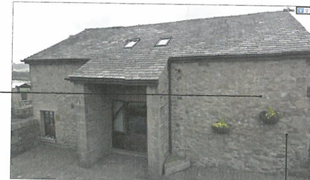
PLATE 7 WEST ELEVATION Proposed sun lounge extension to match random stone walling with dressed stone quoins
