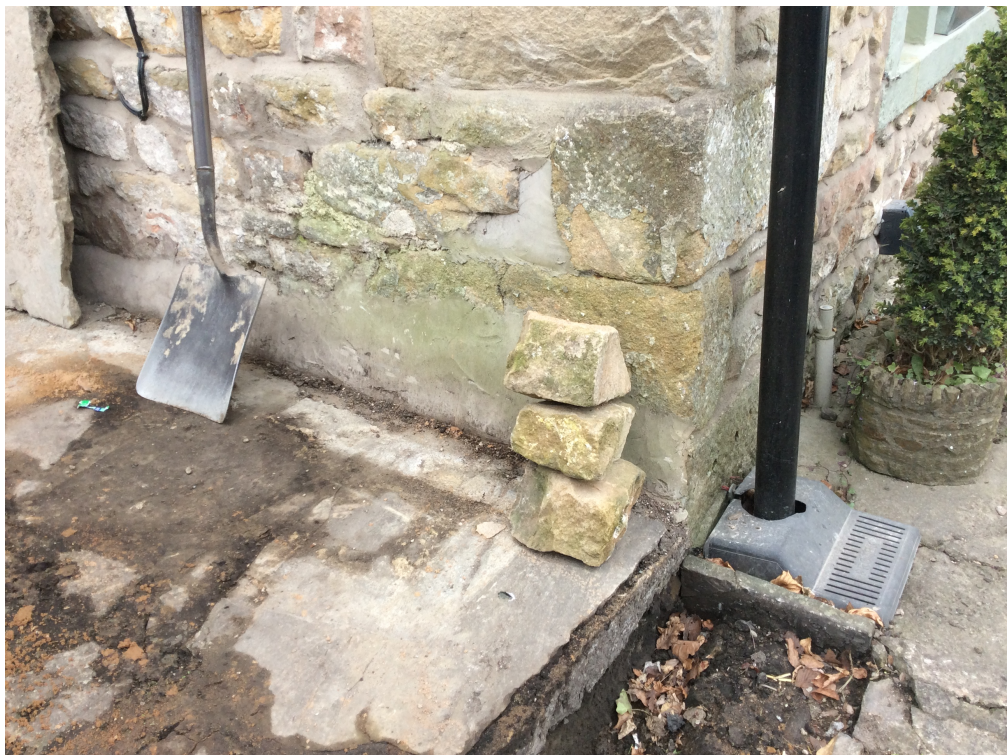
Photograph showing the proposed reclaimed stone for the garden wall and wall under the new bay window
