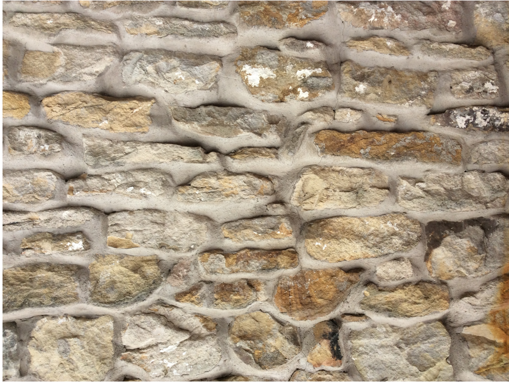
Photograph showing the existing stone
