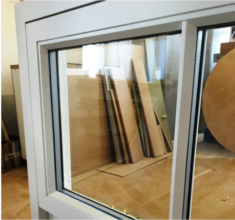
Photograph showing the beads of the top hung casement window
