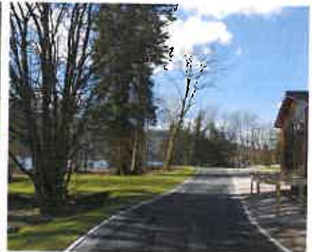
Falbarrow Park, Windermere: Completed CellWeb TRP® Installation
