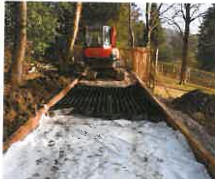
Falbarrow Park, Windermere: CellWeb TRP® Installation
