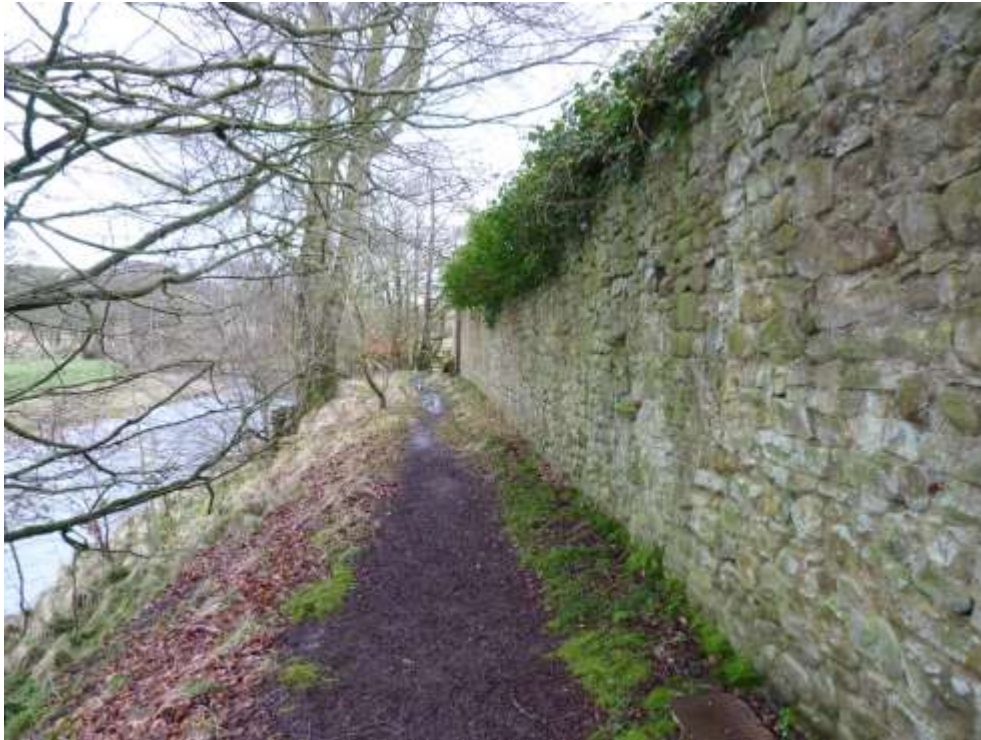
Photograph 3 – Outside northeast boundary of the site looking east along wall on northern boundary
